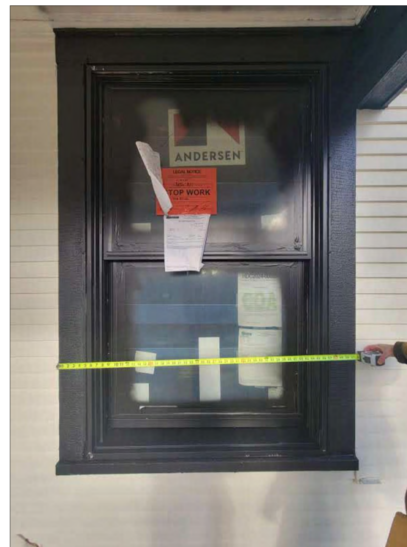
5 FRONT ELEVATION EXISTING WINDOW PHOTO TAKEN NOVEMBER 26, 2024
