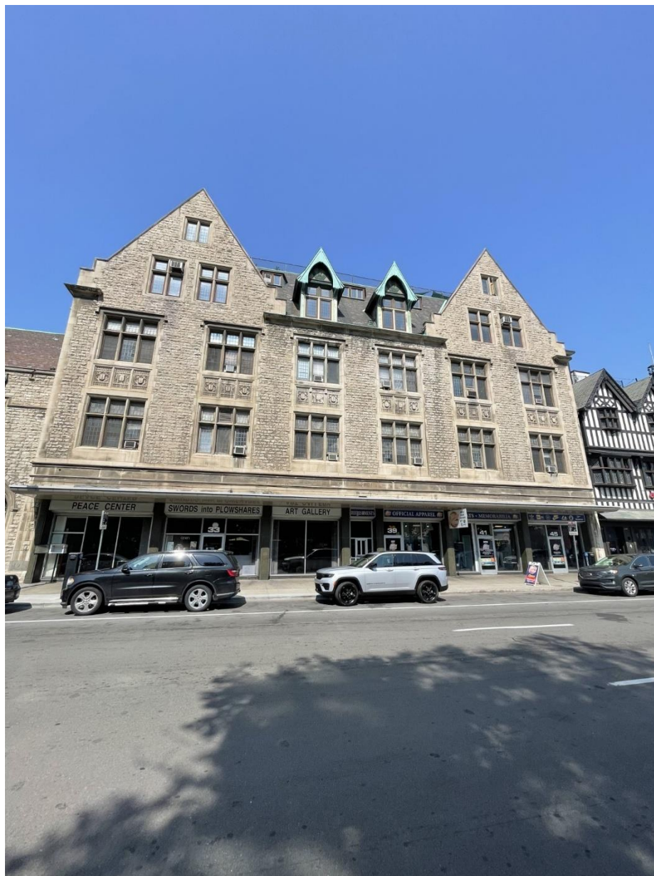
Side View (South East Face of Building)
