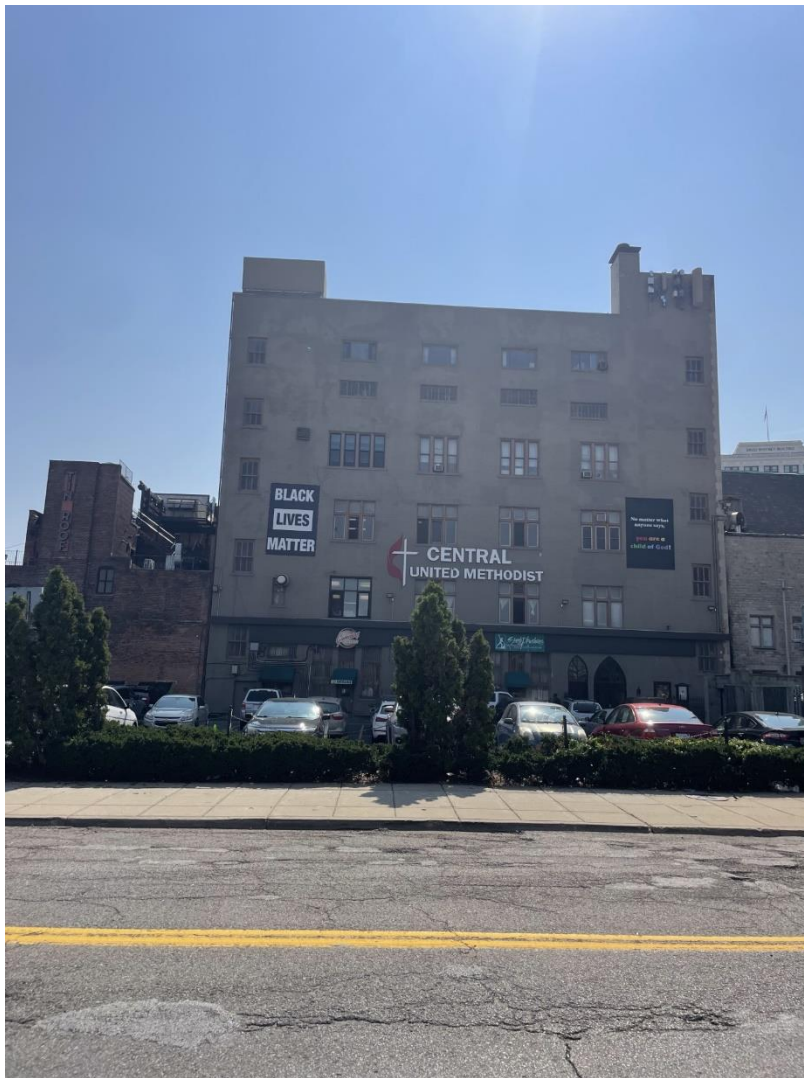
Side View (North West Face of Building)
