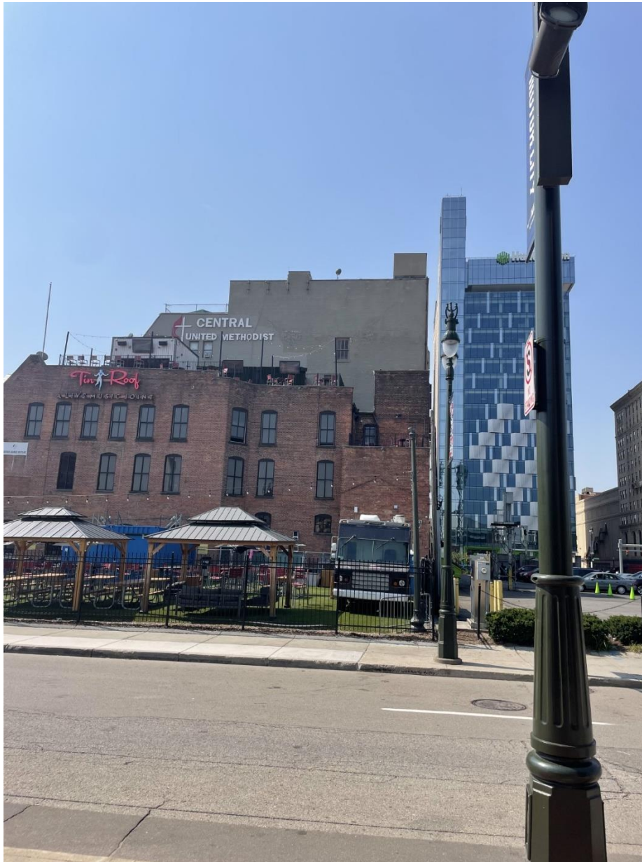
Front View (North East Face of Building)
