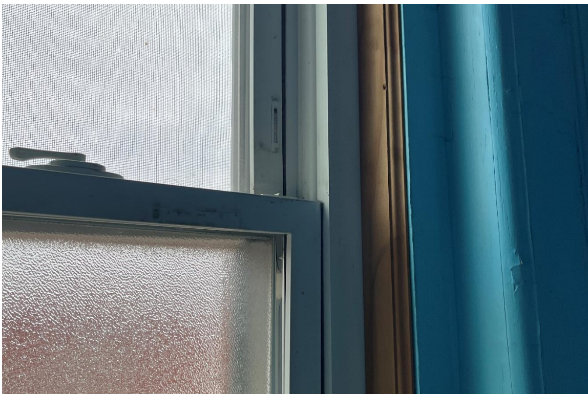
Window 1. 3 rd Floor, east elevation. Vinyl replacement unit. 12/11/2024.
