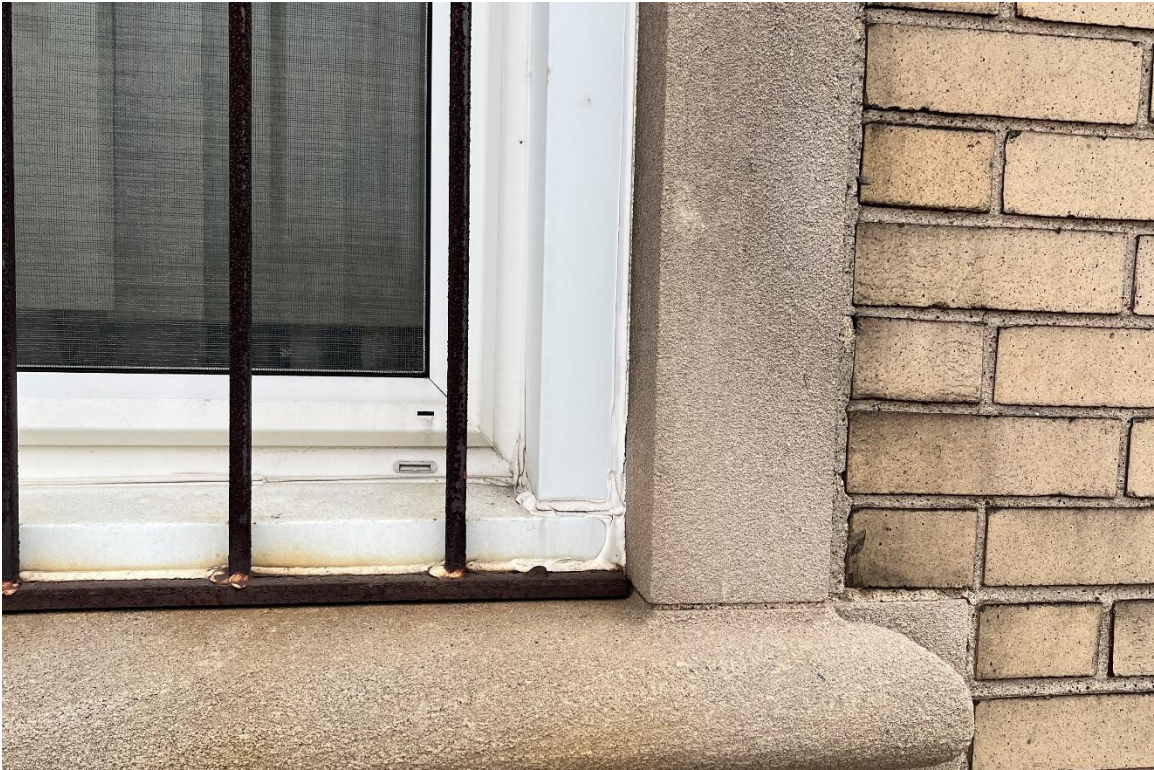
Window 6. 1 st Floor, south elevation. Vinyl replacement unit. 12/11/2024.
