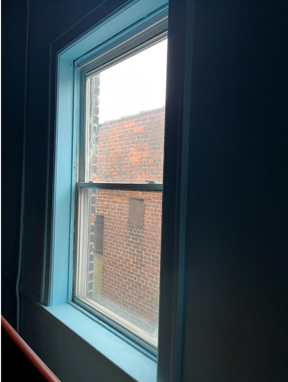
Window 14. 3 rd Floor, alcove, west elevation. Vinyl replacement unit. 12/11/2024.
