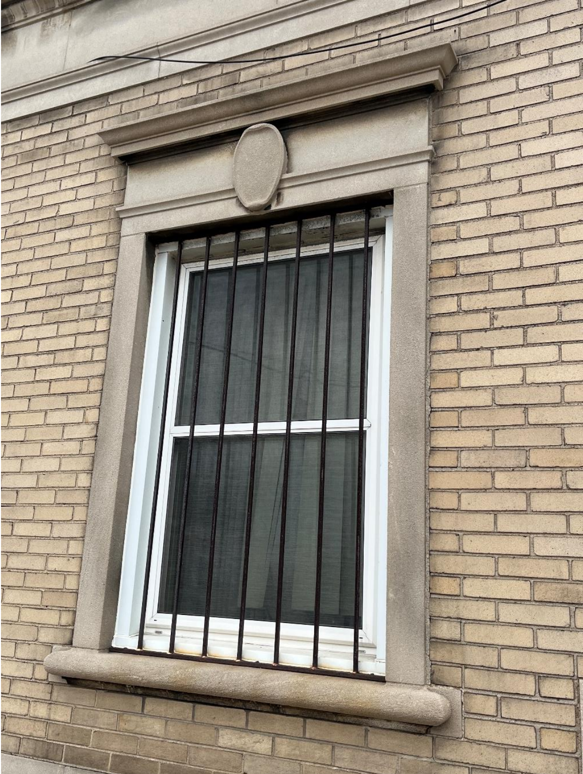
Window 6. 1 st Floor, south elevation. Vinyl replacement unit. 12/11/2024.
