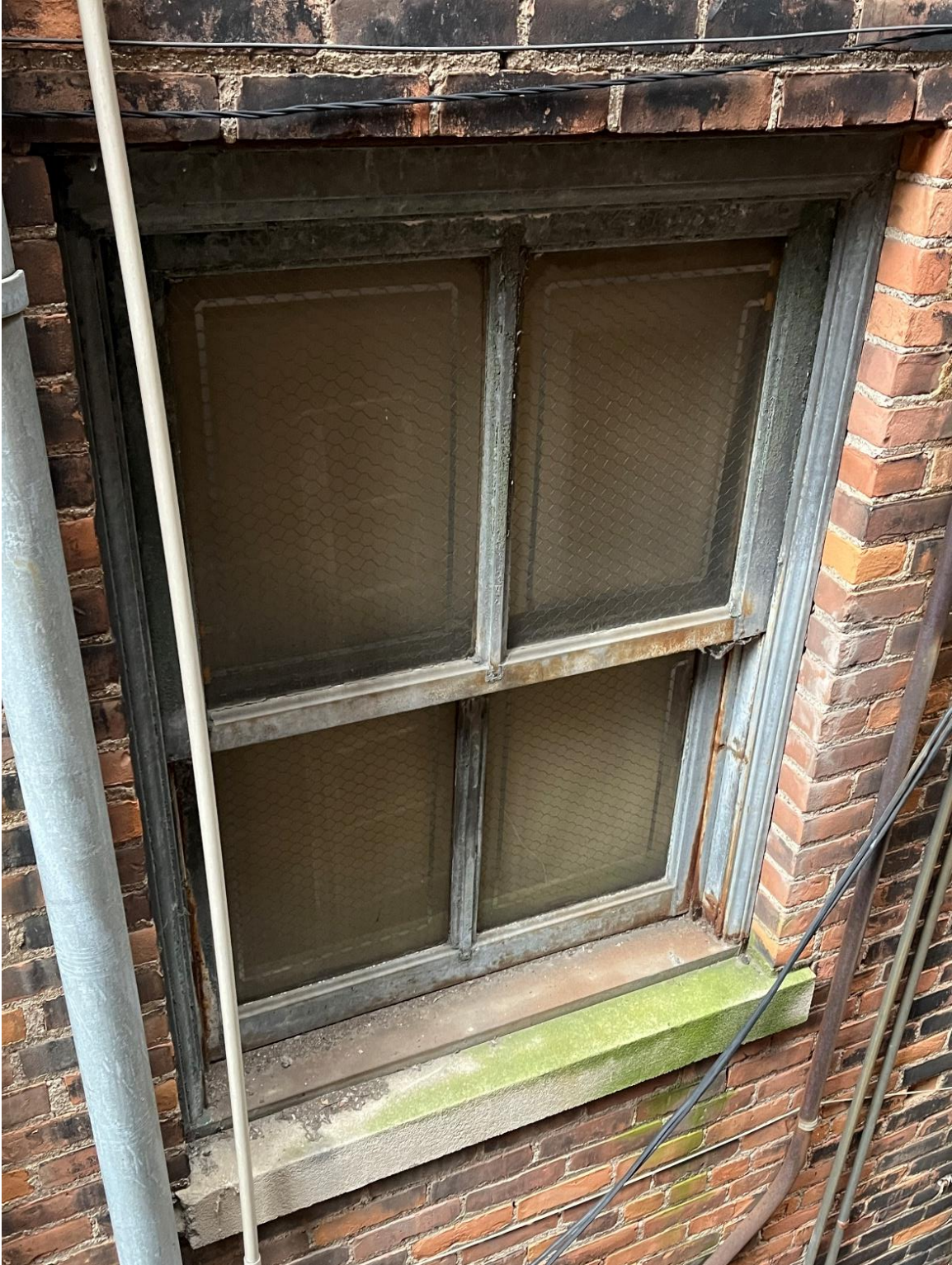
Window 15. 1 st Floor, alcove, west elevation. Cold rolled steel unit. 12/11/2024.
