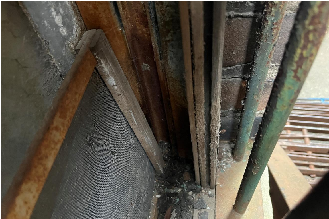
Window 10. 1 st Floor, alcove, east elevation. Cold-rolled steel unit. 12/11/2024.
