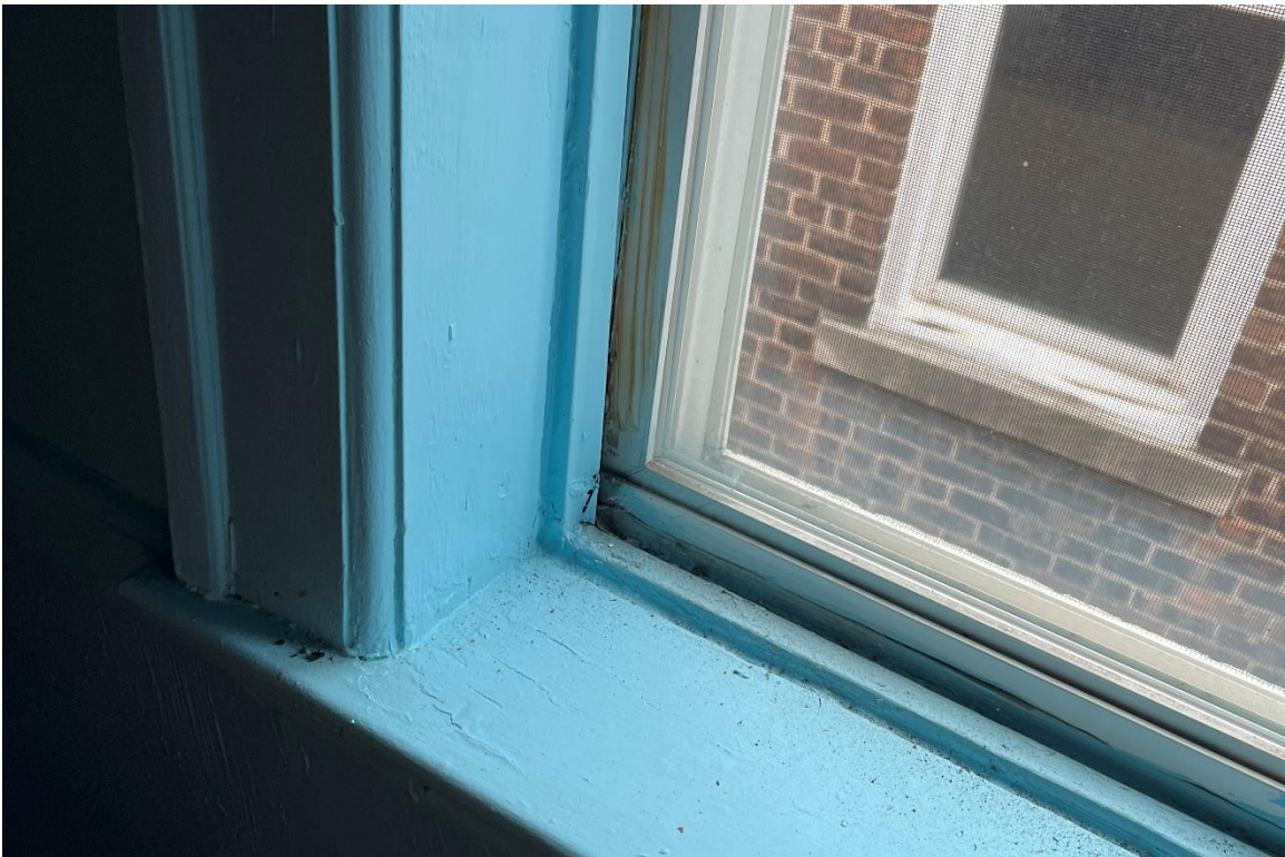
Window 14. 3 rd Floor, alcove, west elevation. Vinyl replacement unit. 12/11/2024.
