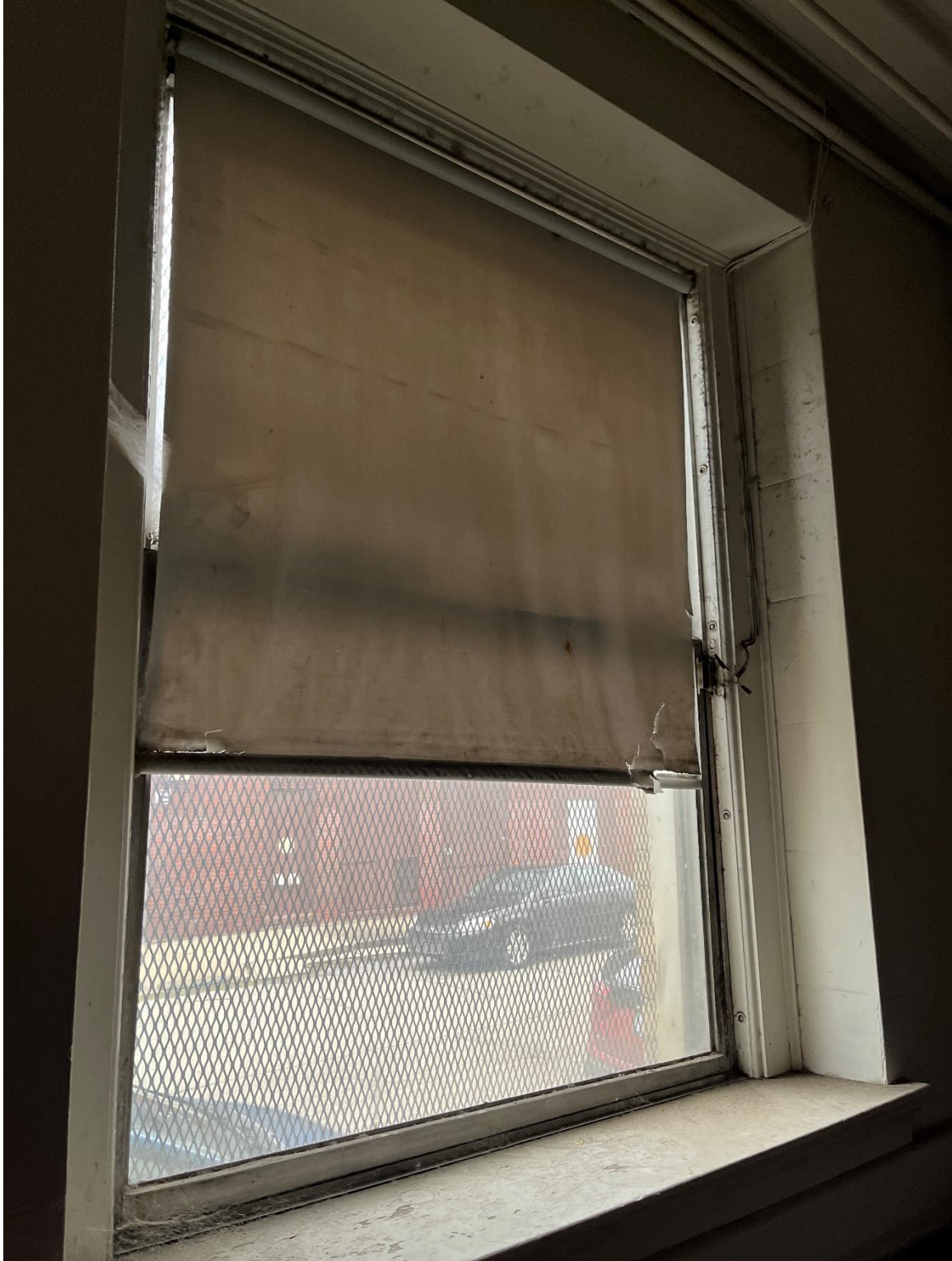
Window 3. 1 st floor, east elevation. Aluminum replacement unit. 12/11/2024.
