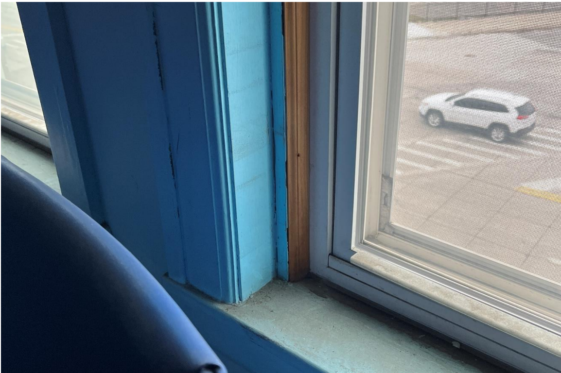
Window 7. 3 rd Floor, west elevation. Vinyl replacement unit. 12/11/2024.
