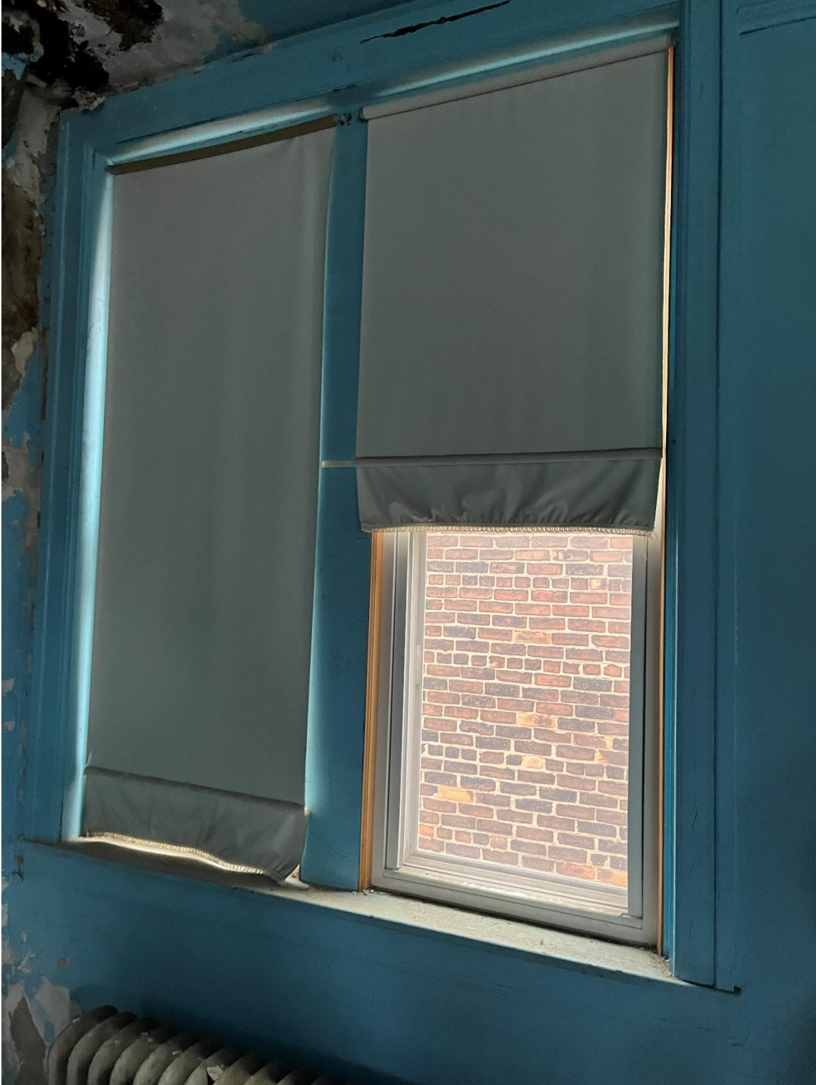
Window 8. 3 rd Floor, alcove, east elevation. Vinyl replacement units. 12/11/2024.
