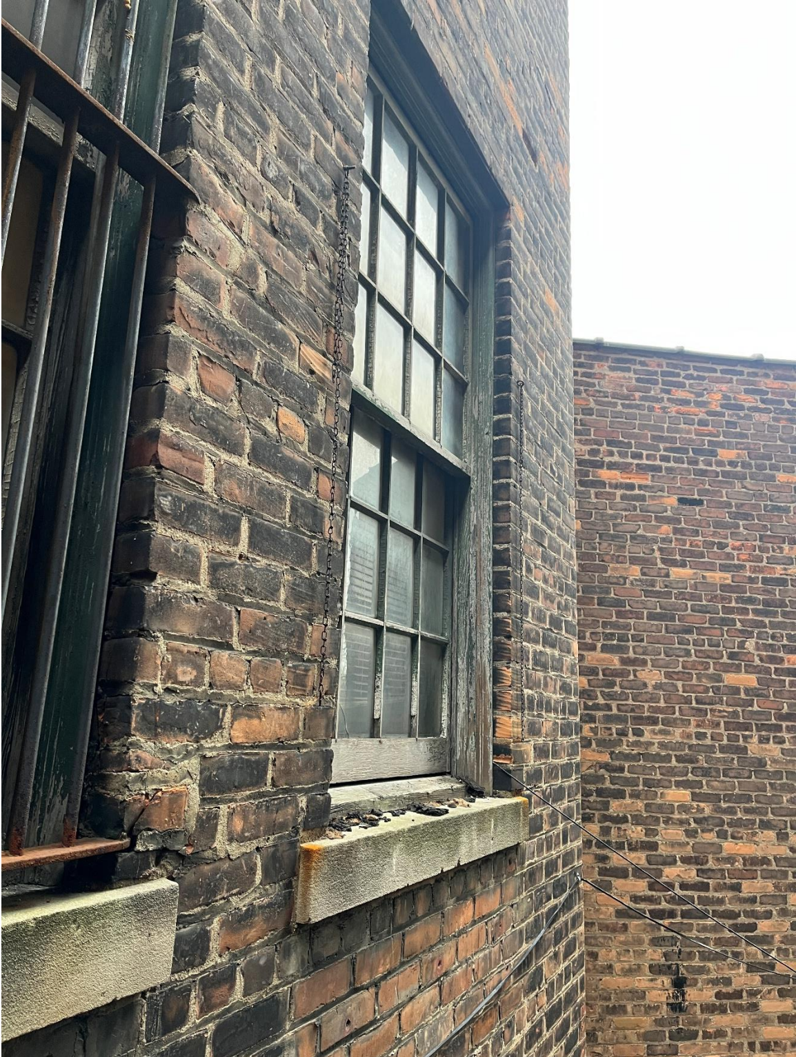
Window 9. 2 nd Floor, alcove, east elevation. Wood unit. 12/11/2024.
