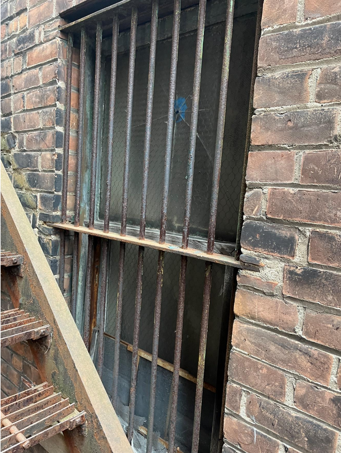
Window 10. 1 st Floor, alcove, east elevation. Cold-rolled steel unit. 12/11/2024.
