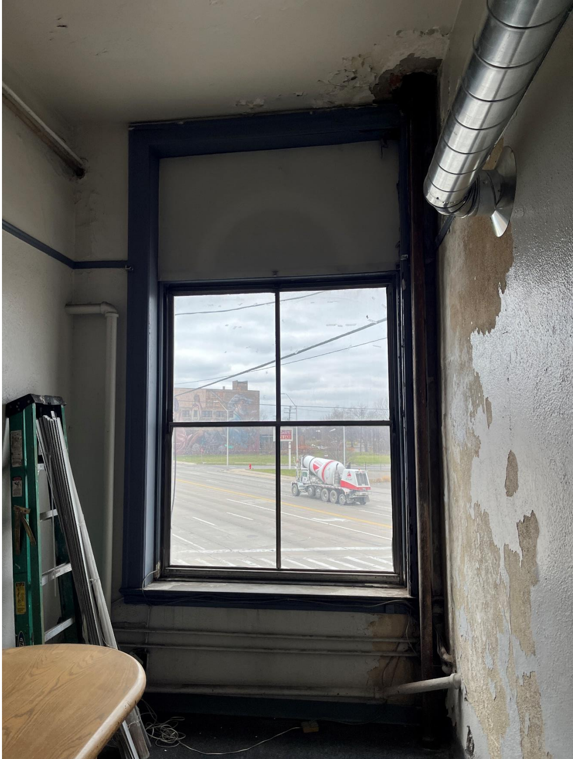
Window 5. 2 nd Floor, south elevation. Aluminum replacement unit. 12/11/2024.
