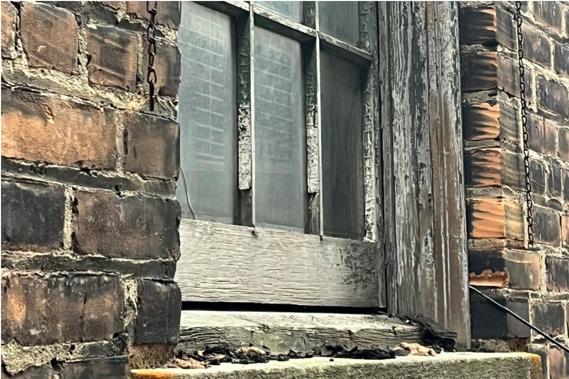
Window 9. 2 nd Floor, alcove, east elevation. Wood unit. 12/11/2024.
