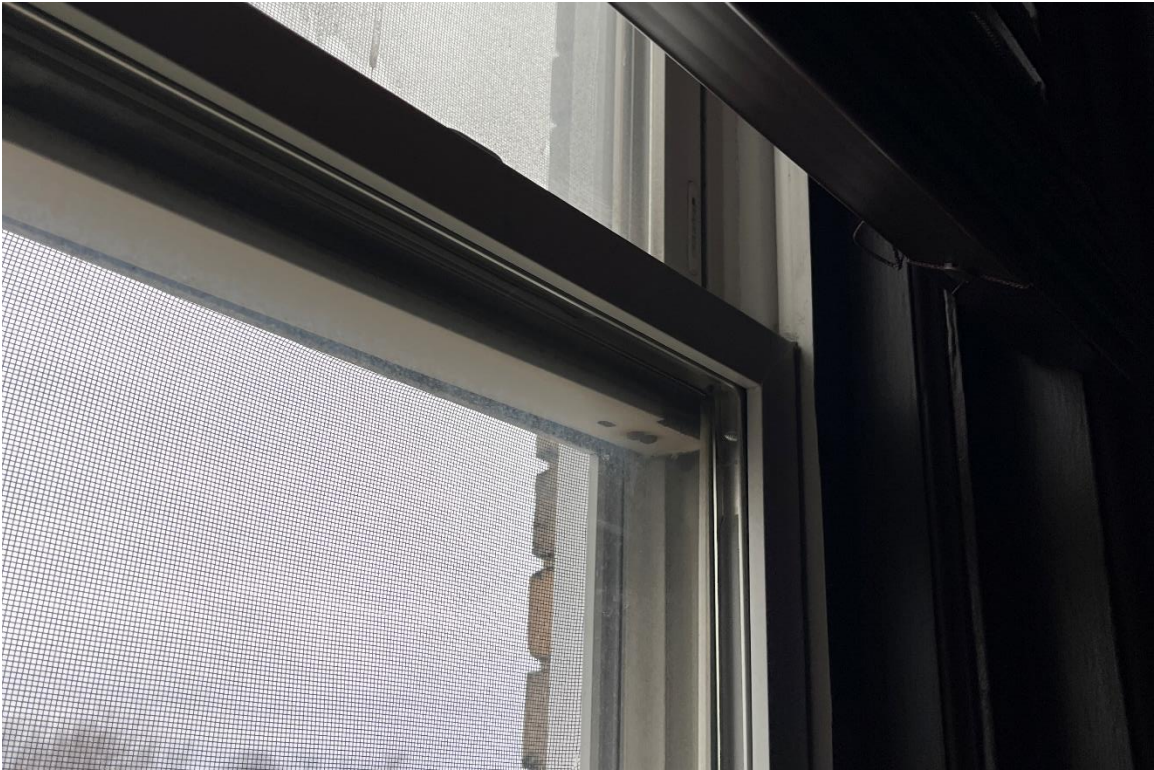
Window 4. 3 rd Floor, south elevation. Vinyl replacement unit. 12/11/2024.
