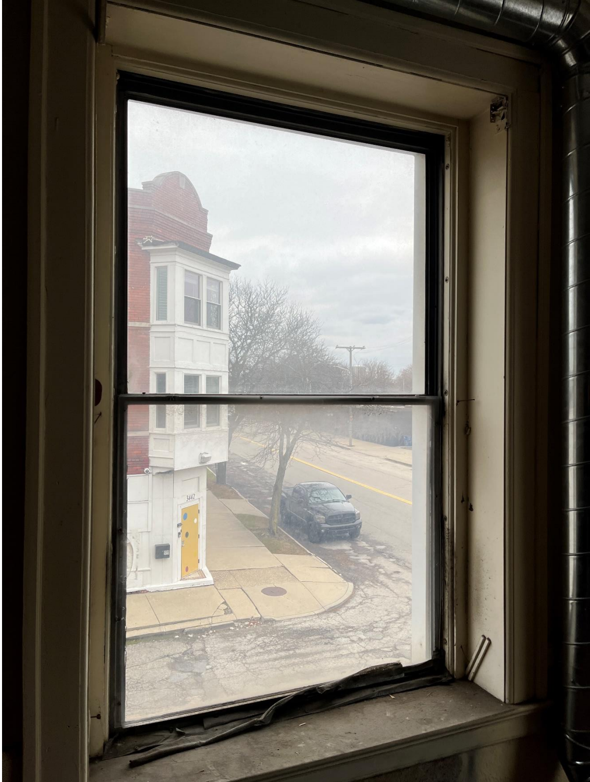
Window 2. 2 nd Floor, east elevation. Aluminum replacement unit. 12/11/2024.
