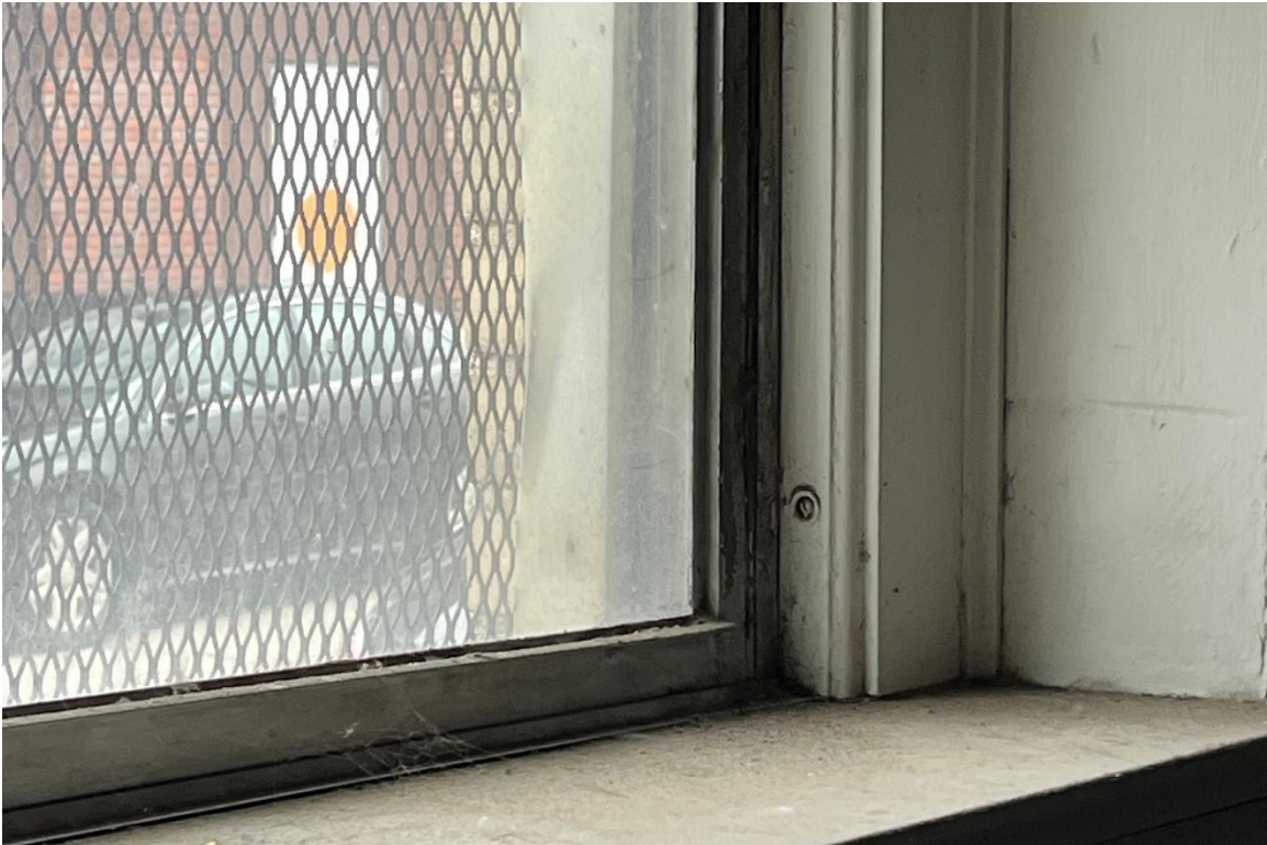
Window 3. 1 st floor, east elevation. Aluminum replacement unit. 12/11/2024.
