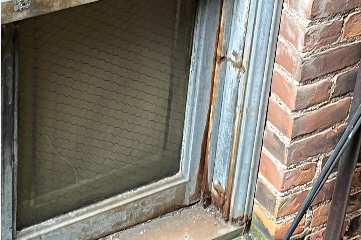
Window 15. 1 st Floor, alcove, west elevation. Cold rolled steel unit. 12/11/2024.
