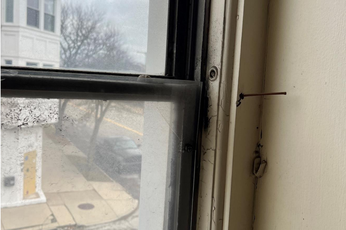
Window 2. 2 nd Floor, east elevation. Aluminum replacement unit. 12/11/2024.
