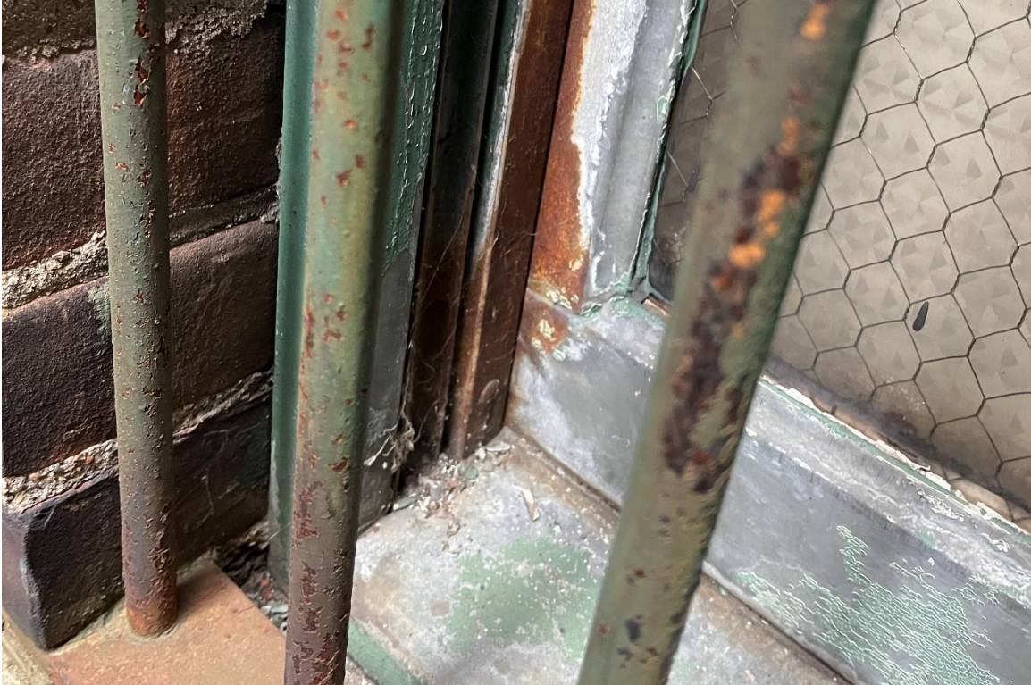
Window 13. 2 nd Floor, alcove, north elevation. Cold rolled steel unit. 12/11/2024.
