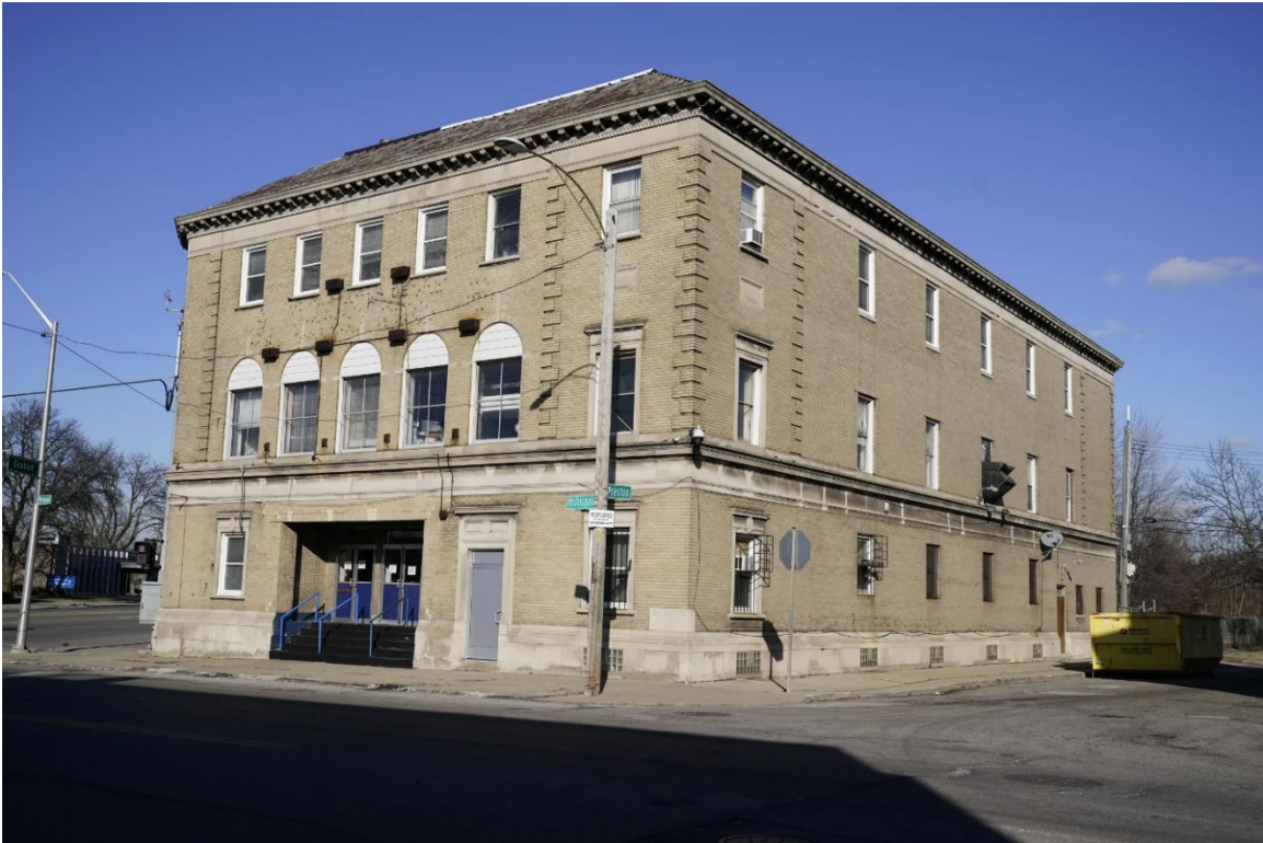
McDougall and Preston facades
