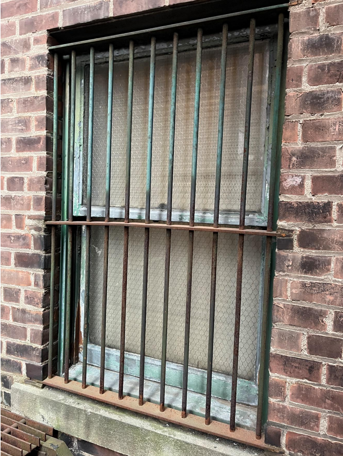
Window 13. 2 nd Floor, alcove, north elevation. Cold rolled steel unit. 12/11/2024.
