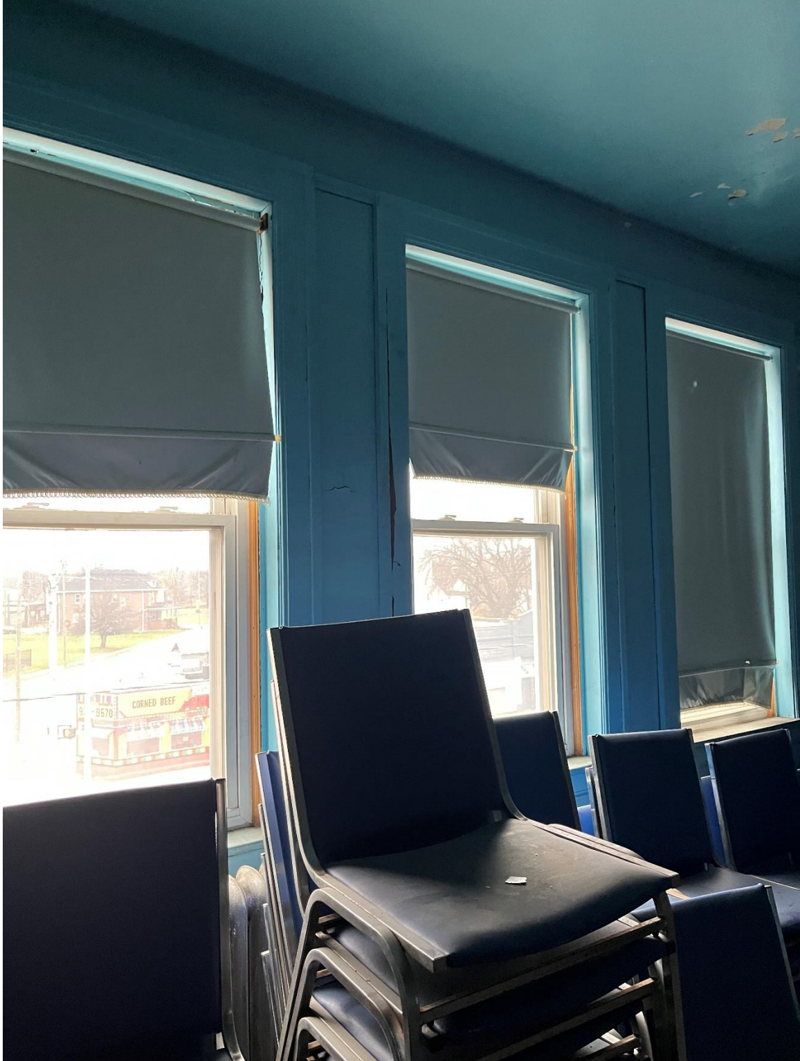
Window 7. 3 rd Floor, west elevation. Vinyl replacement unit. 12/11/2024.
