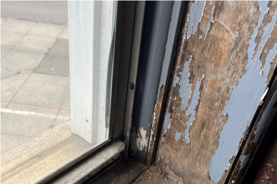
Window 5. 2 nd Floor, south elevation. Aluminum replacement unit. 12/11/2024.
