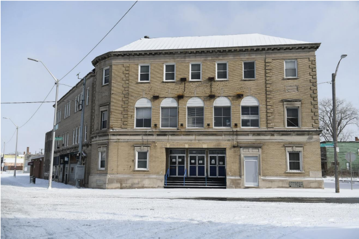
McDougall and Gratiot facades
