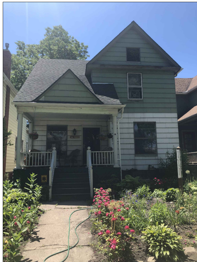
EXISTING PHOTO FRONT OF HOUSE
