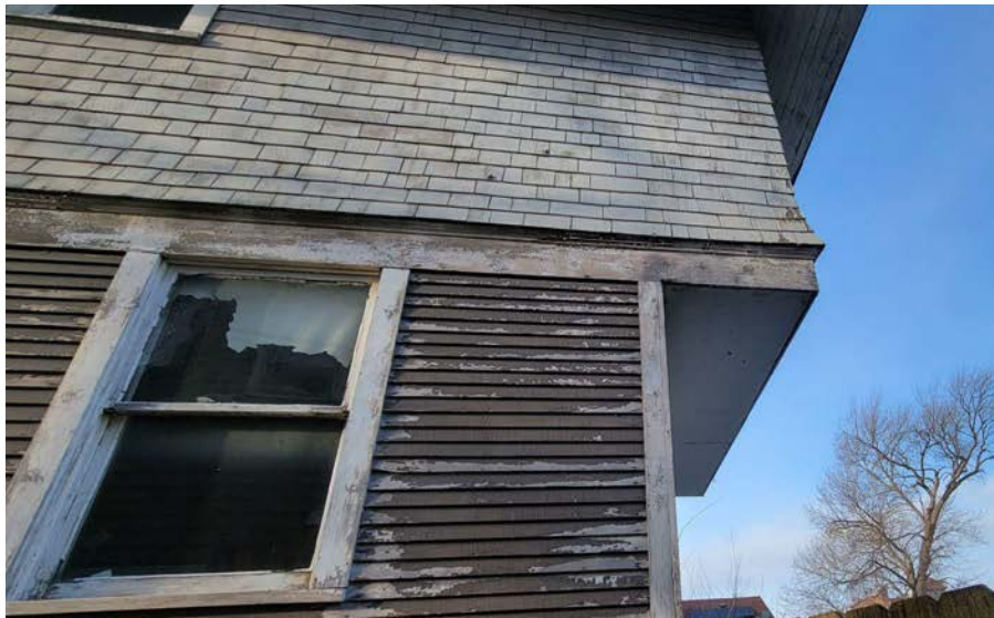
Rear Soffit Detail
