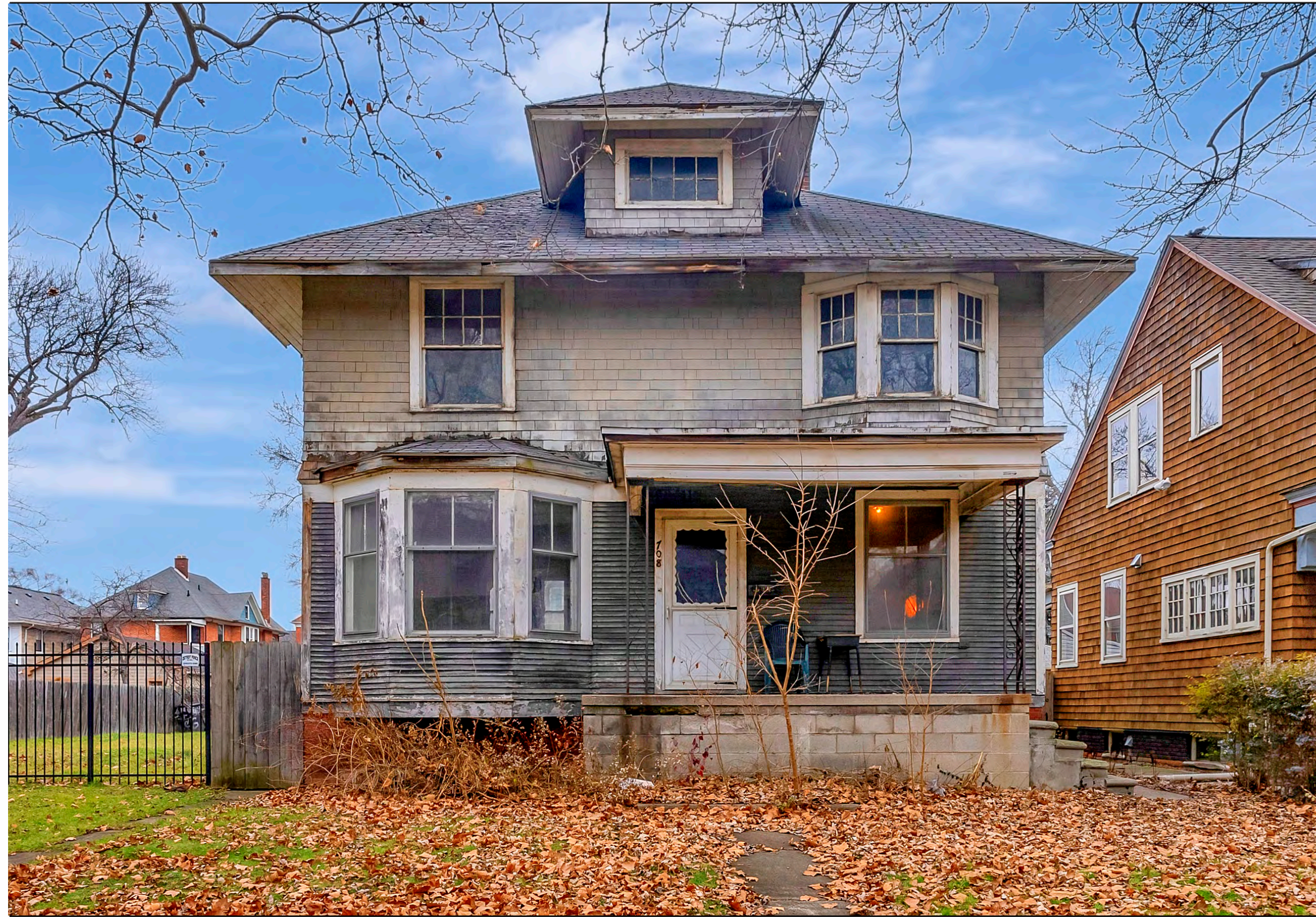
1 SOUTH ELEVATION - JANUARY 2024
