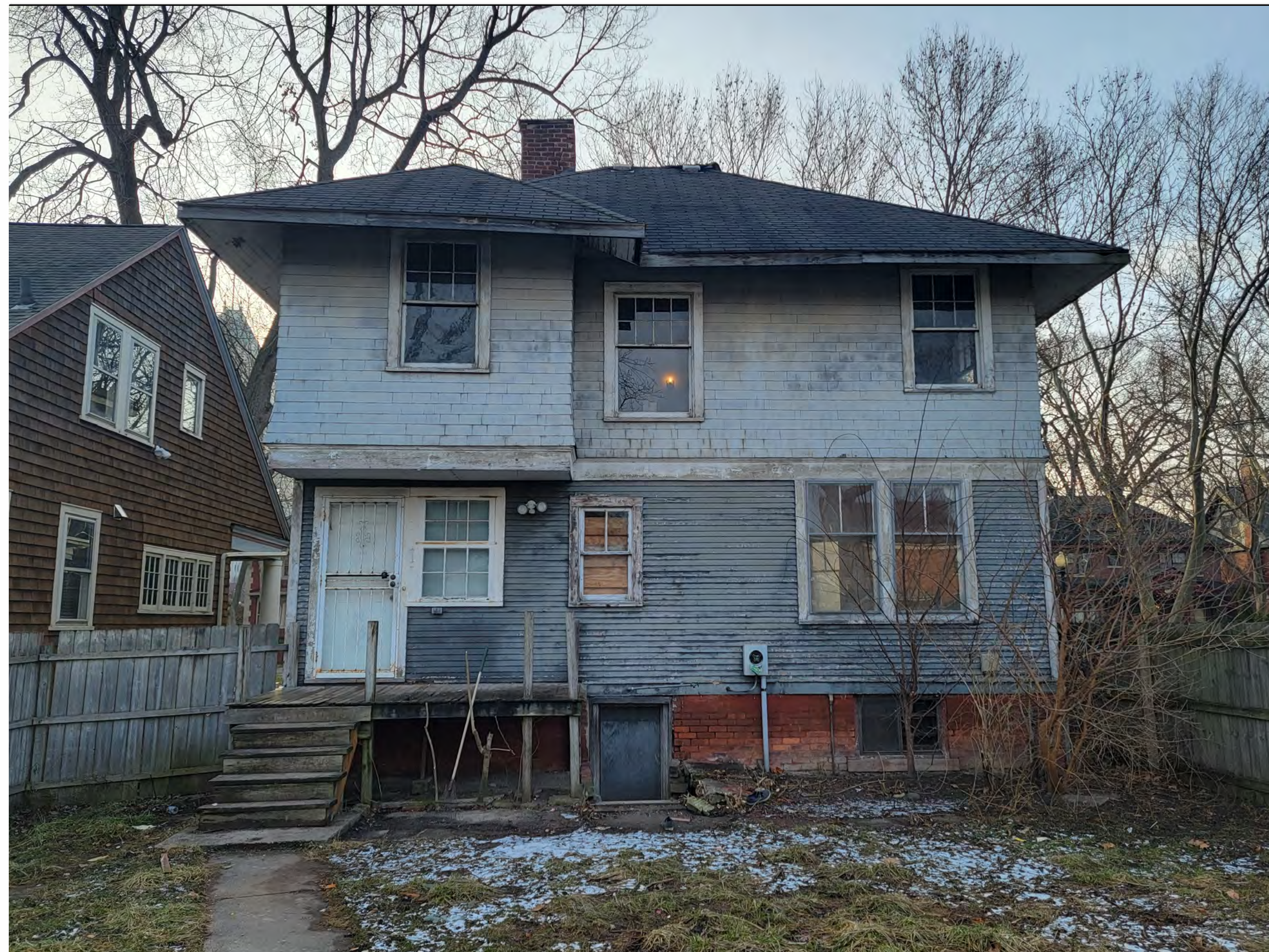
2 NORTH ELEVATION - JANUARY 2024
