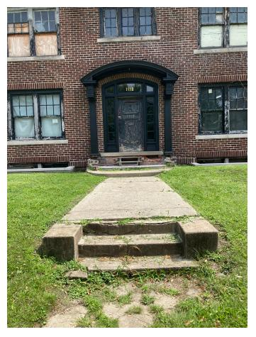
Current front with crumbling stairs and porch that needs to be replicated. Note the template we built to keep the same shape of the steps as was there. This was not salvageable.
