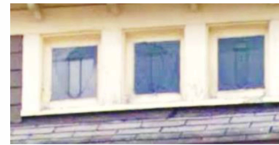
ORIGINAL DORMER WINDOW
