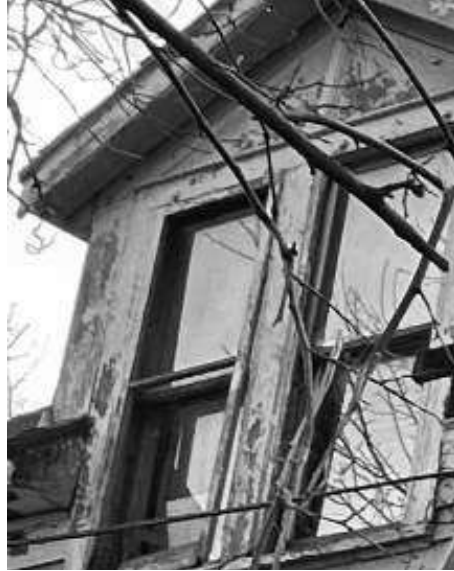
Side Window / Second floor
