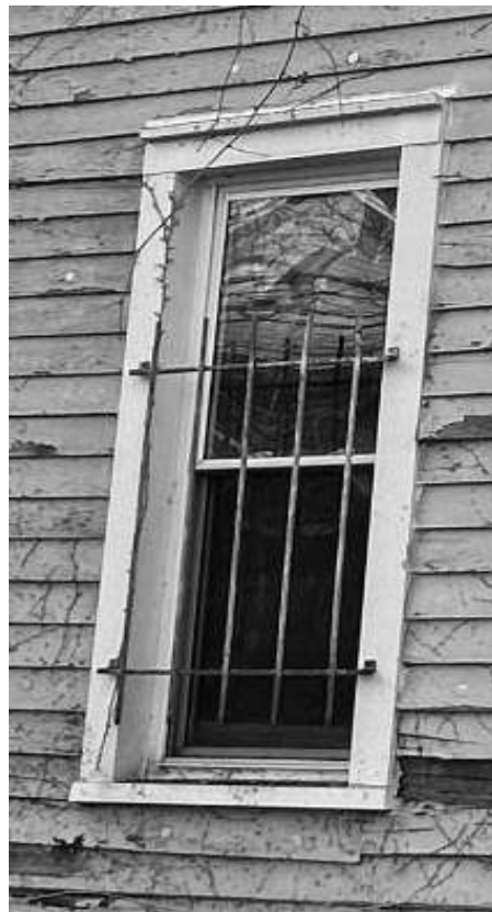
Side Window / First floor
