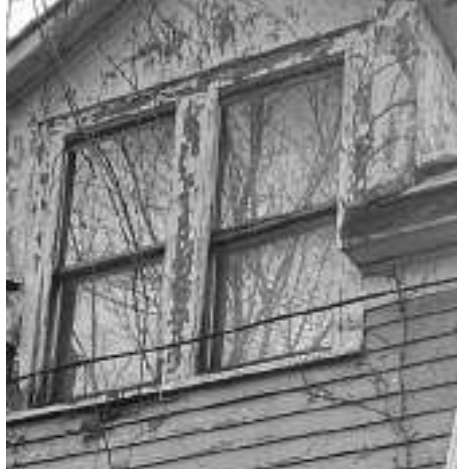
Side Window / Second floor
