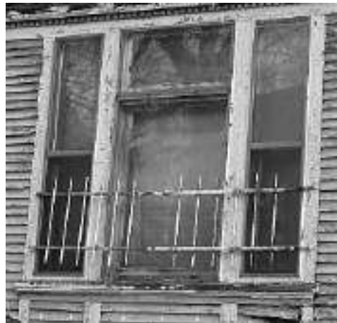
Front Window / First floor
