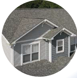
Roofing and Ventilation
