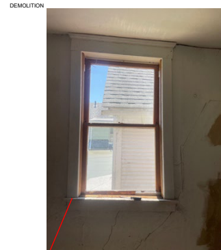
EXISTING WINDOW: Wood (28"x54")
