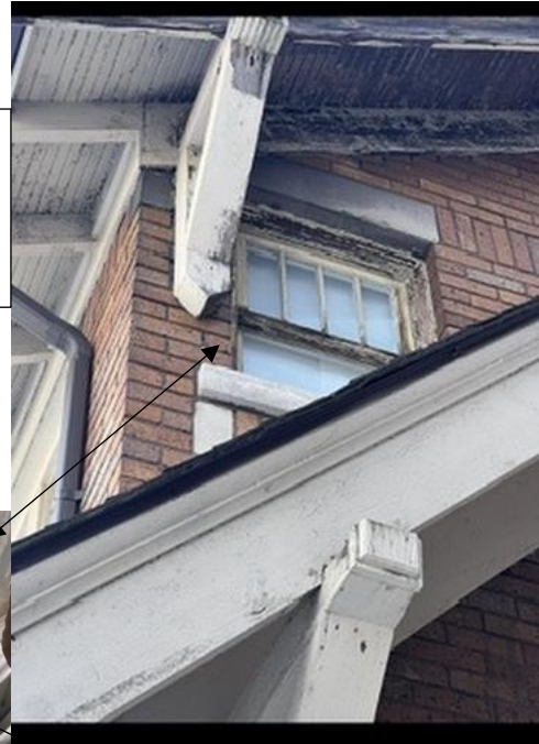
Metal bars drilled into the jambs of the window frame
