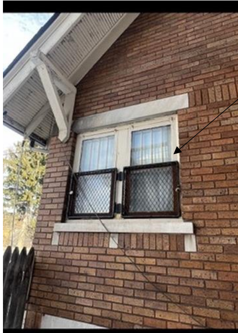
Metal bars drilled into the jambs of the window frame
