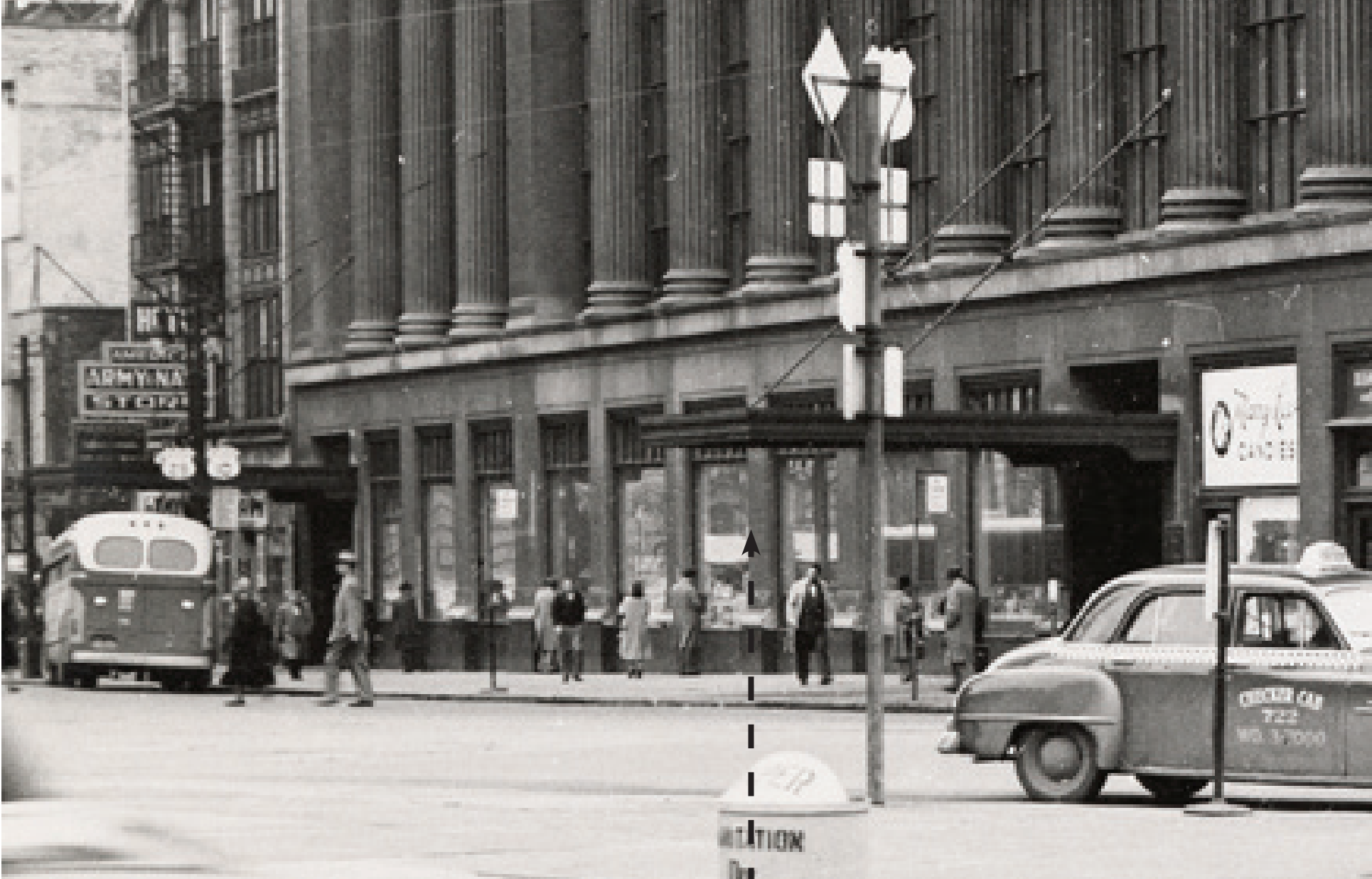
HISTORIC GROUND FLOOR CLADDING IS LIMESTONE. EXIST GRANITE FACING ON GROUND FLOOR IS NON-HISTORIC
