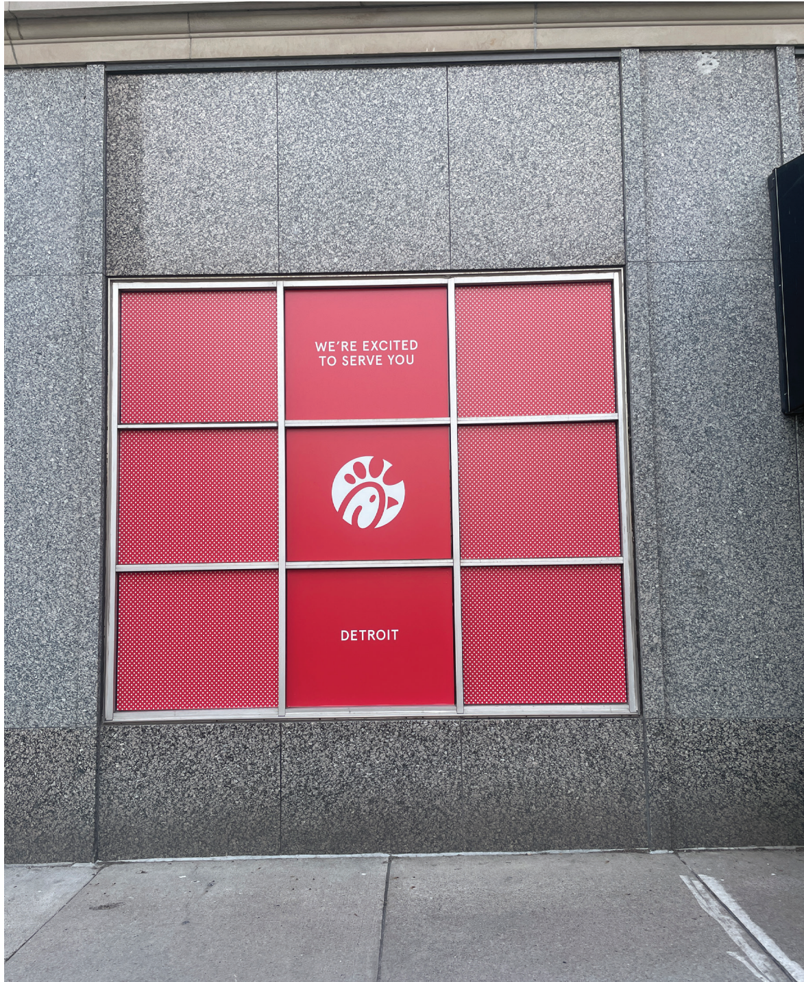
Existing storefront bay, location of proposed new door. Non-historic storefront and non-historic granite base and infill.
