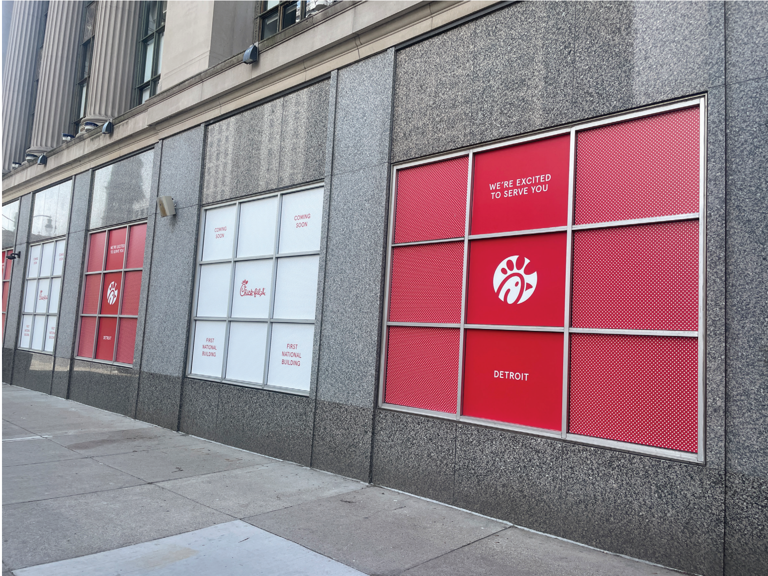
north elevation, looking southeast
