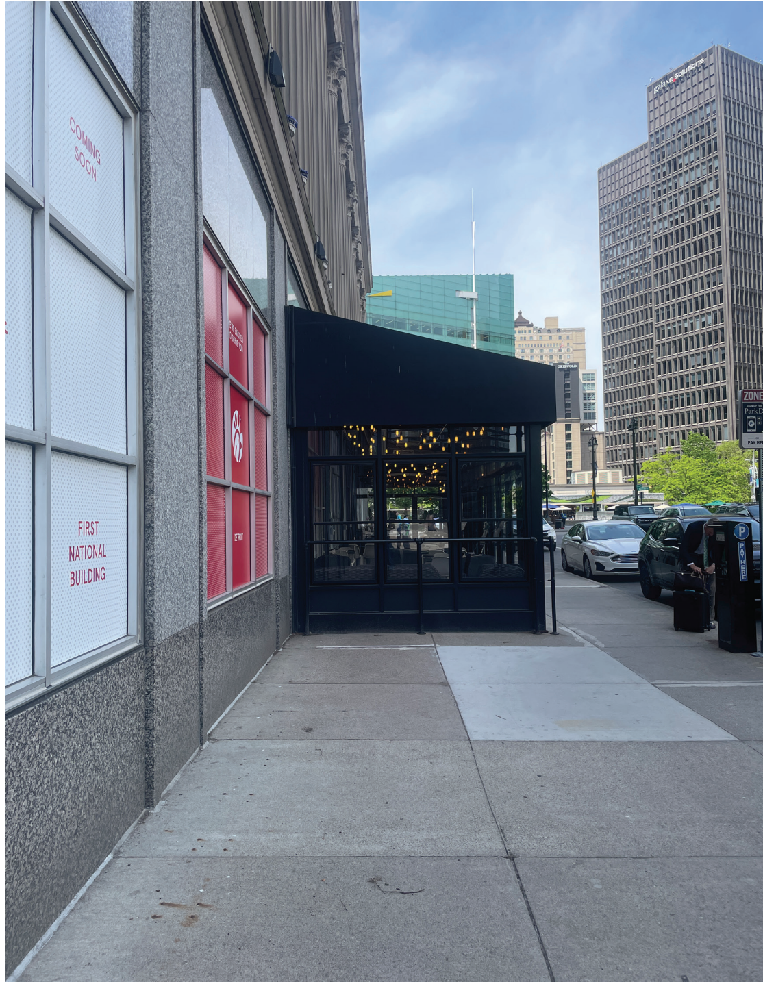
Location of proposed new accessible ramp. Existing permanent structure in background.
