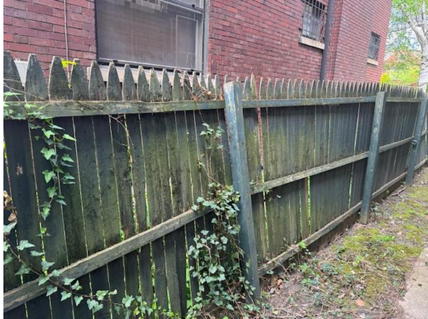
**Bowling falling back at support beams
