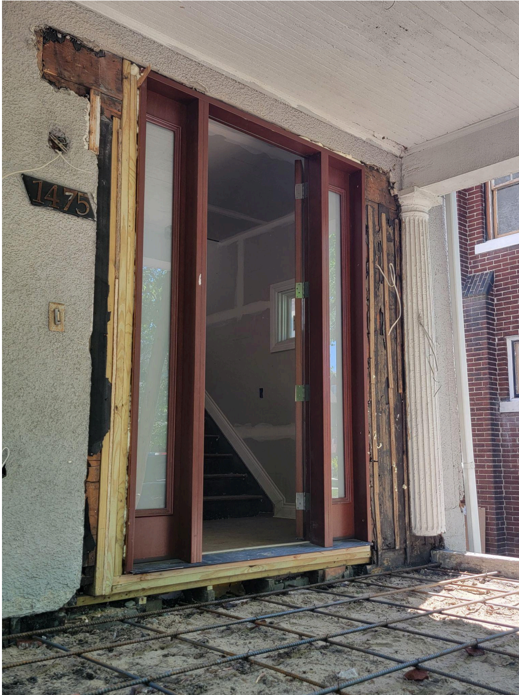
Existing Front Door North Elevation
