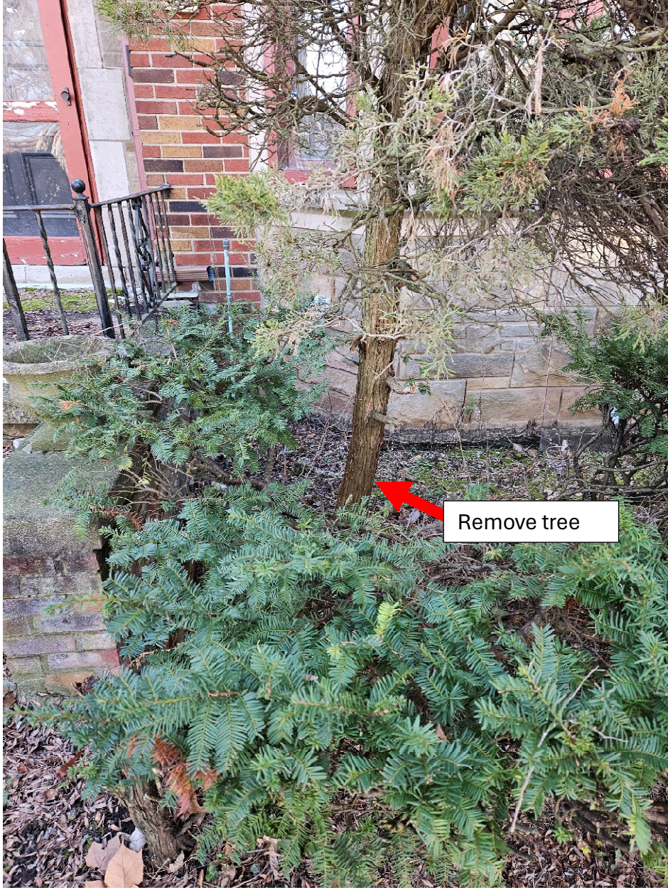
House North Elevation - Remove small tree near foundation wall
