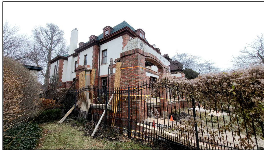
West Elevation of Front Porch / Driveway
