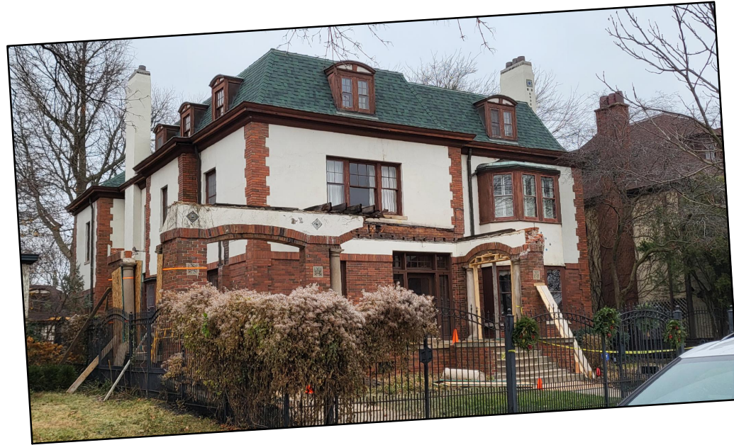
Current State of Front Porch
