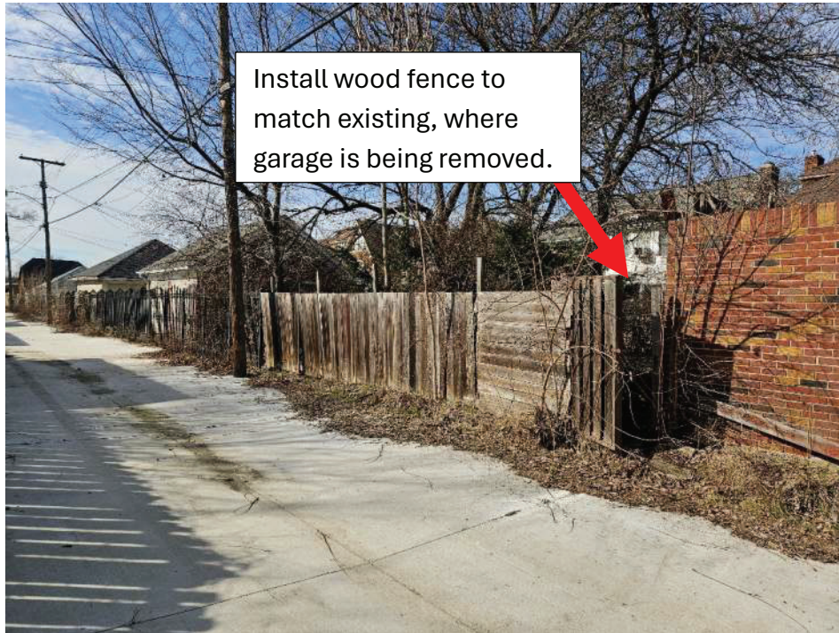
Existing wood fence at the alley
