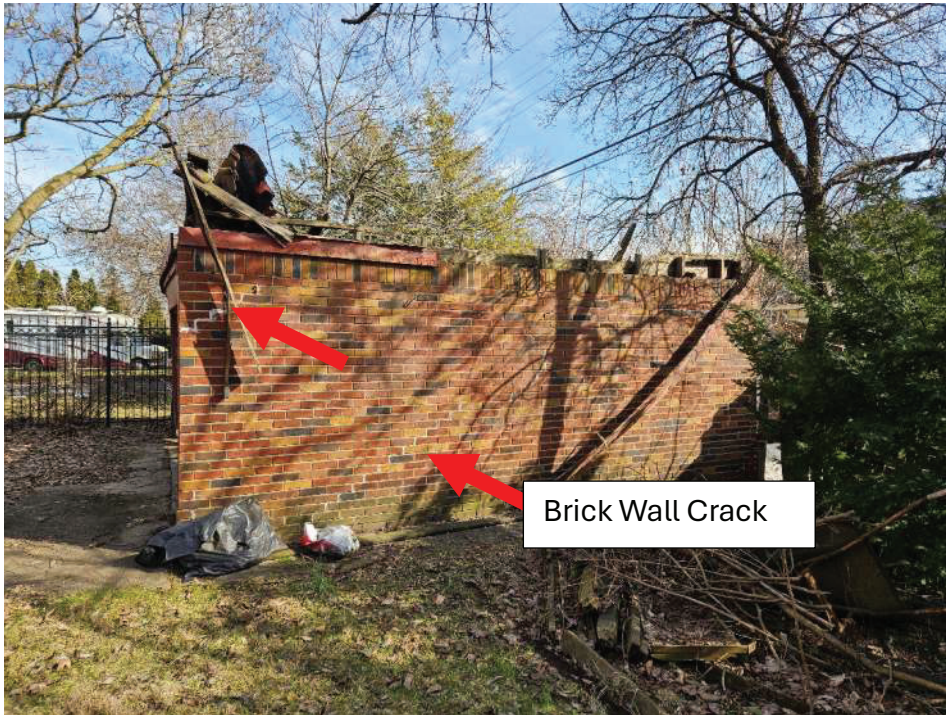
Garage West Elevation – Overview
