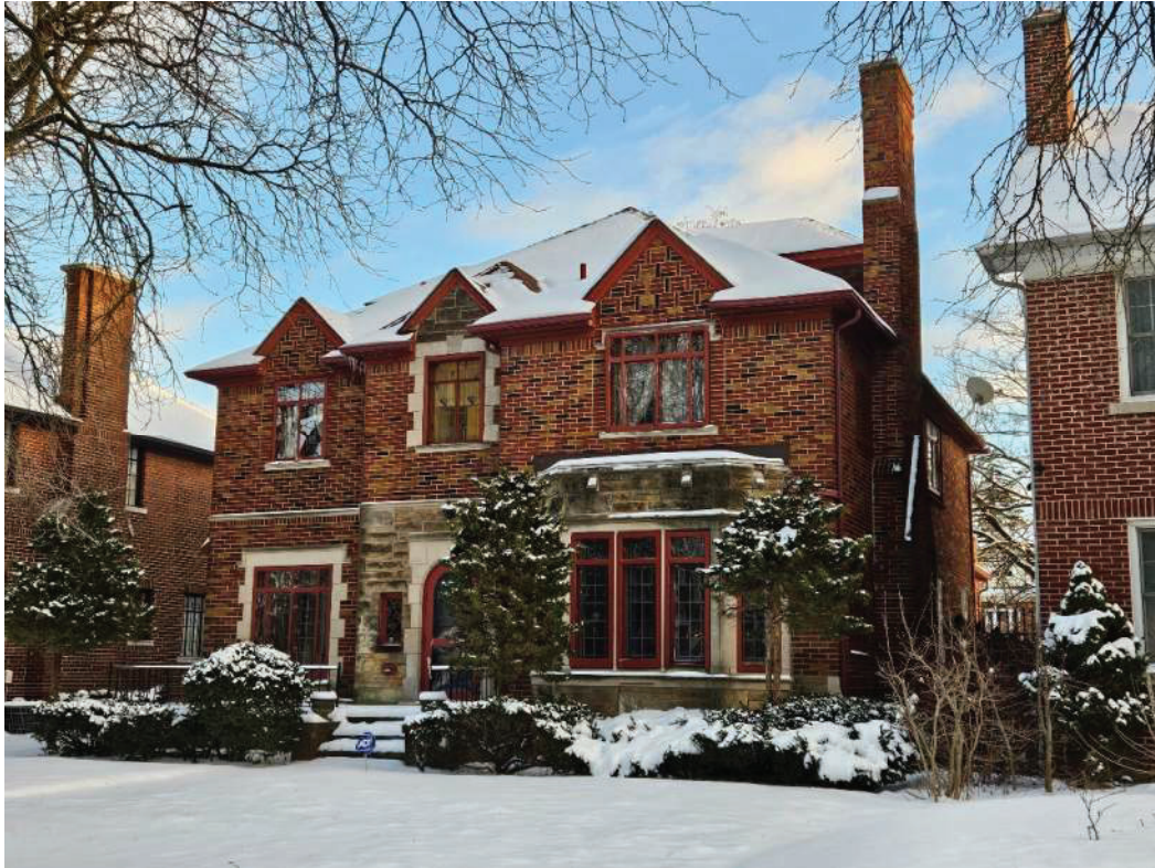
Overview Photo of the North Elevation
