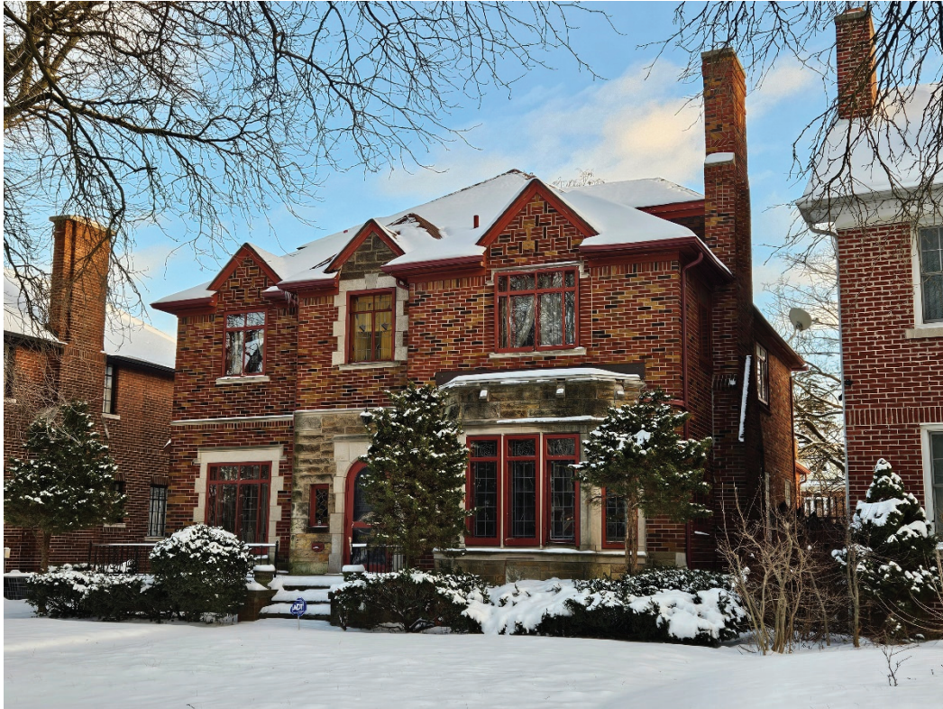
Overview Photo of the North Elevation
