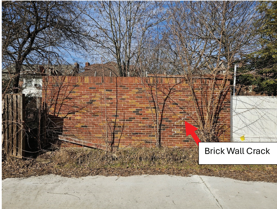
Garage South Elevation – Overview
