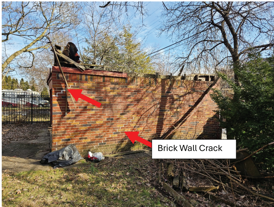
Garage West Elevation – Overview
