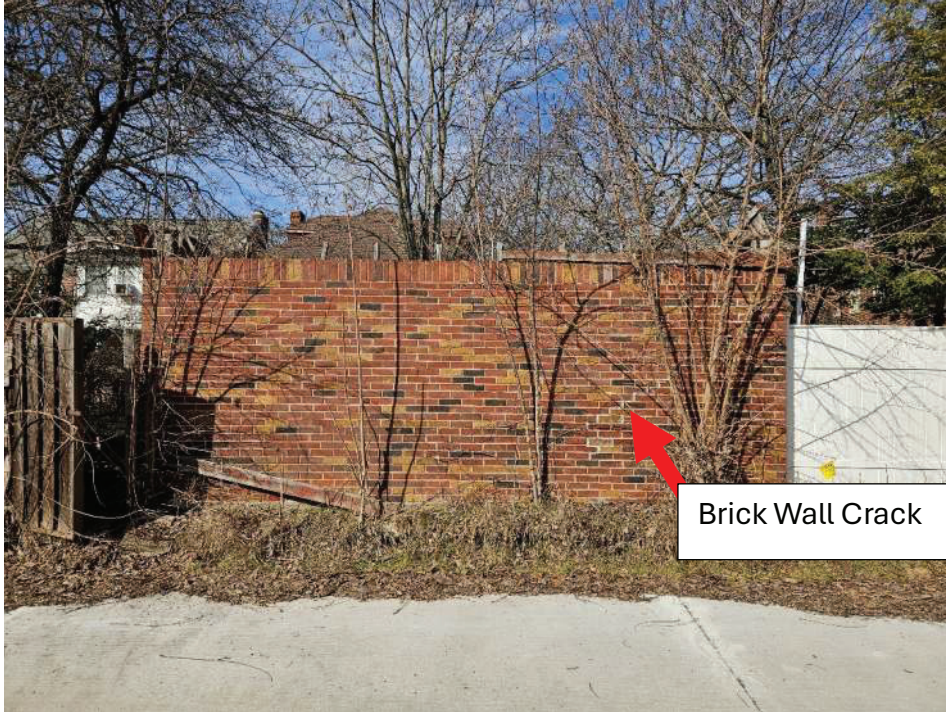
Garage South Elevation – Overview
