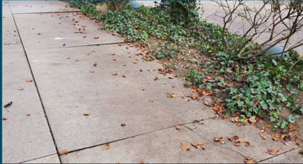
A. Perimeter sidewalk: Where cracked, will be removed and replaced. If in good condition, will be power-washed.
