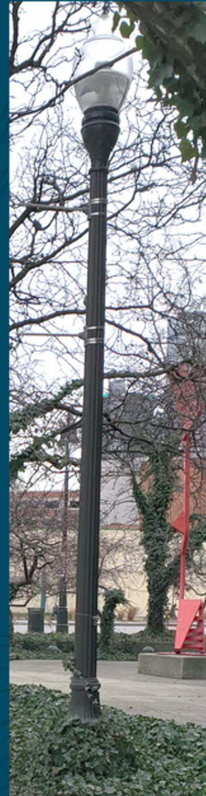
C. Perimeter Pole Luminaires: Acorn top lights to remain, upgrade to LED fixtures. Ornamental fluted poles and bases to be repainted. Where fixtures are damaged, will be replaced in kind.
