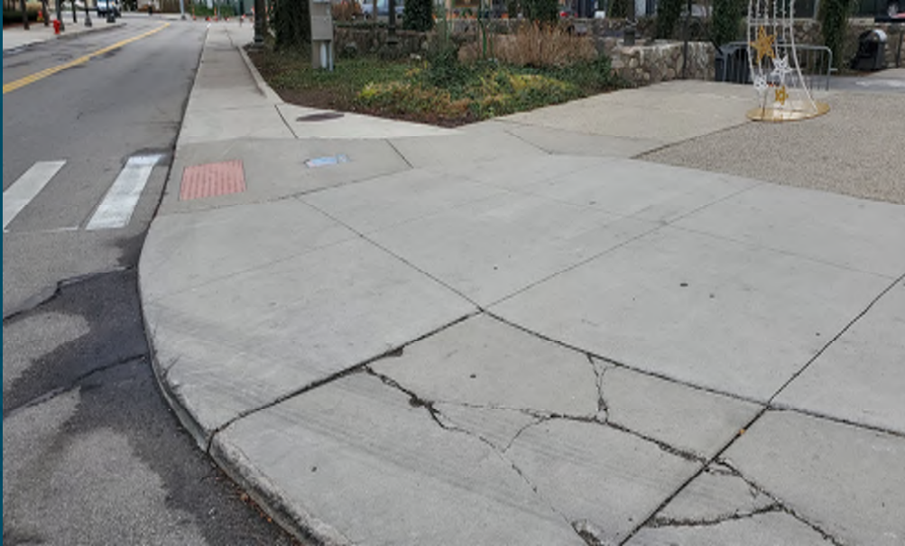
A. Perimeter sidewalk: Where cracked, will be removed and replaced. If in good condition, will be power-washed.
