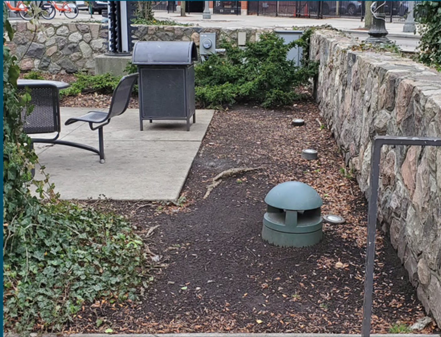
K. Interior uplights in pavers, wall washers, and tree uplights would be removed and replaced with LED fixtures, as well as the light under the concrete stage.
