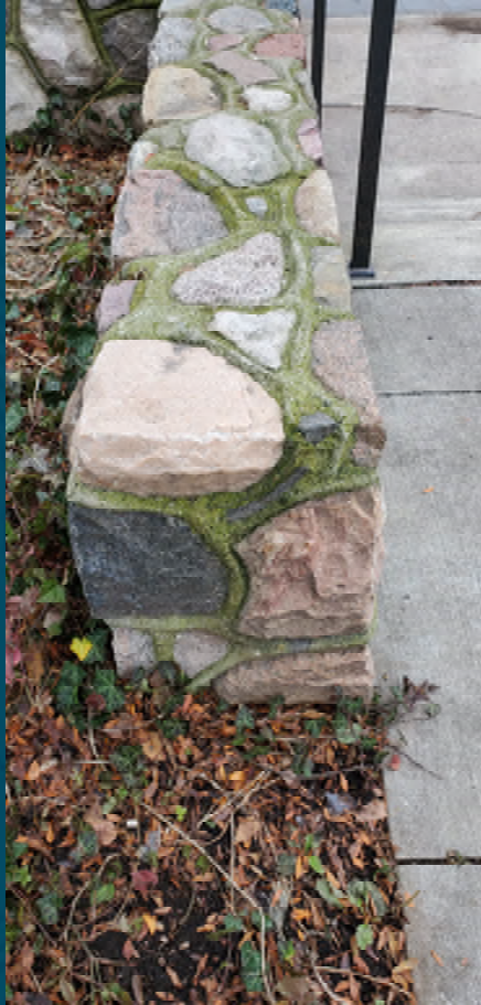
D. Stone Walls: Will be cleaned, mortar replaced and re-pointed to restore to original condition.
