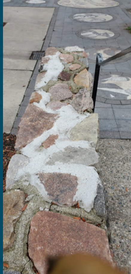
D. Stone Walls: Will be cleaned, mortar replaced and re-pointed to restore to original condition.
