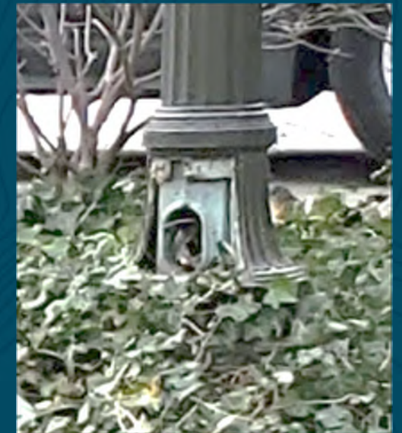
C. Perimeter Pole Luminaires: Acorn top lights to remain, upgrade to LED fixtures. Ornamental fluted poles and bases to be repainted. Where fixtures are damaged, will be replaced in kind.
