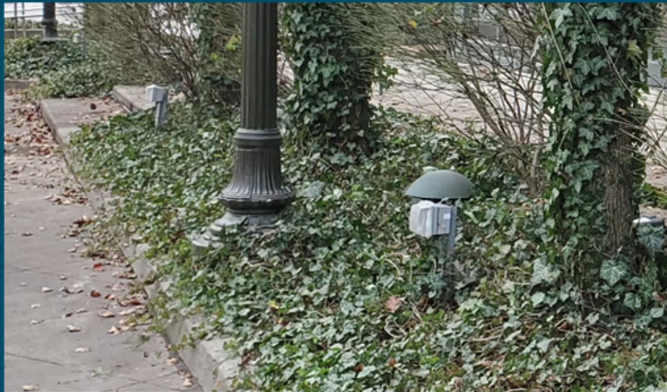
Y. Power pedestals to be replaced.
