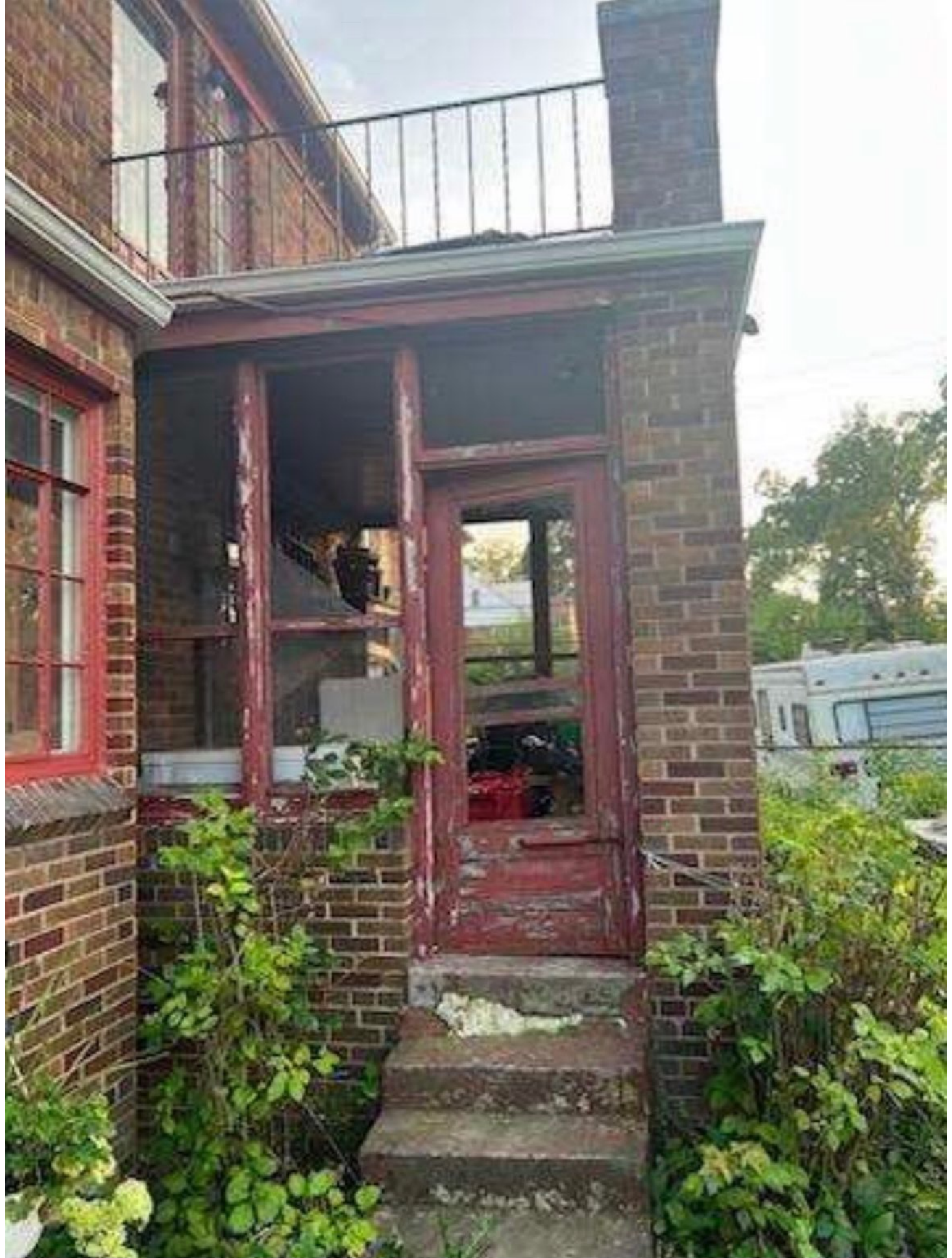
East wall: "bank of 2-windows" & 1-stationary/fixed window above doorway
