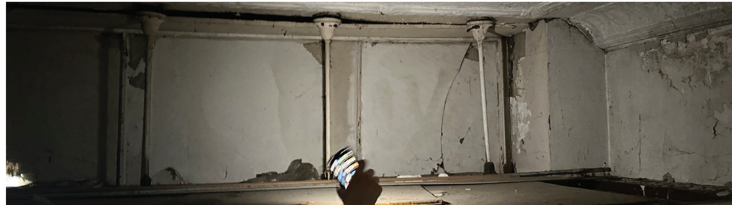
INTERIOR VIEW OF TRANSOM
