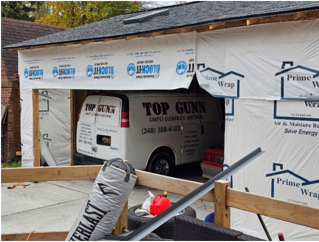
View from Deck to Garage
