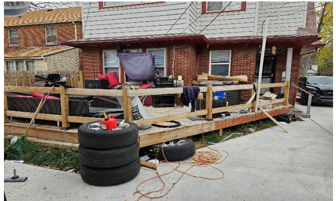
View of deck
