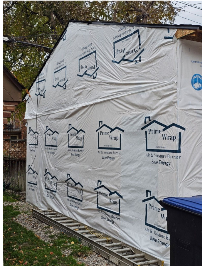
Left side of Garage with gravel
