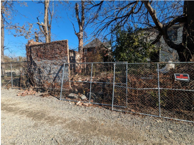
Remnants of an old accessory building north in the alley
