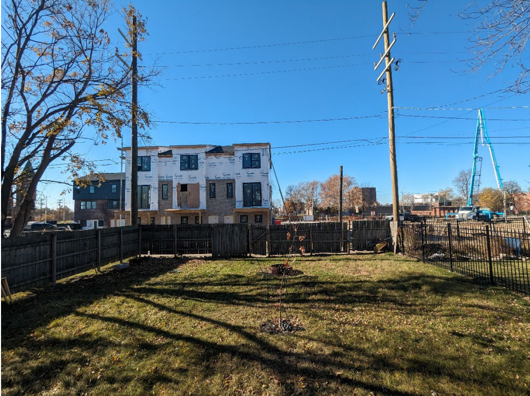
Ground Level view
