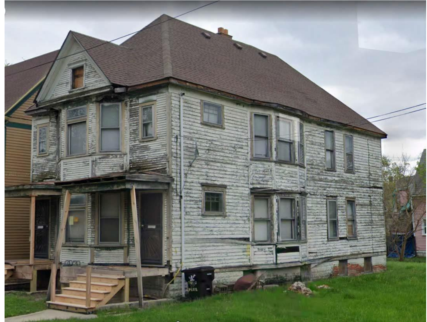
PREVIOUS CONDITION OF 7908 SAINT PAUL BEFORE SIDING AND WINDOWS WERE REMOVED; IMAGE FROM 2019 - FRONT & SIDE ELEVATIONS
