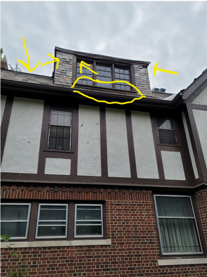
Exhibit 7. Front dormer apron, walls, flat roof
