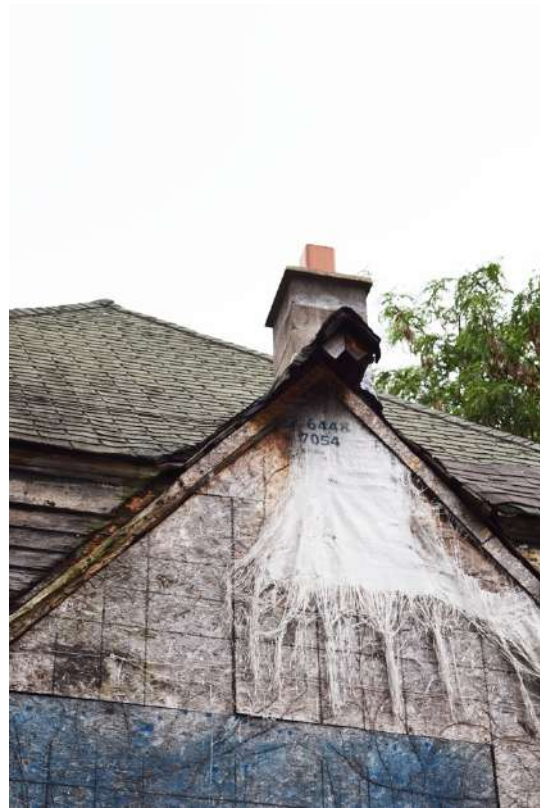
Rear coal chimney proposed for removal
