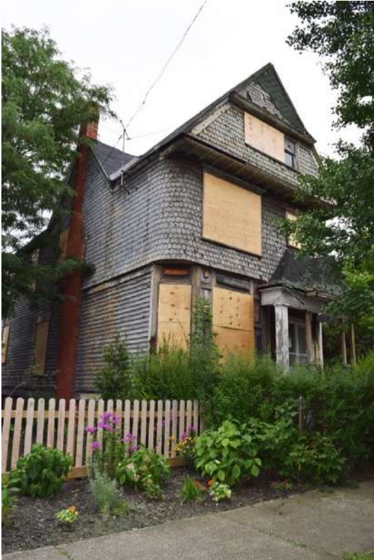
Front Façade looking East
