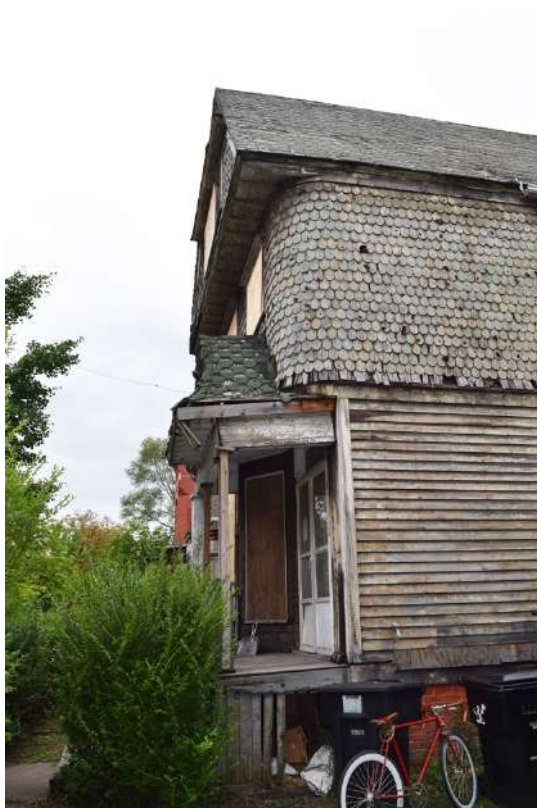
Front porch / South Façade from side yard.
