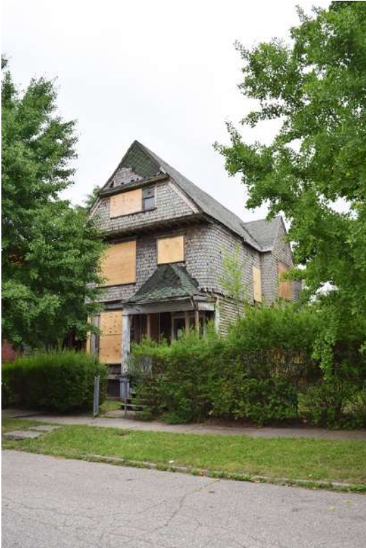
Front Façade looking North
