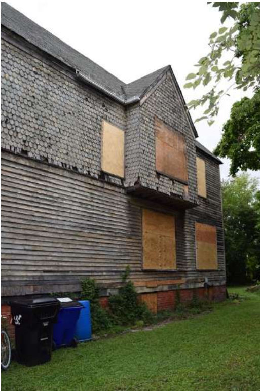
South Façade from side yard
