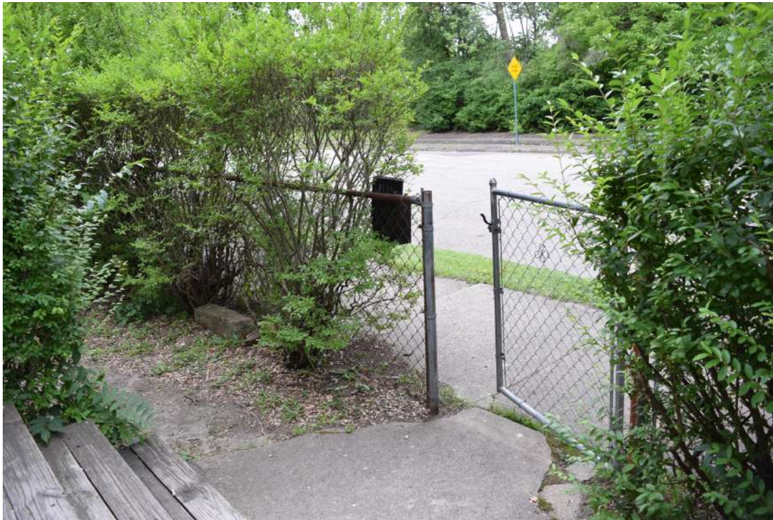
Front chain link fence proposed for removal
