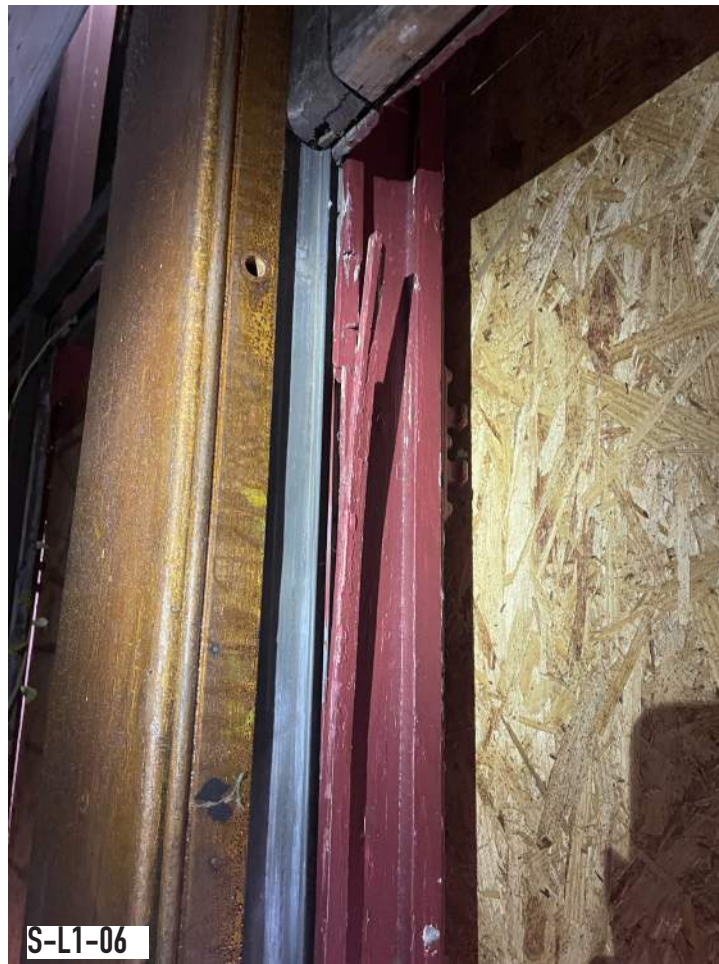
S-L1-06 LOWER SASH OUT OF PLANE
