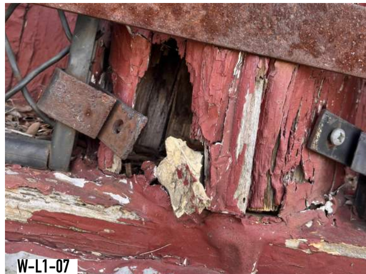
TYPICAL ROTTED BRICK MOLD AT BASE RESULTING FROM SAFETY SCREEN MOUNTING BRACKETS FASTENERS
