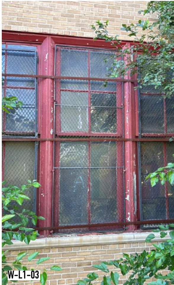
INTACT BRICK MOLD REQUIRING NEW PAINT AND CAULK ABATEMENT
