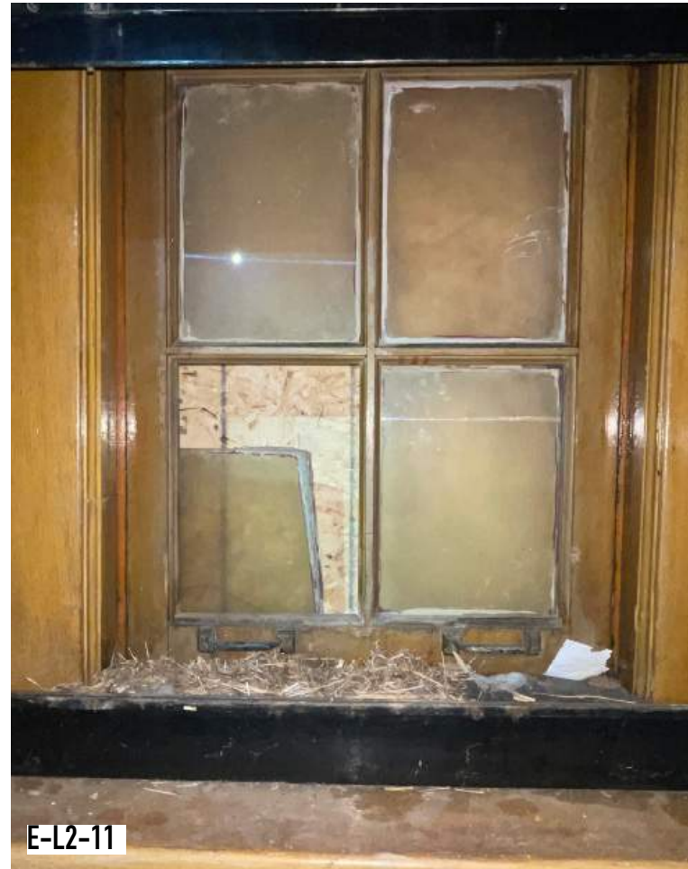
WINDOW REQUIRING REPLACEMENT GLASS, FINISH IN FAIR CONDITION
