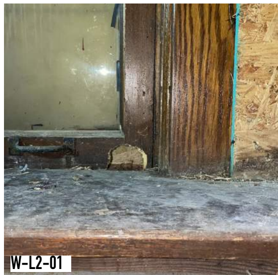
MOUSE HOLE IN SASH RAIL
