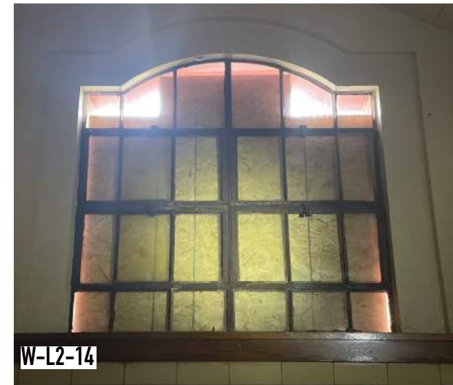
DECORATIVE STEEL WINDOW WITH MINOR RUST REQUIRING PAINT AND REPLACEMENT GLASS
