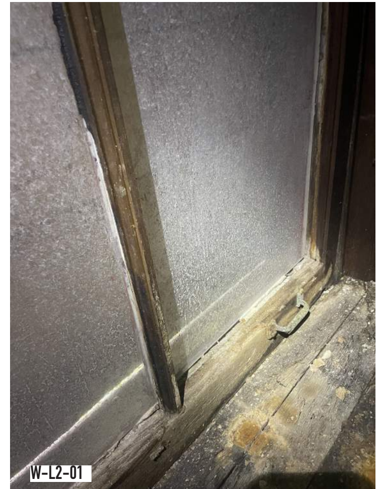
ROTTED INTERIOR SILL AND SASH DUE TO WATER INTRUSION
