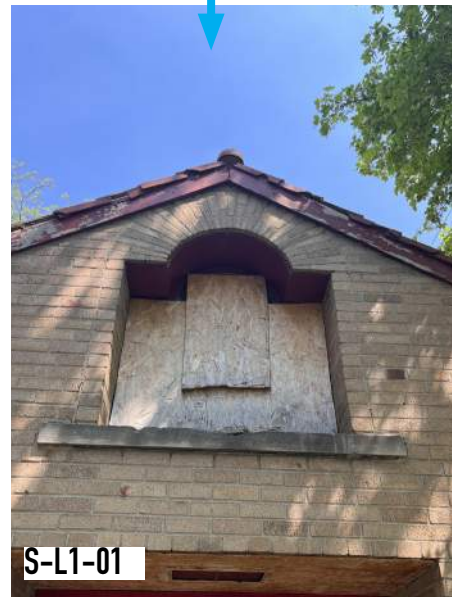
S-L1-01 EXISTING FIXED DECORATIVE STEEL WINDOW
