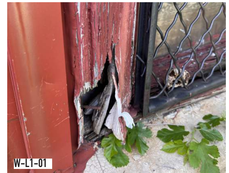
TYPICAL ROTTED BRICK MOLD DUE TO INSTALLATION OF FIRE WINDOWS
