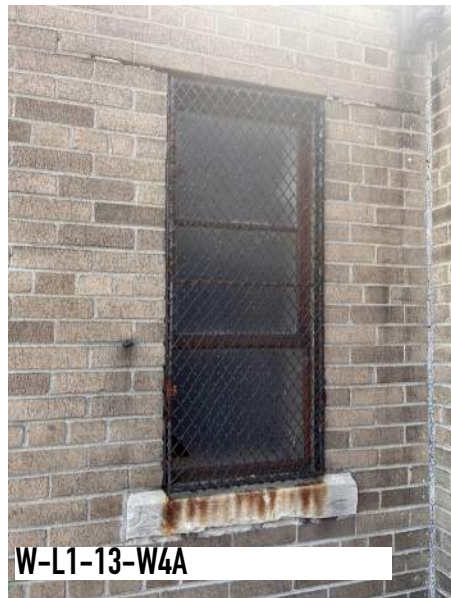
W-L1-13-W4A STEEL HOPPER WINDOW
