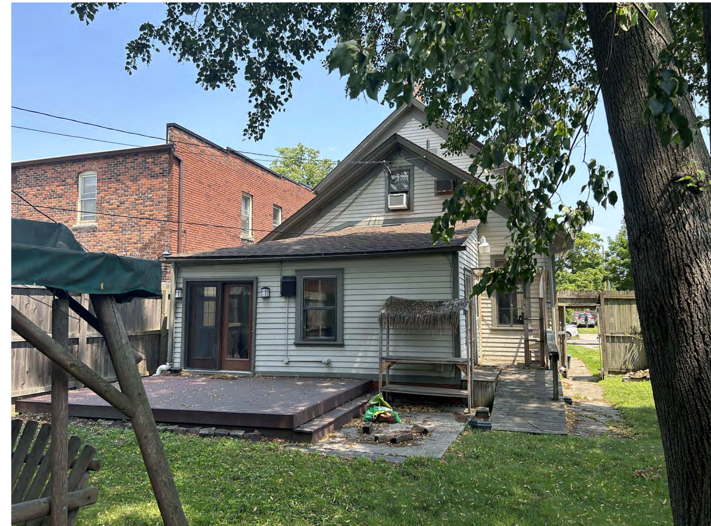
3. VIEW OF REAR LOOKING EAST (JULY 2023)
