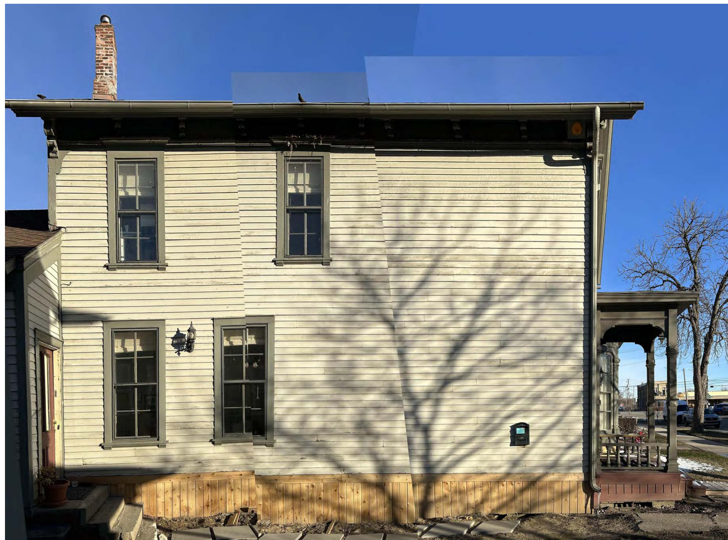
4. PARTIAL SOUTH ELEVATION AT FRONT SECTION OF BUILDING (MARCH 2023)
