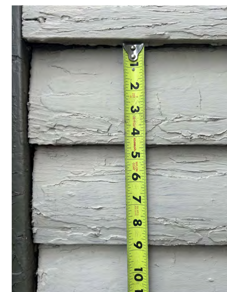
7. PHOTO OF EXISTING CONDITIONS
