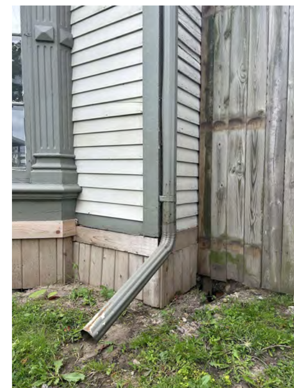
5. EXISTING CONDITION IMAGE OF DOWNSPOUT
