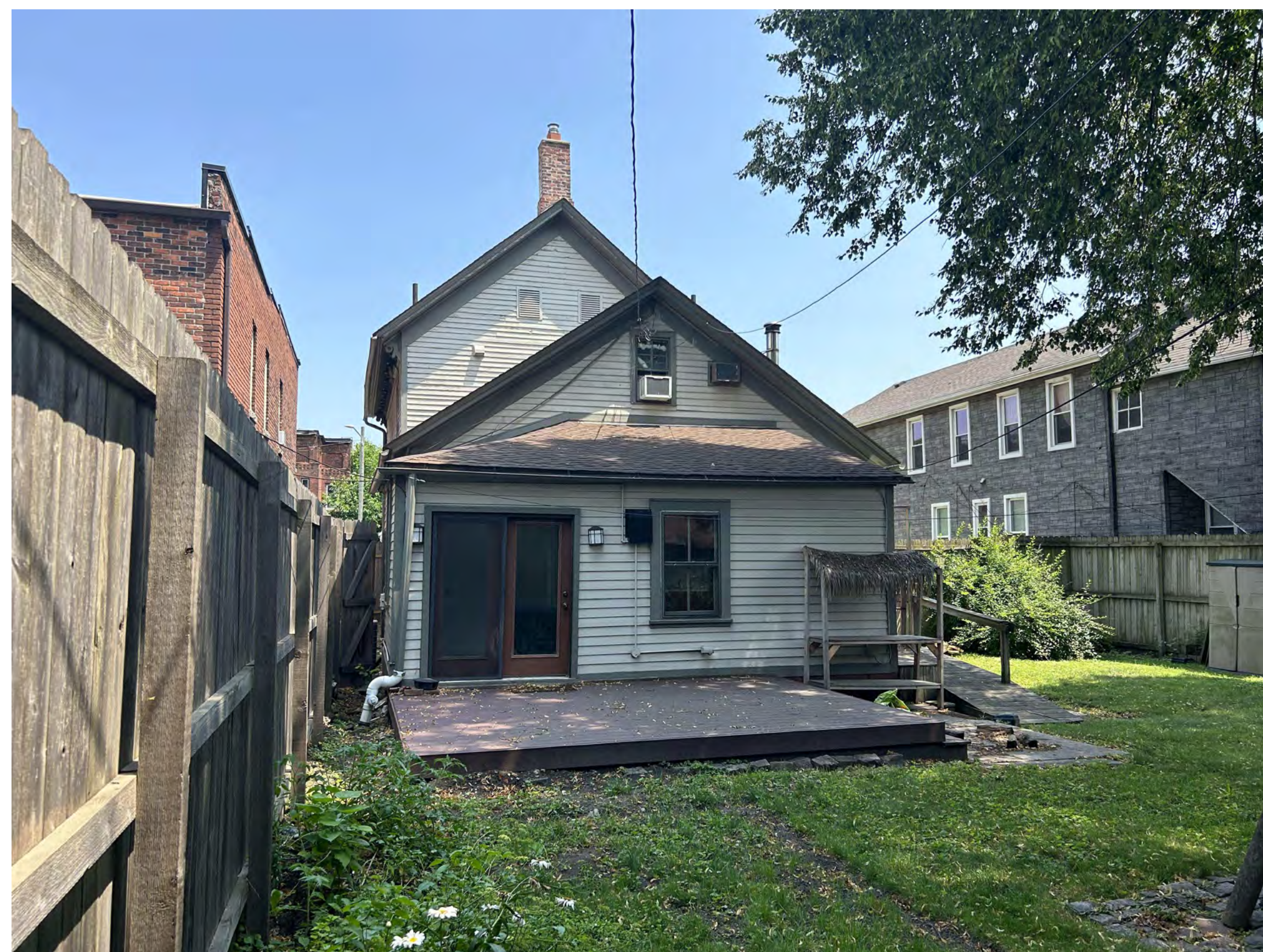
4. VIEW OF REAR LOOKING EAST (JULY 2023)
