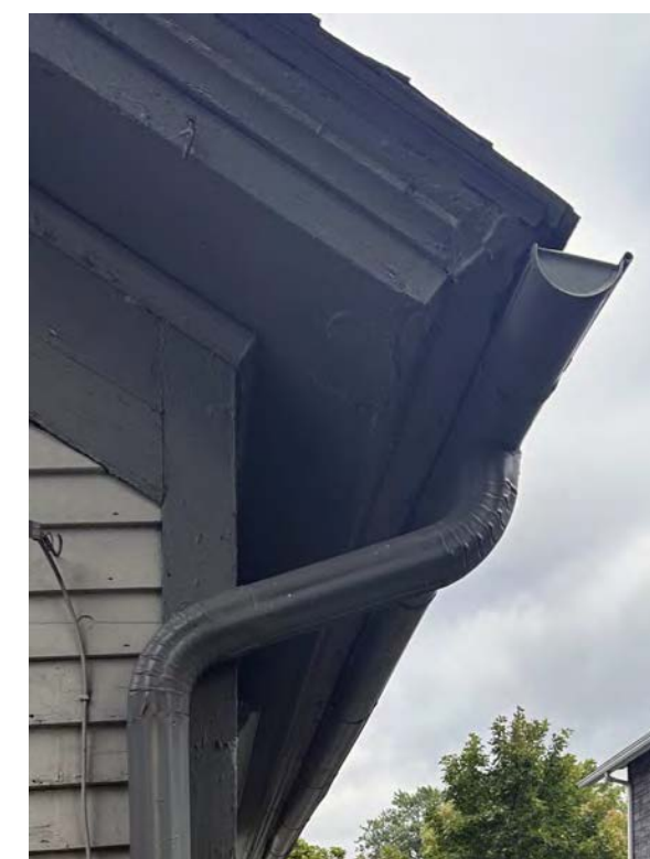
4. EXISTING CONDITION IMAGE OF GUTTER & DOWNSPOUT
