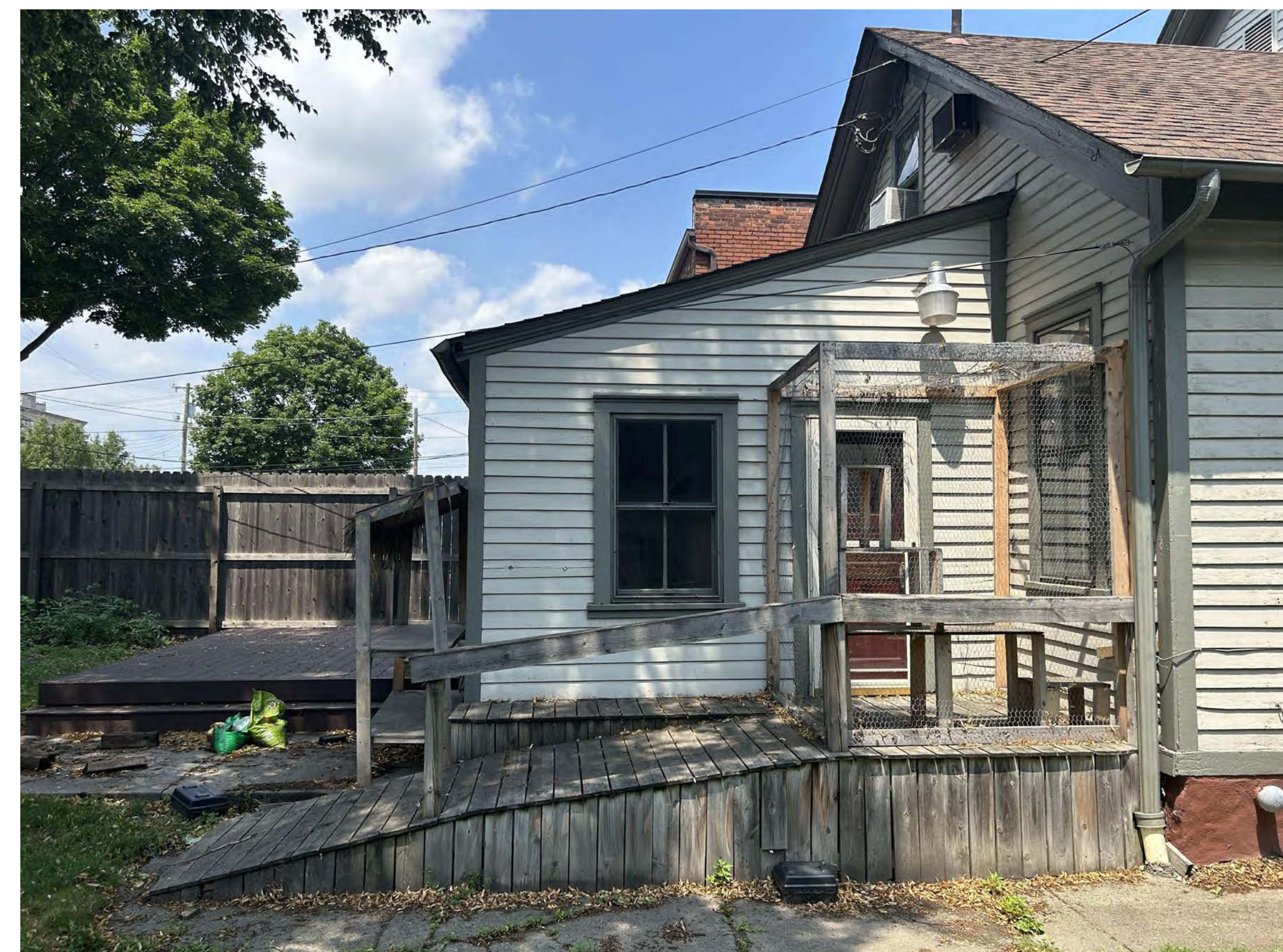
5. VIEW OF REAR LOOKING NORTH (JULY 2023)
