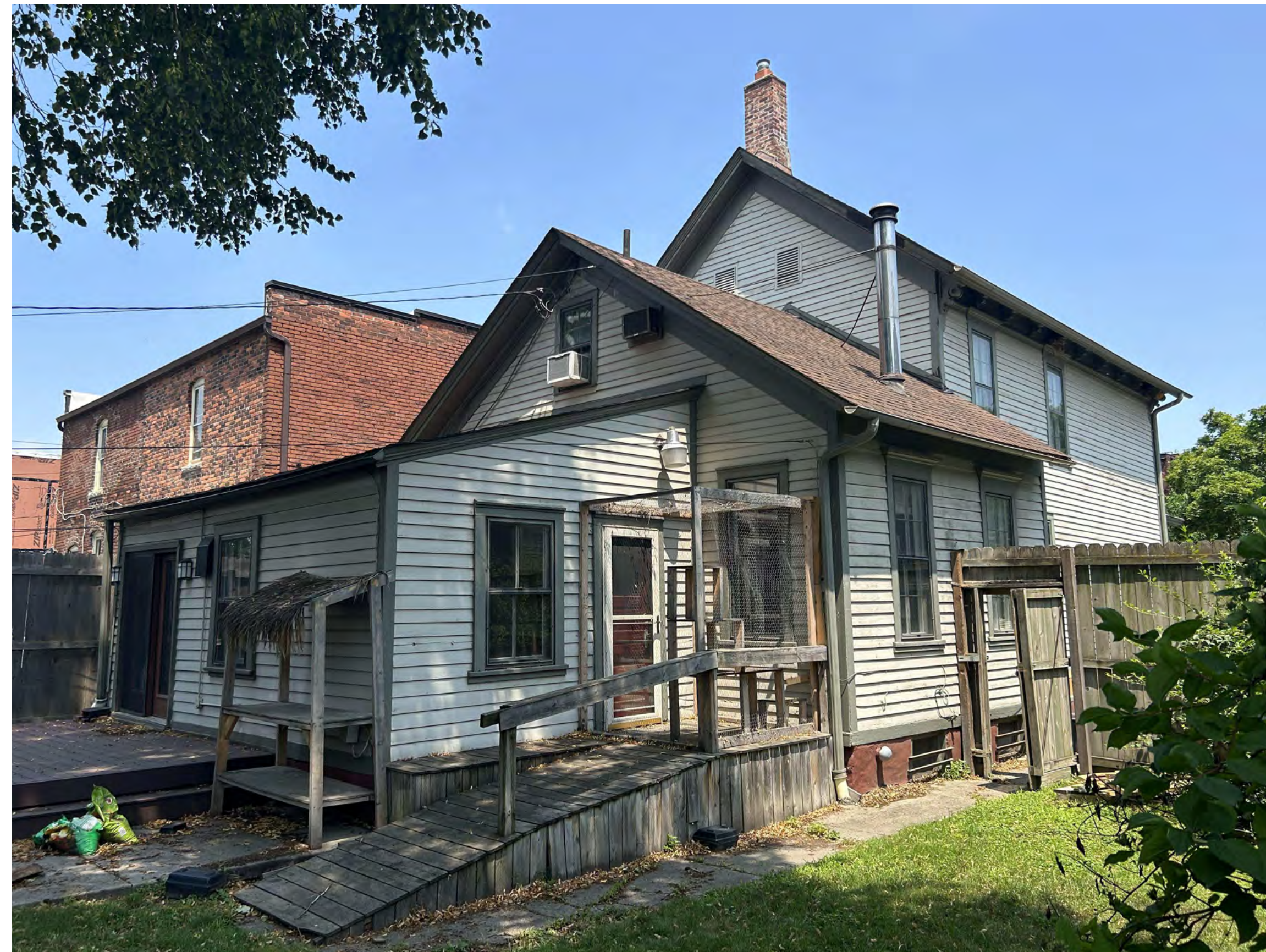
2. VIEW OF REAR LOOKING NORTHEAST (JULY 2023)
