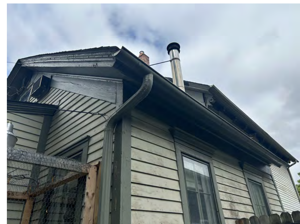
3. EXISTING CONDITION IMAGE OF GUTTER & DOWNSPOUT
