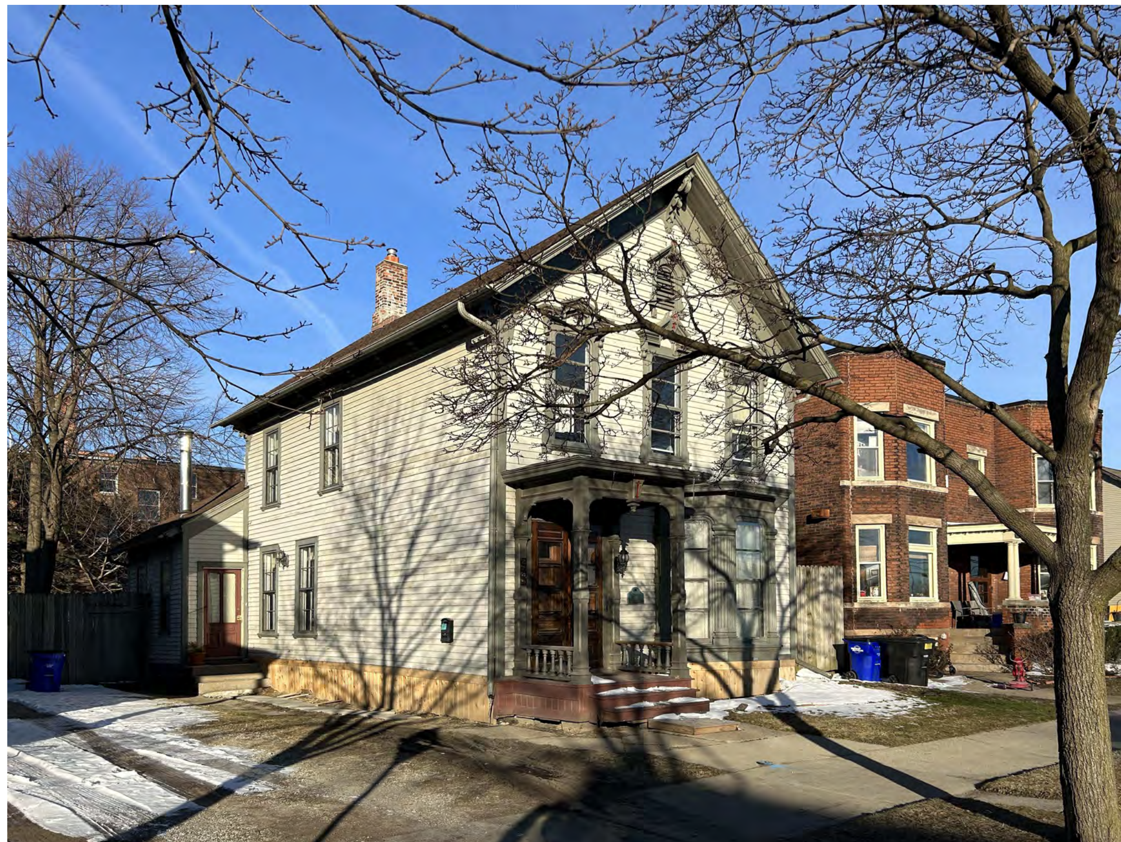
1. VIEW FROM STREET TOWARDS NORTHWEST (MARCH 2023)
