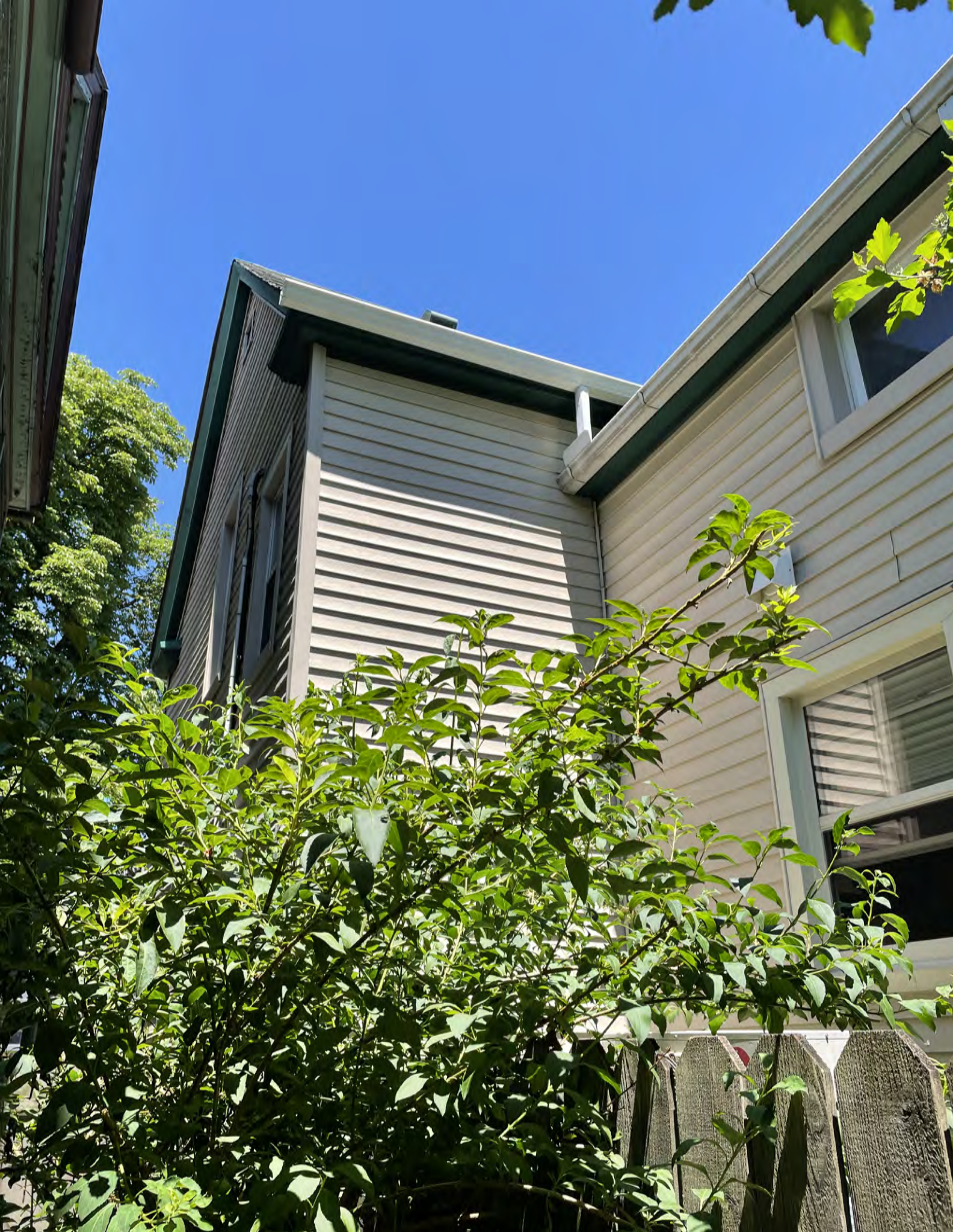
WEST FACADE VIEW FROM THE SOUTHWEST
