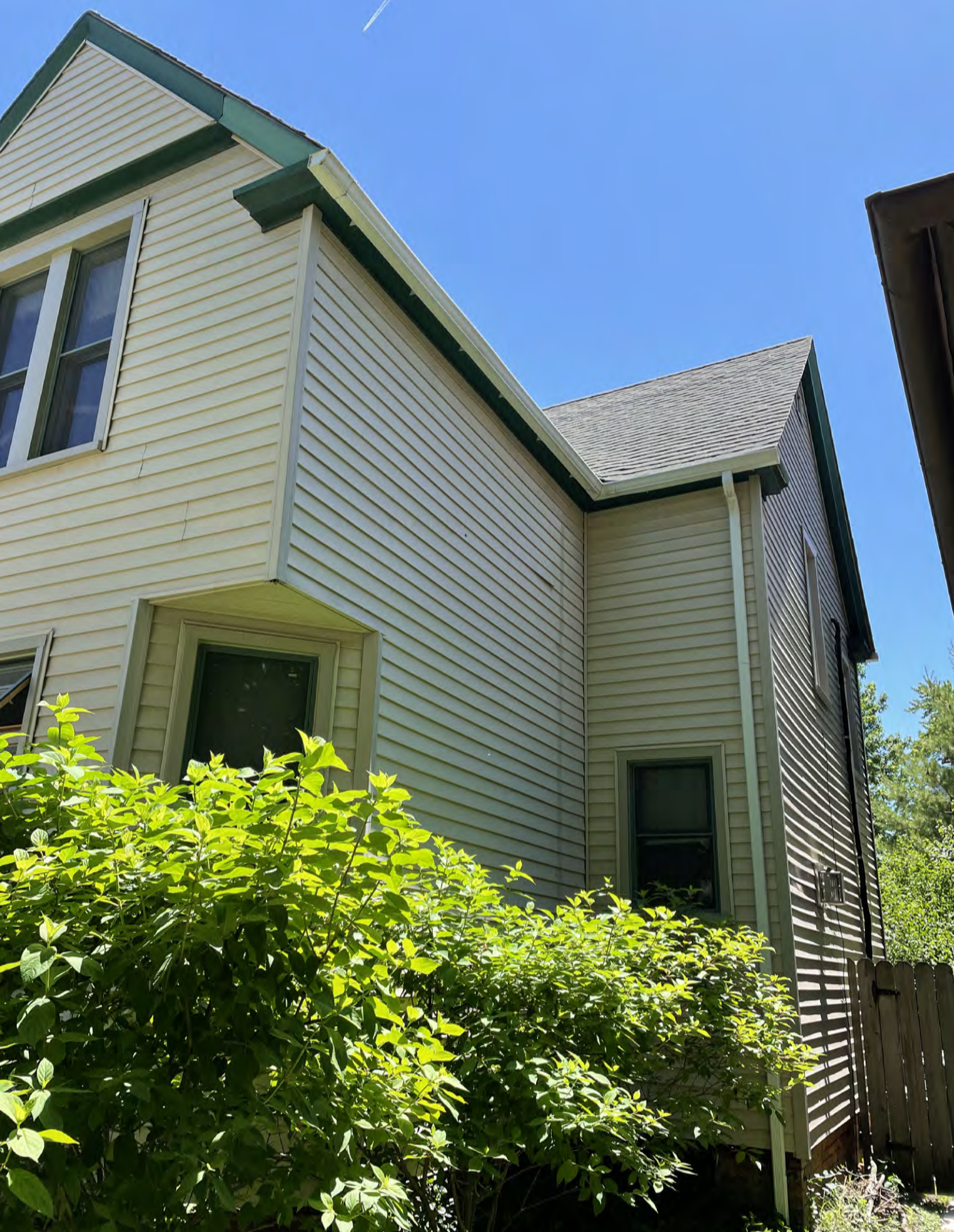
WEST FACADE VIEW FROM THE NORTHWEST
