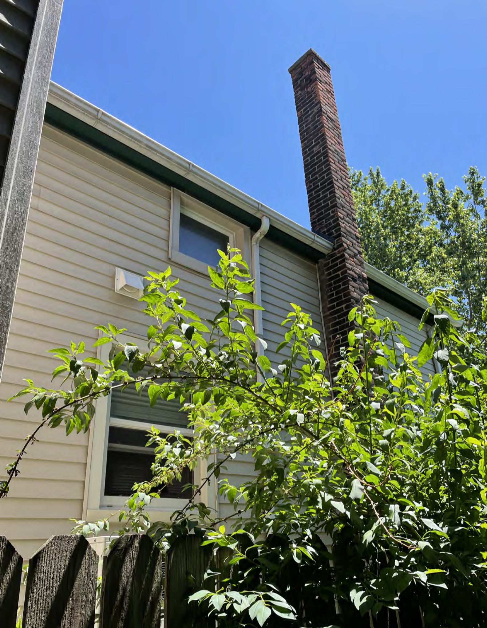
WEST FACADE TO THE SOUTH OF THE WEST GABLE
