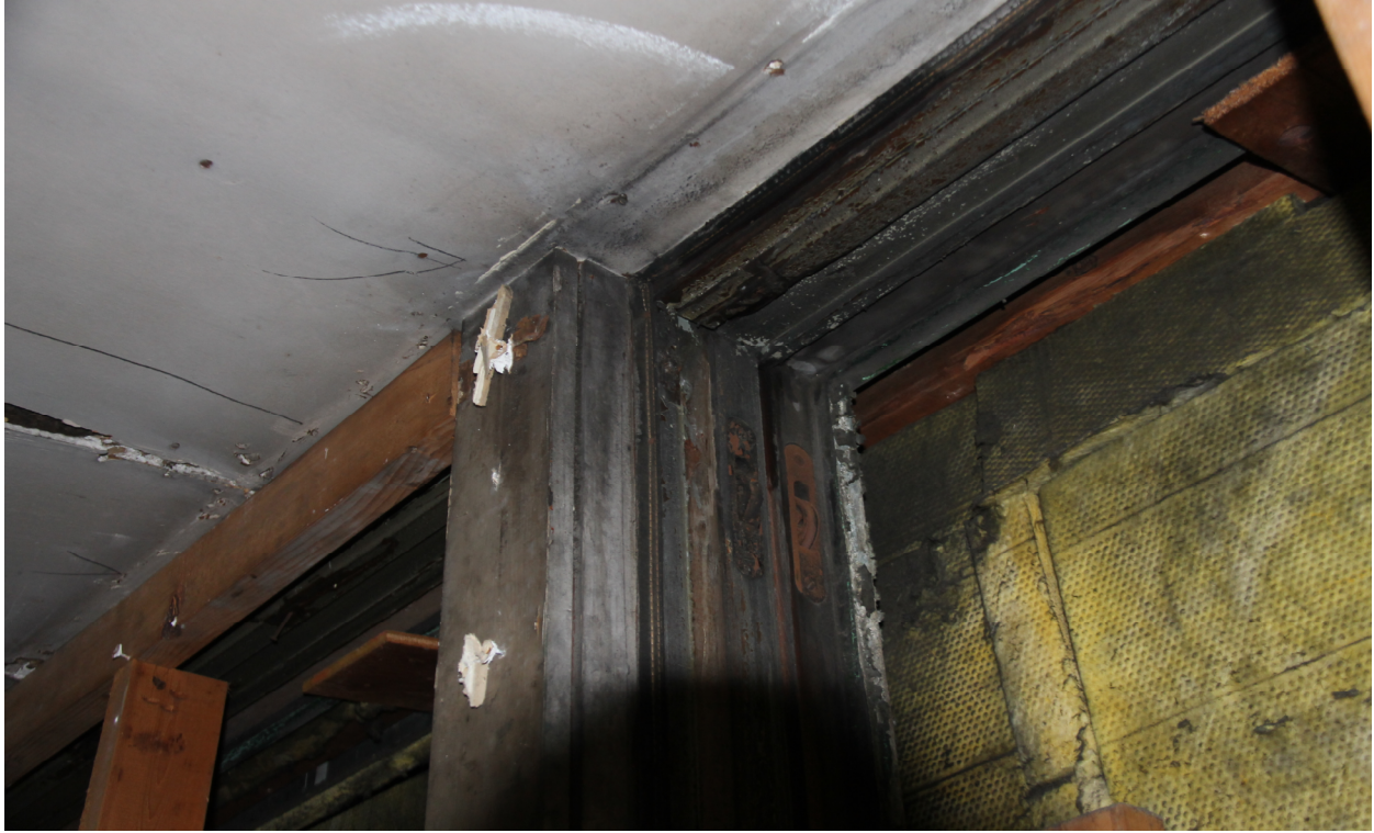
Interior 1332-1336 Broadway Center Building, 3 rd Floor
