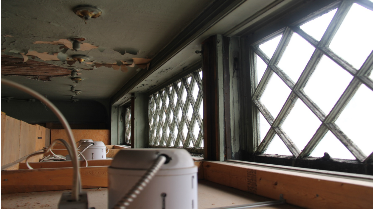
Interior 1332-1336 Broadway Center Building, 2 nd Floor
