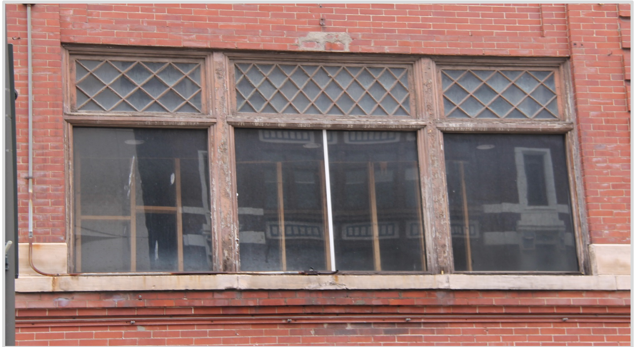
Window Front Façade 1332-1336 Broadway Center Building, 2 nd Floor
