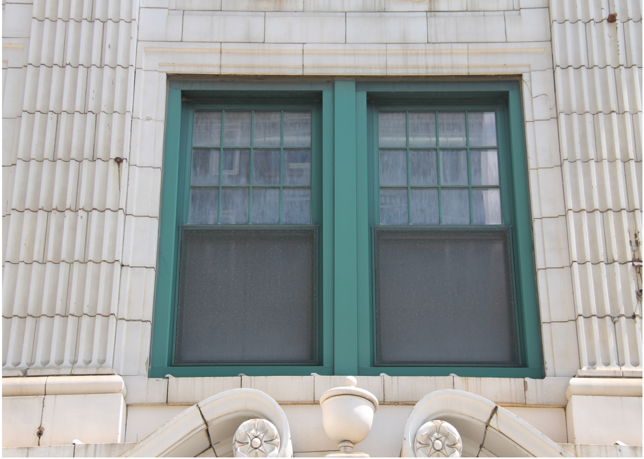
1332-1336 Broadway Right Building Windows
