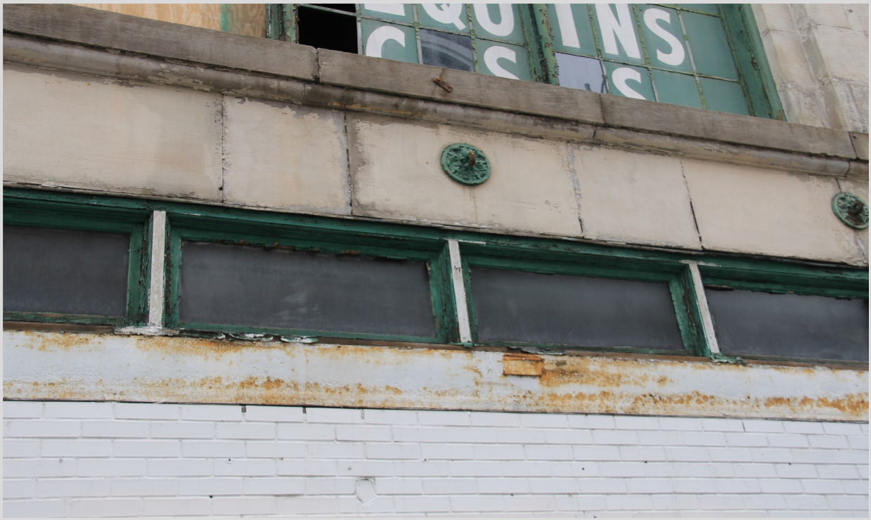
132 Broadway Wood Transoms Left Building
