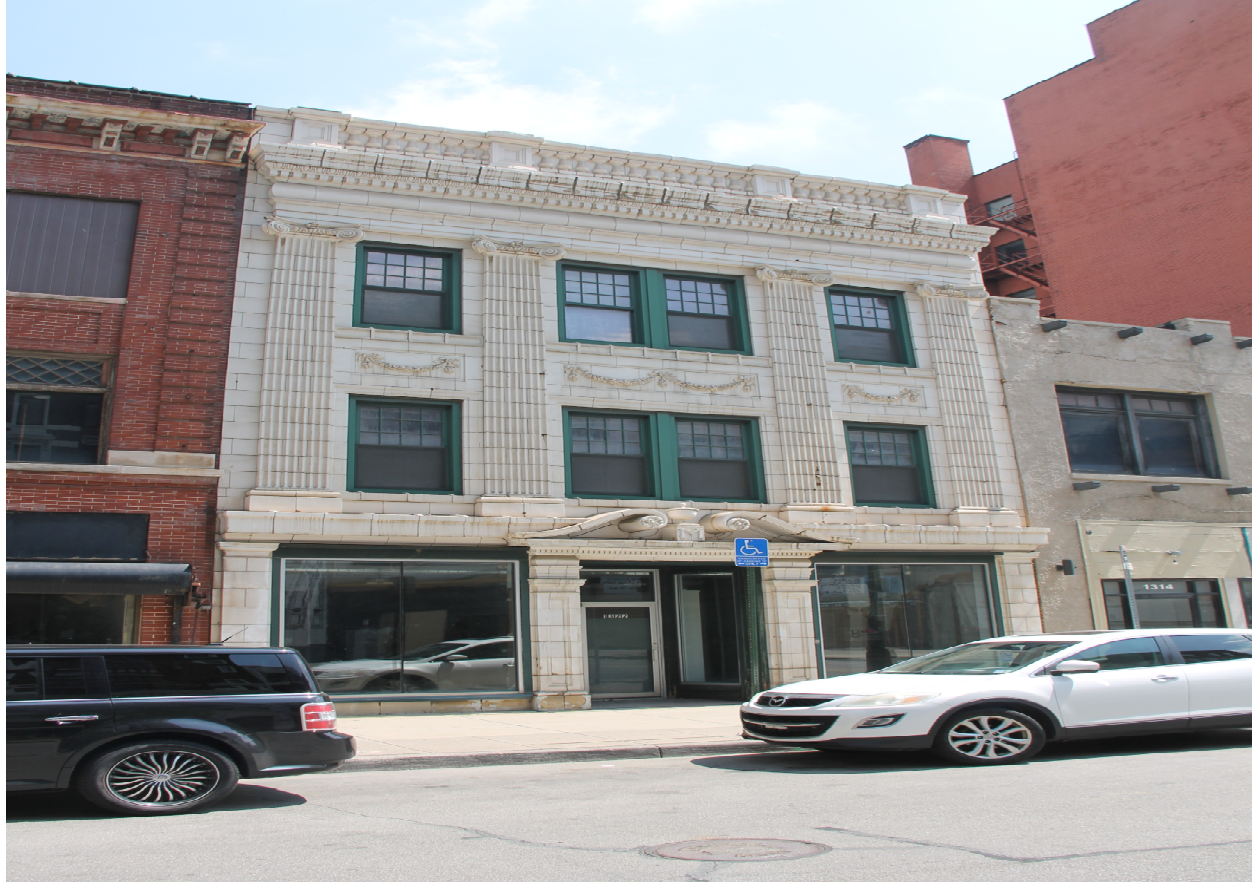
1332-1336 Broadway Right Building
