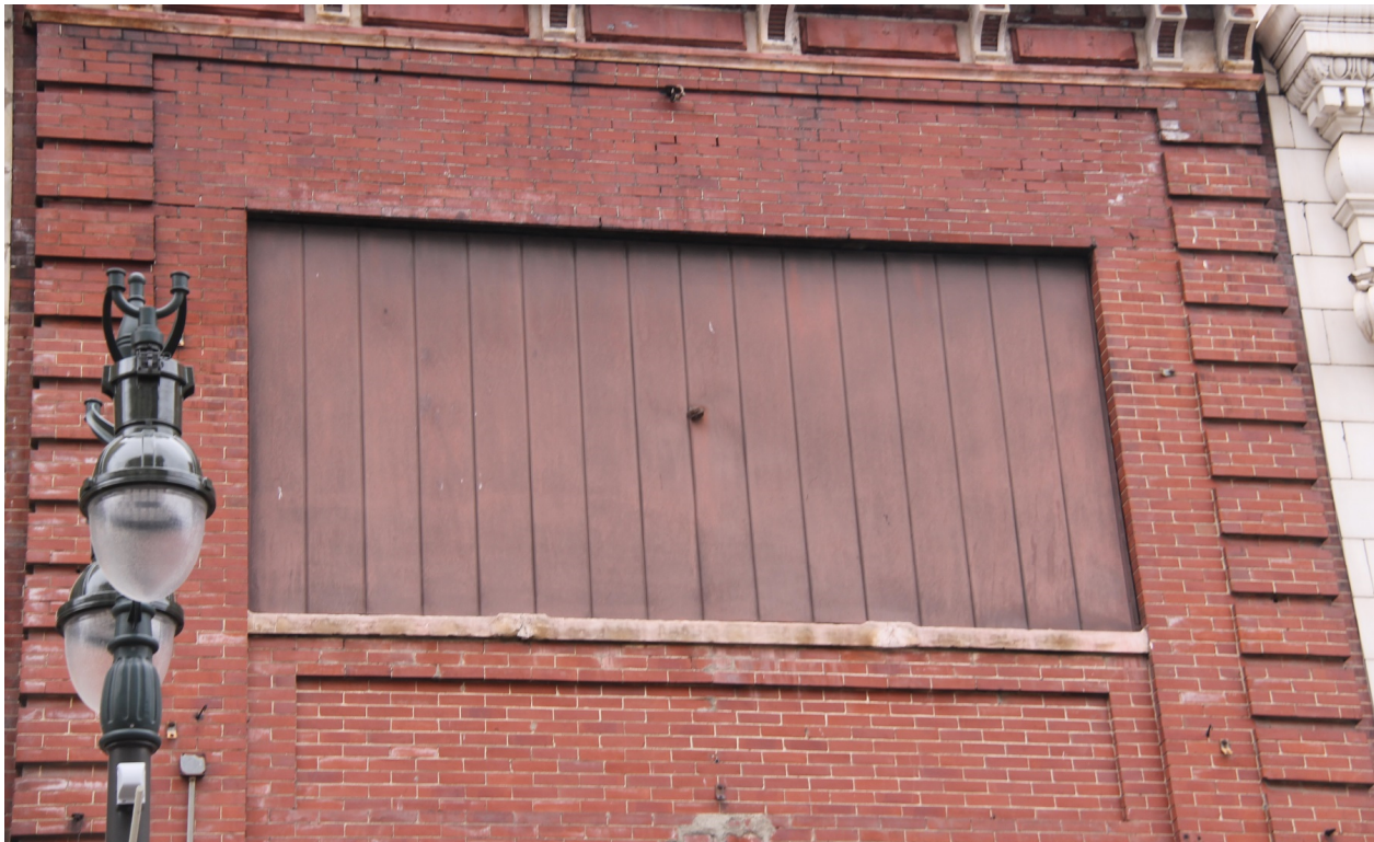
Window Front Façade 1332-1336 Broadway Center Building, 3 rd Floor
