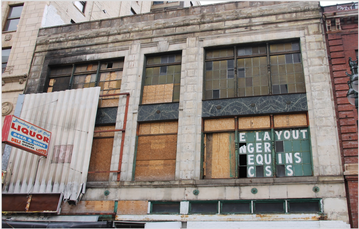
Windows on Front Façade of 1332 Broadway Left Building
