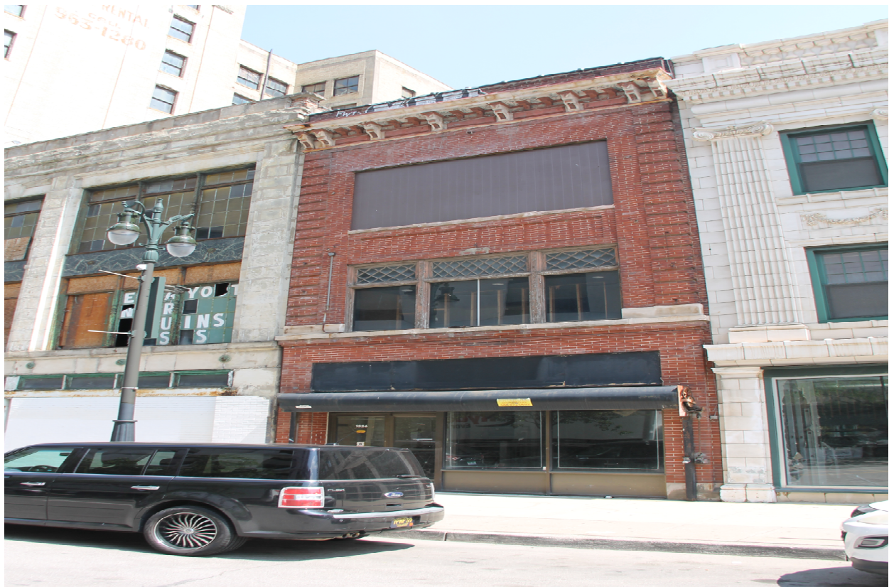
1332-1336 Broadway Center Building
