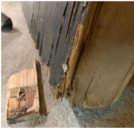
Images showing front door deterioration, and back porch entrance door
