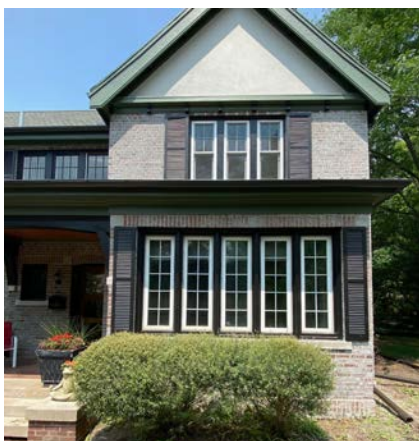
Current state of facade (showing restored brick moulding & gable)
