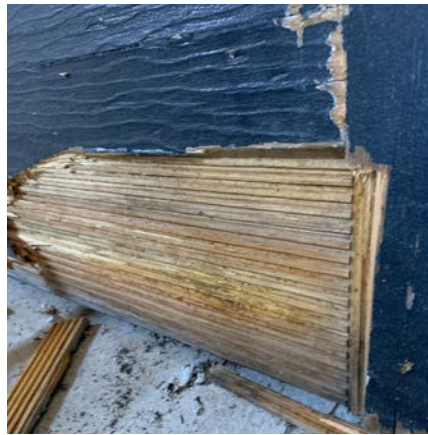
Images showing front door deterioration, and back porch entrance door
