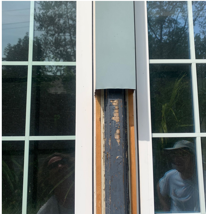
Aluminum capping covering all brick moulding and mullions. Existing picture window in place
