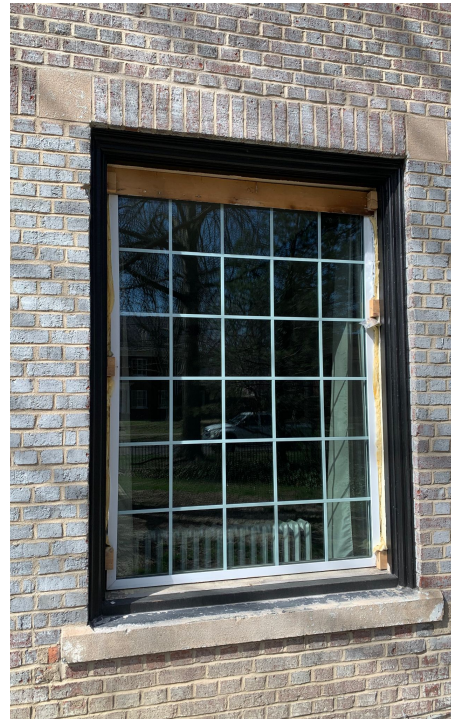
Aluminum capping covering all brick moulding and mullions. Existing picture window in place
