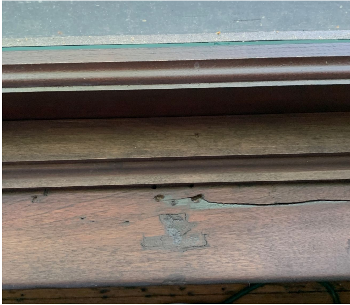
Original latch location centered on sill of picture window. Radiator in front of picture window
