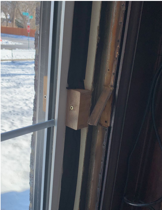
Original hinge and latch locations found at first floor casement openings (including picture windows-lower left image)
