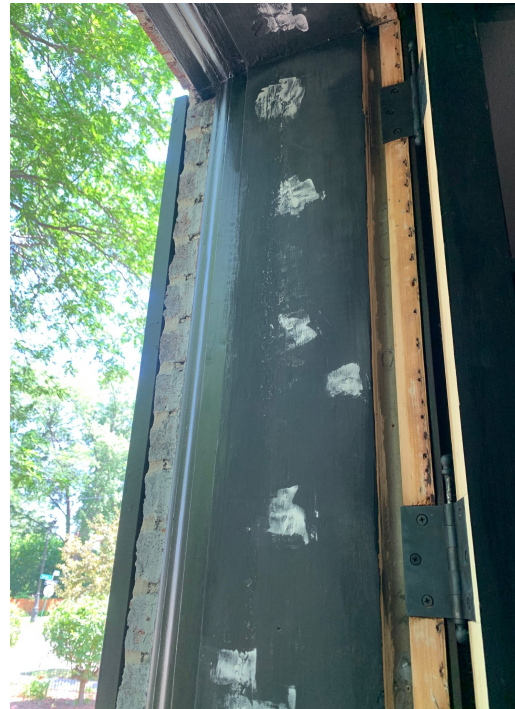
Original hinge and latch locations found at first floor casement openings (including picture windows-lower left image)
