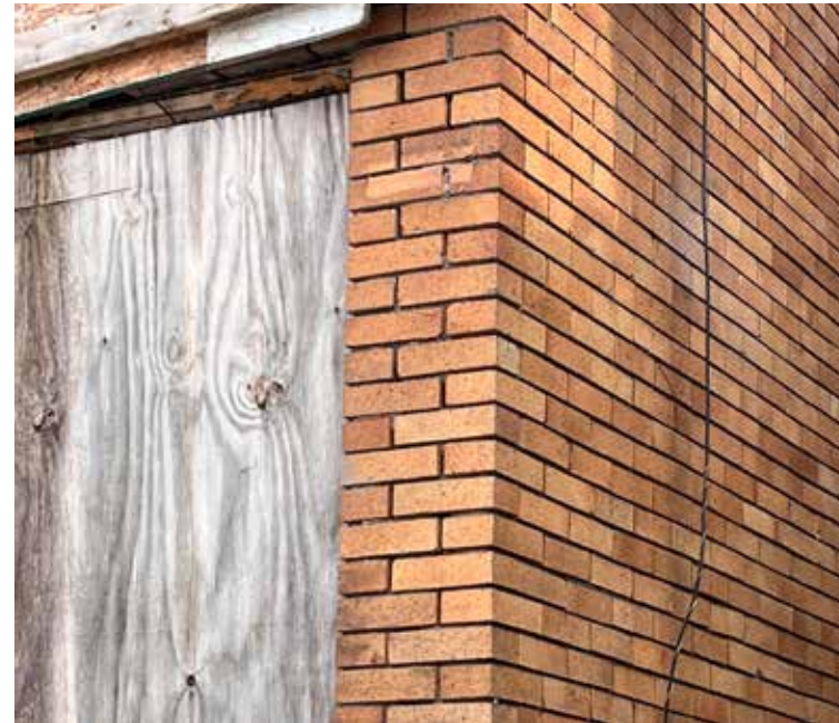
WEST FRONT PORCH ENTRY AT TRANSITION TO WEST FACADE
