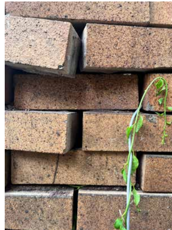
BRICK AT RIGHT FRONT SIDE DETAIL
