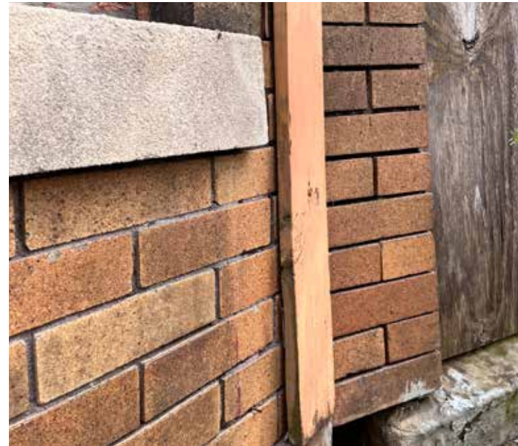
BRACING AT LOWER PORTION OF BAY
