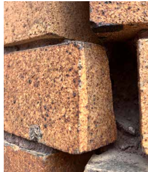
CLOSE UP OF BRICK AT CORNER BAY
