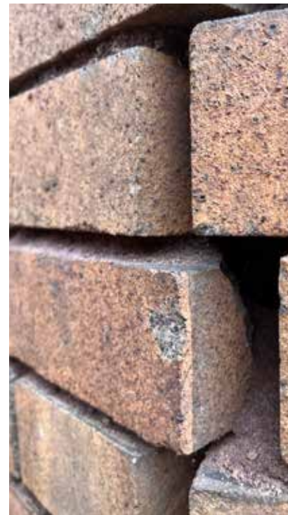
TYPICAL CONDITION AT BAY CORNERS
