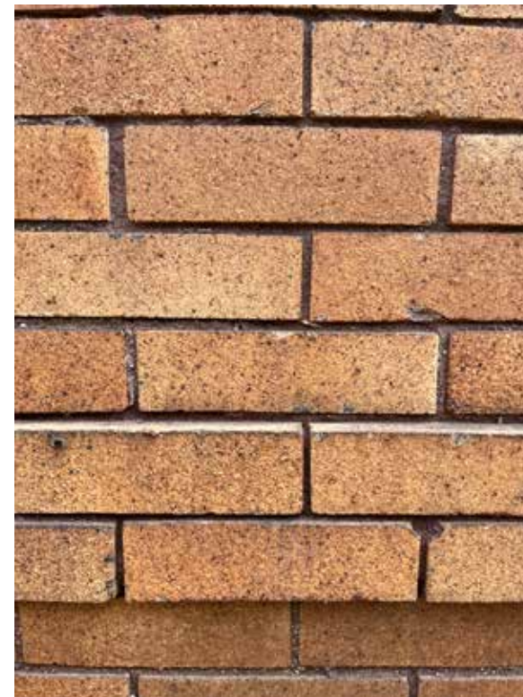
BRICK DETAIL AT MIDDLE FRONT BAY
