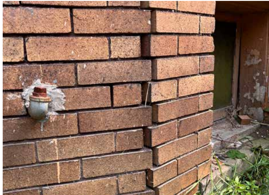
WEST FACE OF FRONT BAY AT GRADE
