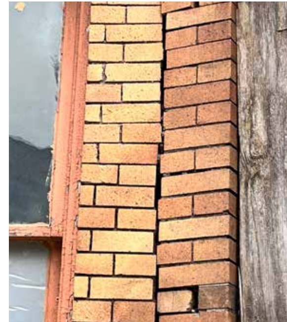
WEST FRONT PORCH ENTRY AT TRANSITION TO FRONT BAY
