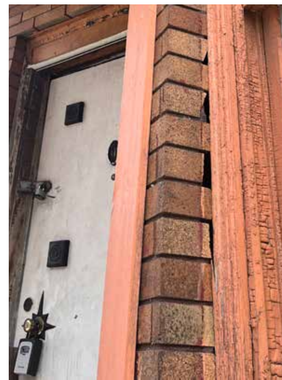
DETAIL OF EAST SIDE OF FRONT BAY AT FIRST LEVEL
