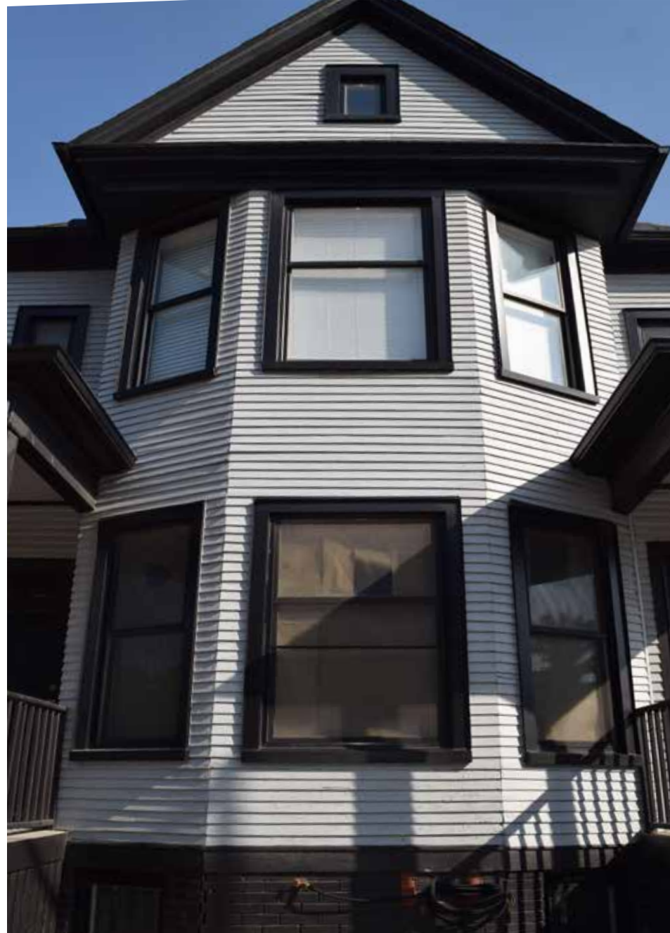
WINDOW CONDITION AT ADJACENT NEIGHBORING BUILDING WITH REPLACEMENT (NOT ORIGINAL) ALUMINUM-CLAD WINDOWS. BOTH BUILDINGS WERE BUILT IN 1907 AND ARE IDENTICAL IN DESIGN EXCEPT FOR THE CLADDING MATERIAL.
