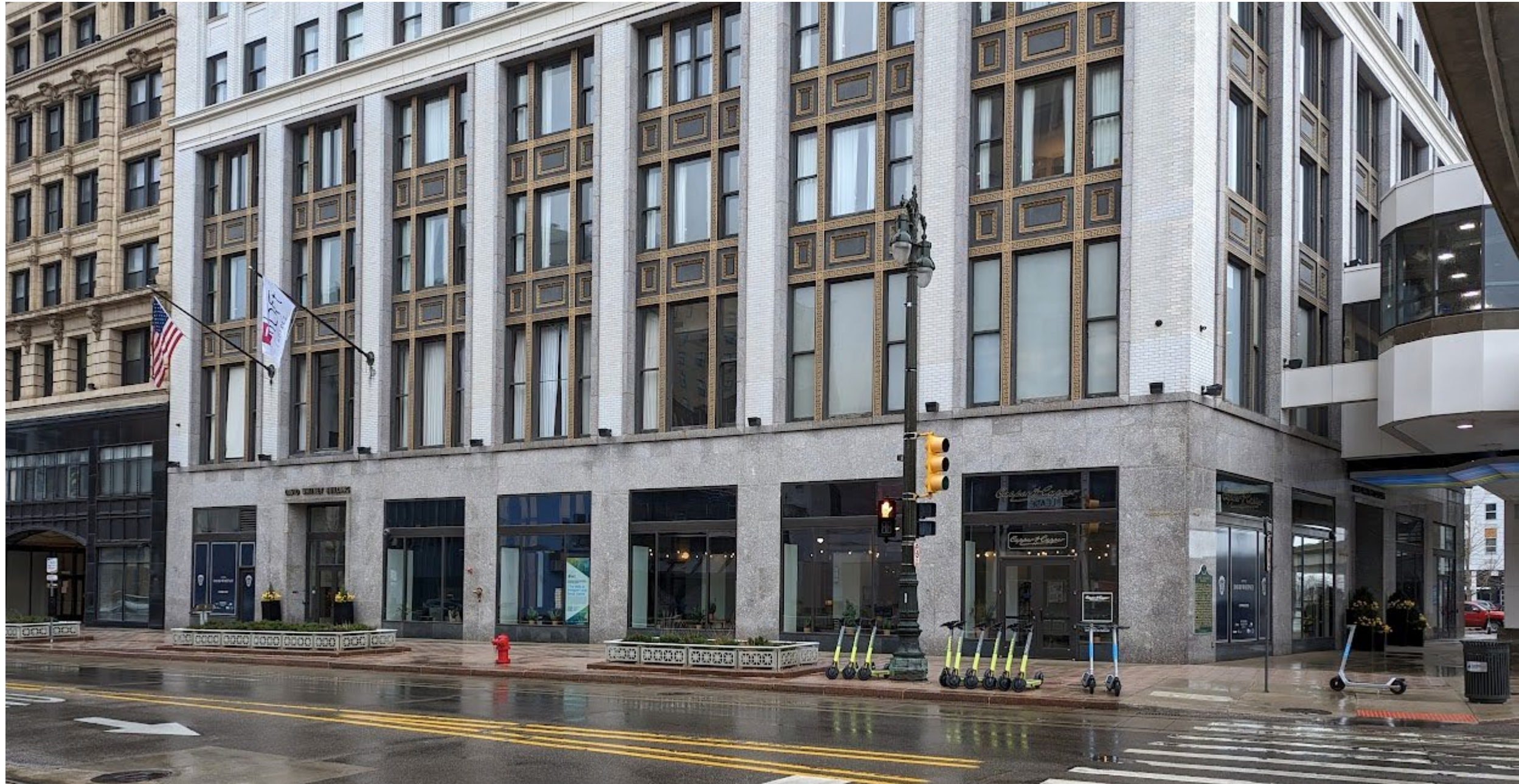
Northeast Corner of Building
