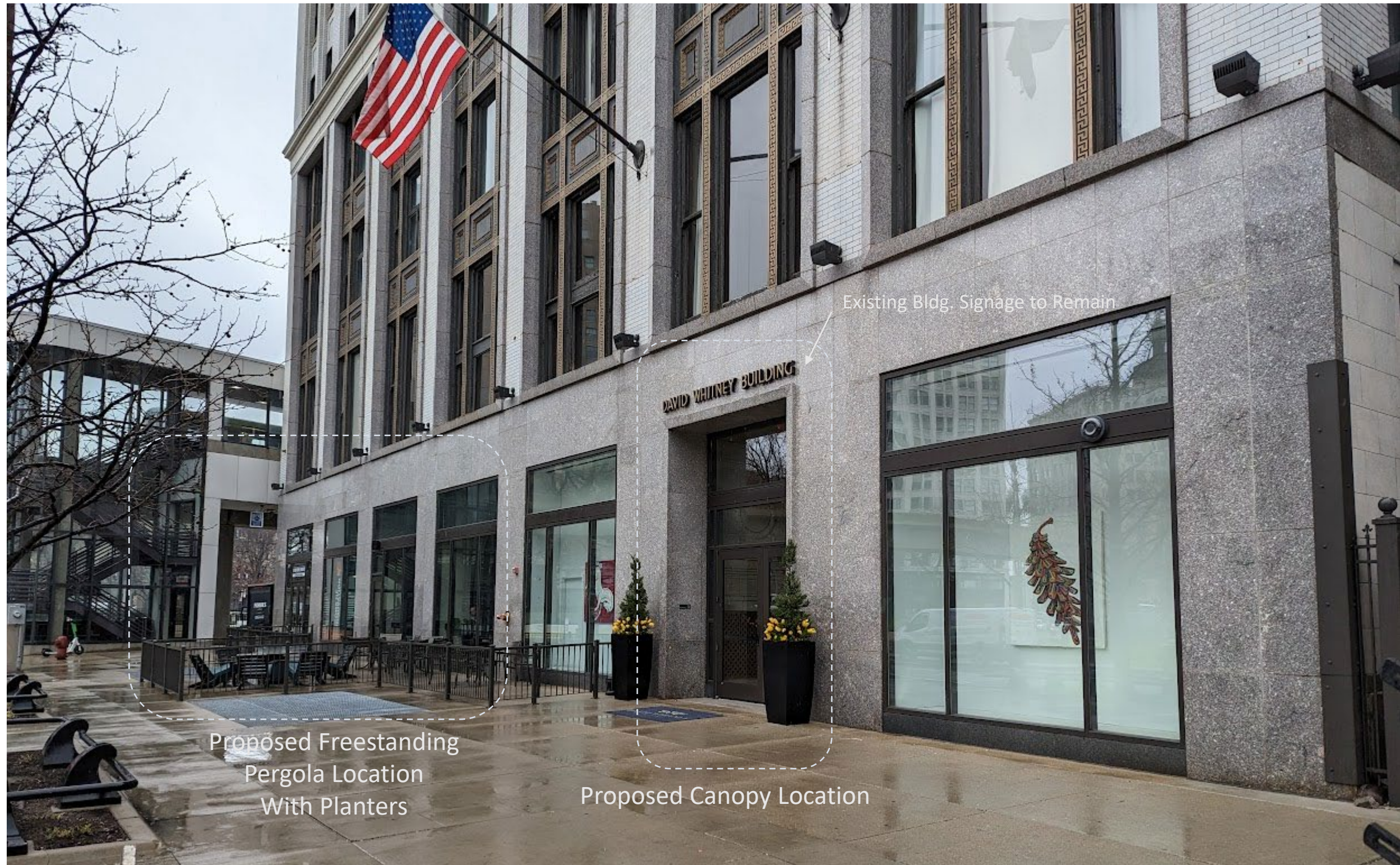
Southwest Corner – Looking North towards Grand Circus Park
