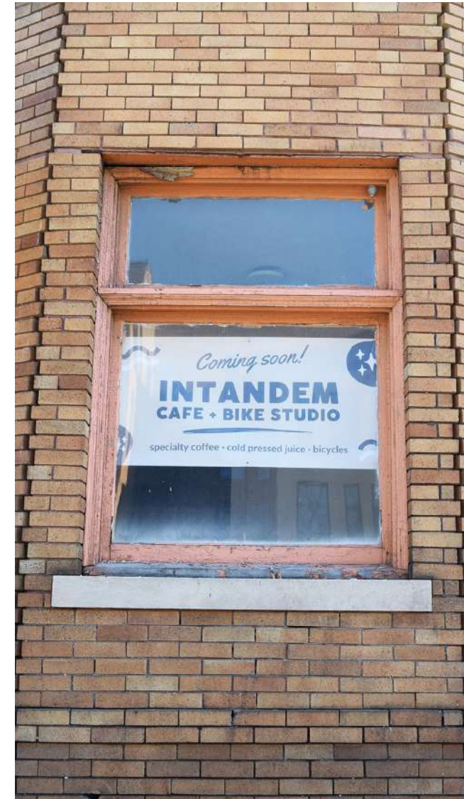
WINDOW 1.2 FIRST LEVEL FRONT MIDDLE BAY WINDOW, FIXED + FIXED TRANSOM
