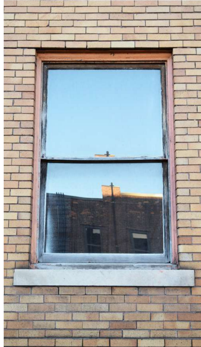
WINDOW 1.7 FIRST LEVEL, ALLEY SIDE DOUBLE-HUNG
