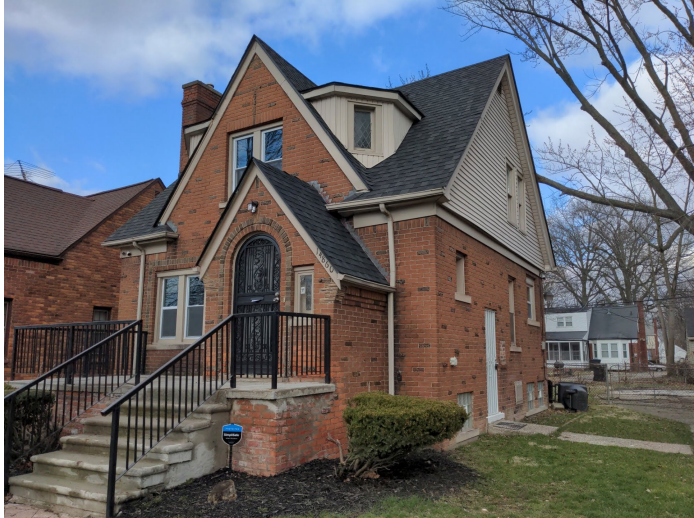
East view (1 window first floor)
