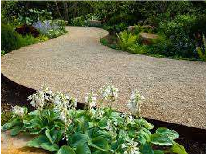
decomposed granite walking path with stabilizer
