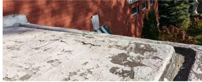
**MULTIPLE LAYERS OF DECAYED ROOFING, LEAKING INTEGRAL GUTTER, INADEQUATE GUTTER DEPTH, DECAYED WALL COUNTERFLASH**
