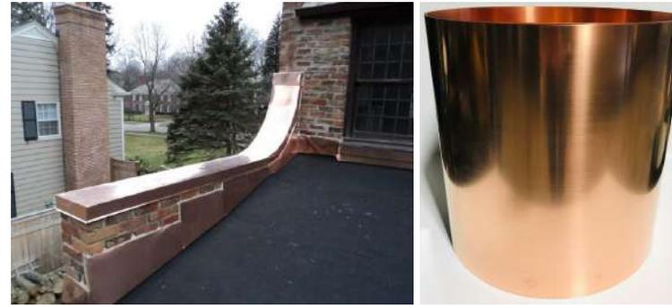
FLASHING AND COPING: TYPICAL 22 MIL COPPER FLASHING AND COPING MATERIAL
