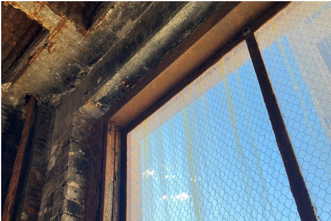
Window #19, 6 th Floor, South courtyard elevation, 04/03/23.
