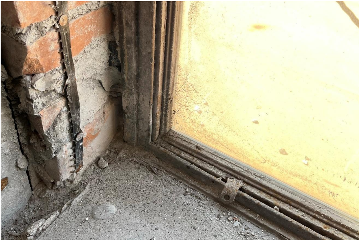
Window #35, Mezzanine, South elevation, 04/03/23.
