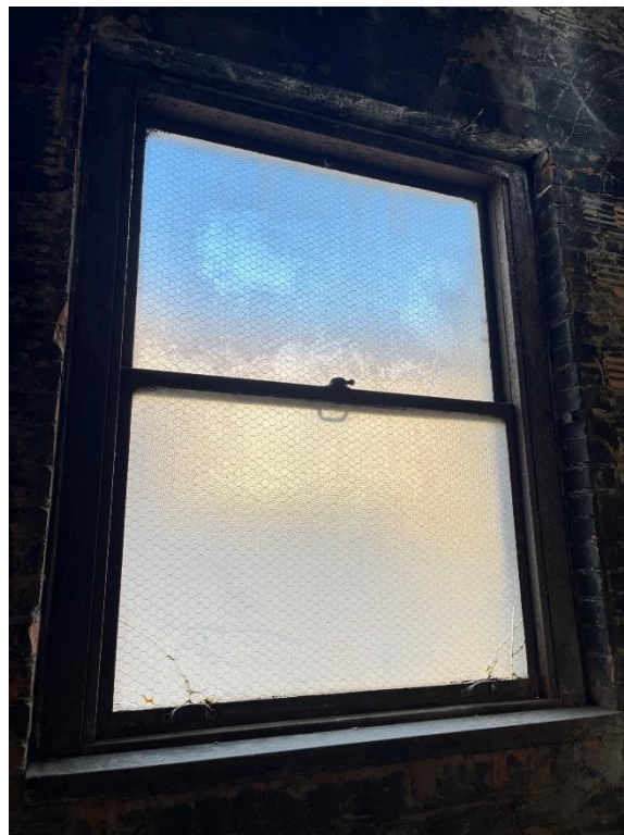
Window #26, 4 th Floor, West elevation, 04/03/23.
