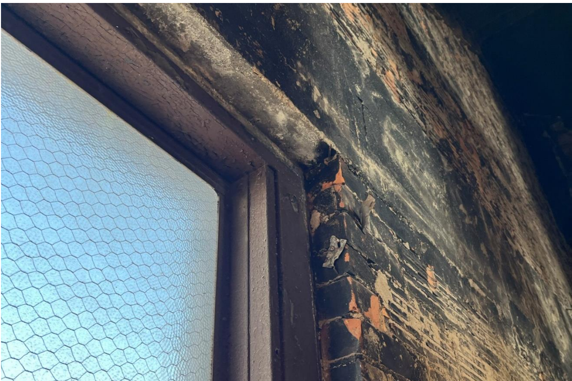
Window #17, 6 th Floor, West elevation, 04/03/23.
