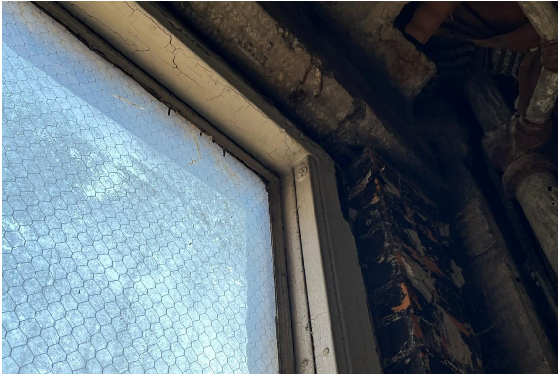
Window #31, 3 rd Floor, North elevation, 04/03/23.
