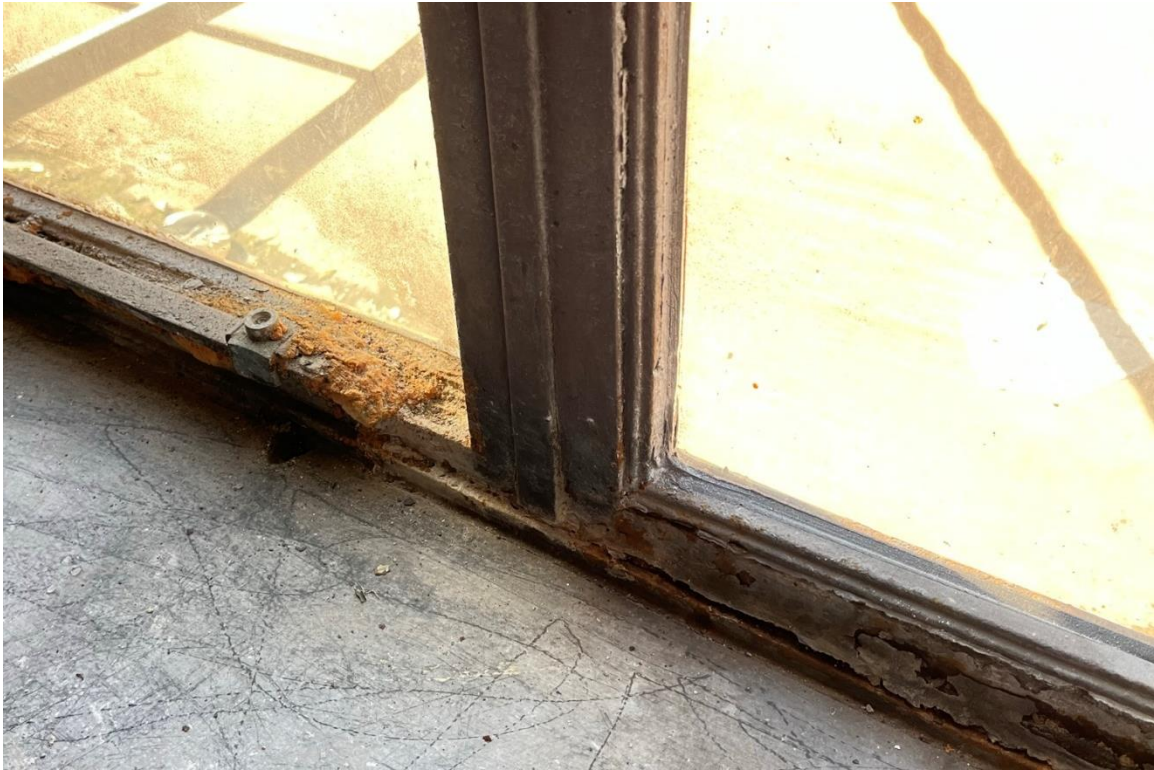
Window #34, Mezzanine, South elevation, 04/03/23.
