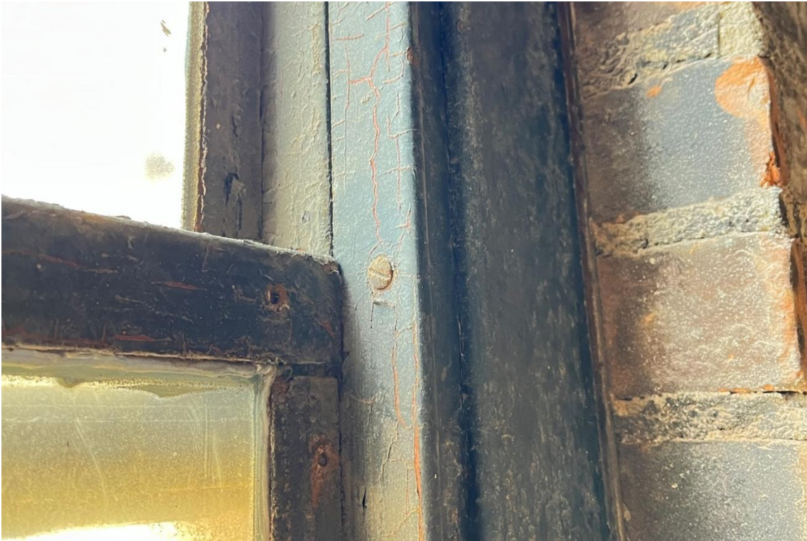
Window #29, 4 th Floor, North elevation, 04/03/23.
