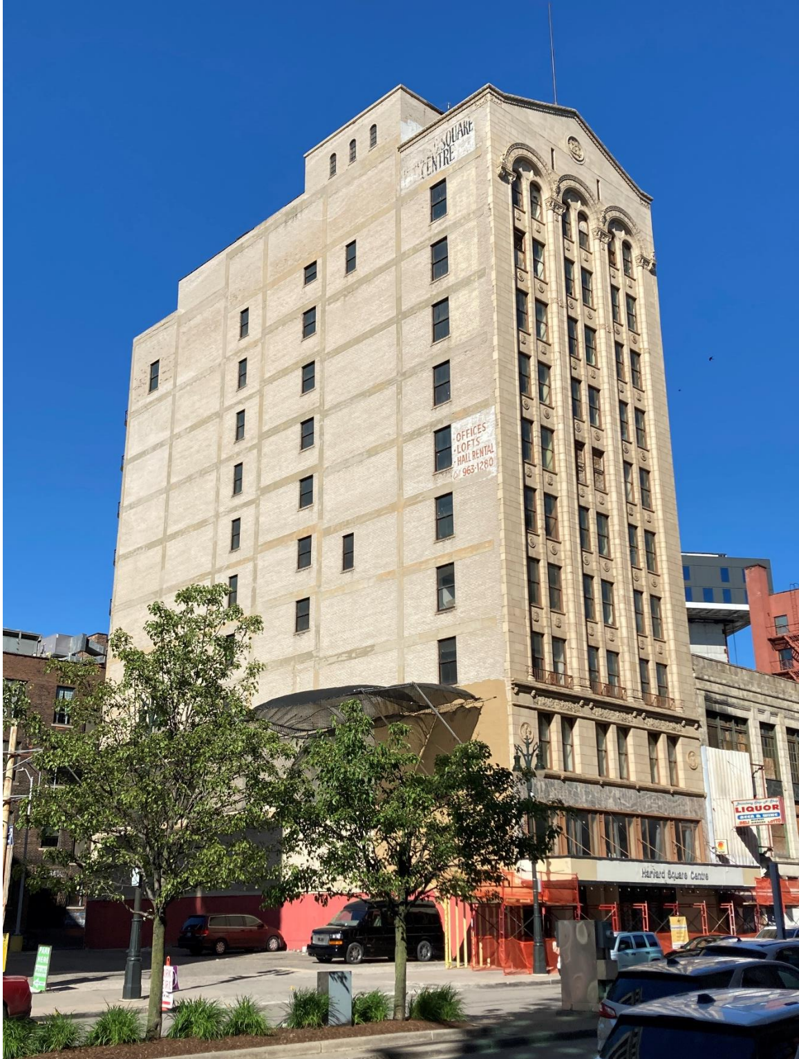
South elevation (facing Broadway) and west elevation, Looking northeast. 06/23/22.
