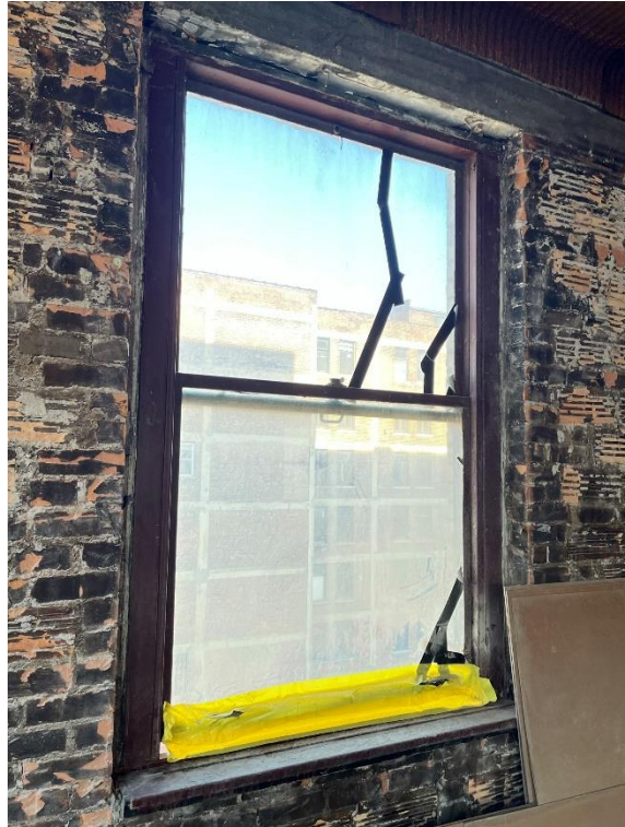
Window #21, 5 th Floor, West elevation, 04/03/23.
