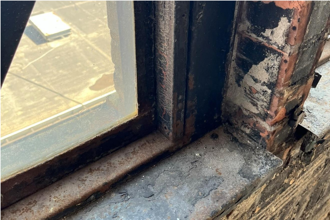
Window #20, 6 th Floor, North elevation, 04/03/23.
