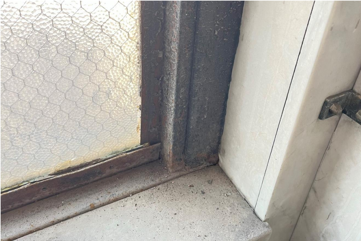
Window #4, 10 th Floor, West elevation, 04/03/23.
