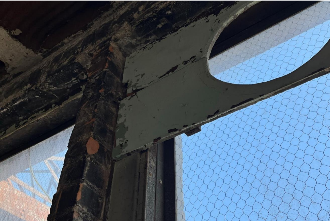
Window #16, 7 th Floor, North elevation, 04/03/23.
