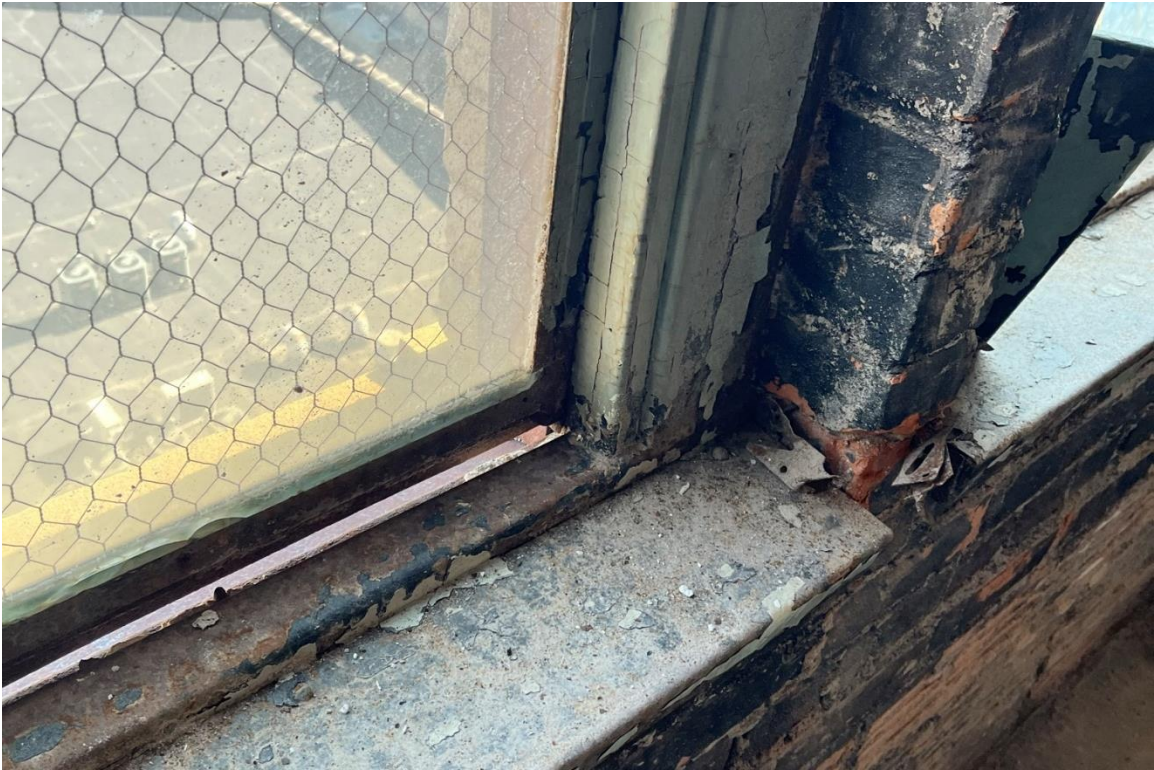
Window #8, 9 th Floor, North elevation, 04/03/23.
