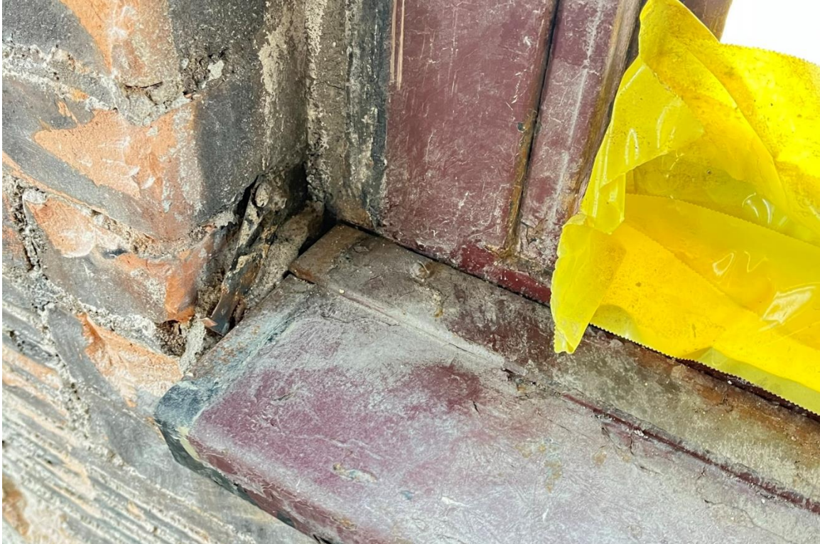
Window #21, 5 th Floor, West elevation, 04/03/23.
