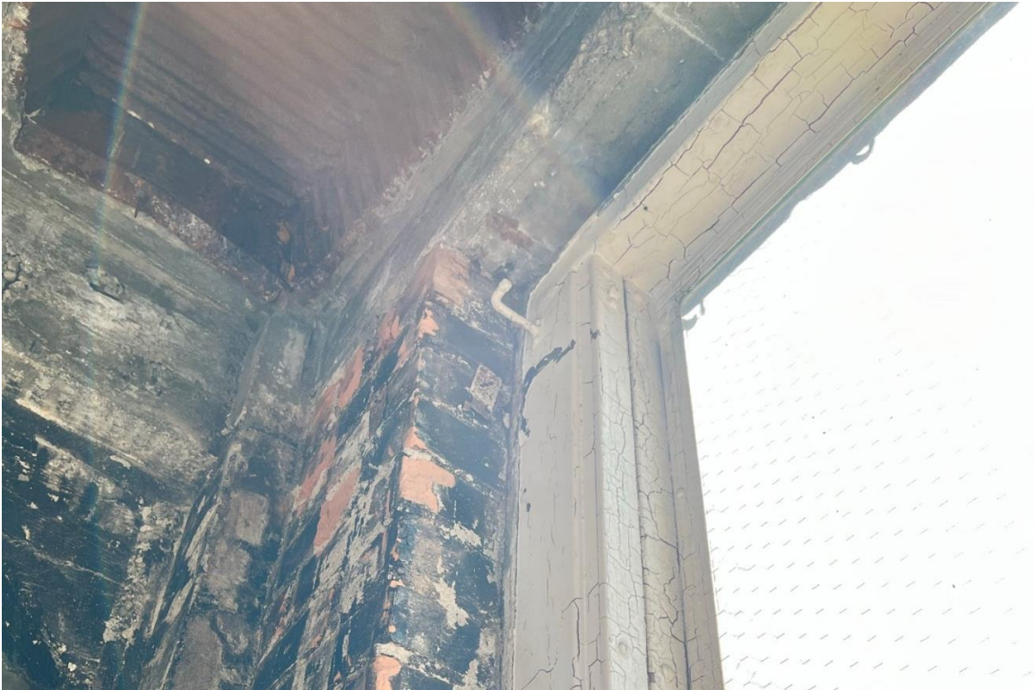
Window #30, 3 rd Floor, East elevation, 04/03/23.
