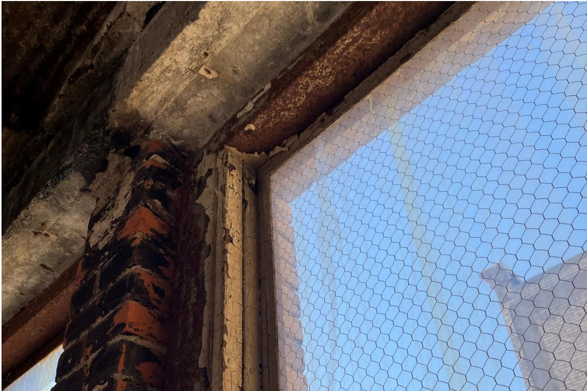
Window #7, 9 th Floor, South courtyard elevation, 04/03/23.
