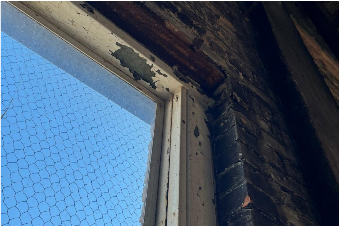
Window #3, 10 th Floor, North elevation, 04/03/23.
