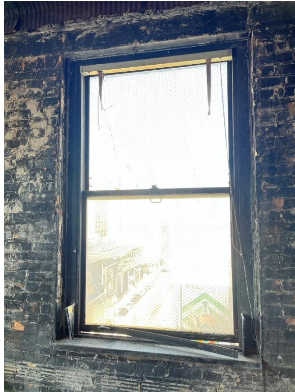
Window #9, 8 th Floor, West elevation, 04/03/23.
