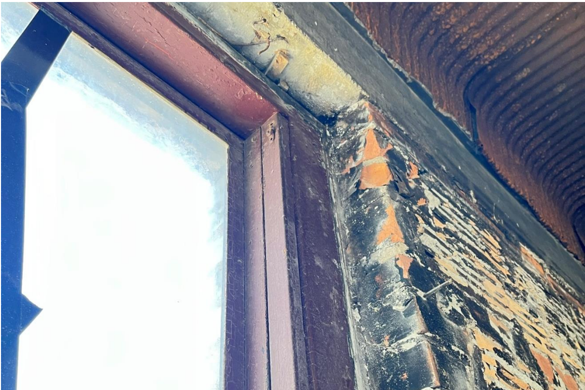
Window #21, 5 th Floor, West elevation, 04/03/23.
