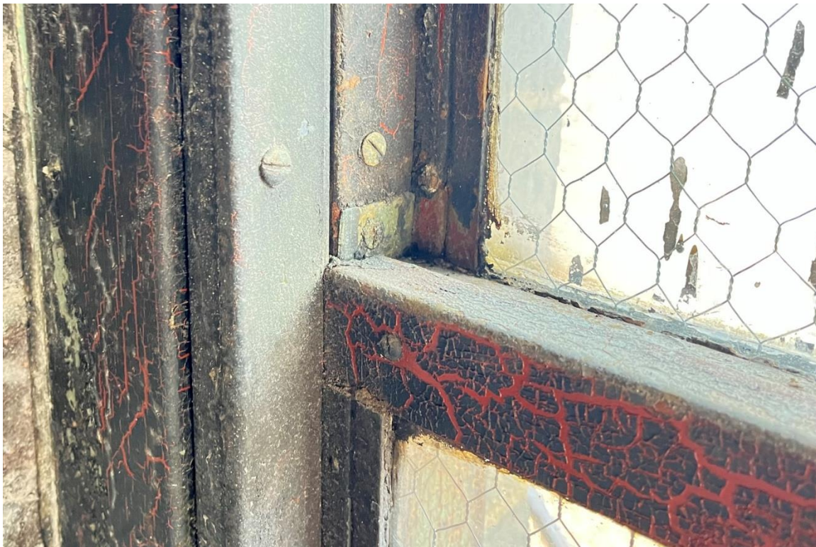
Window #28, 4 th Floor, North elevation, 04/03/23.
