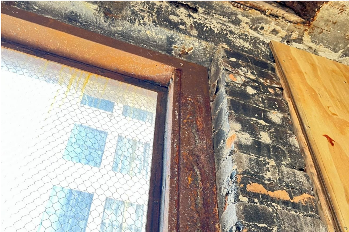
Window #19, 6 th Floor, South courtyard elevation, 04/03/23.
