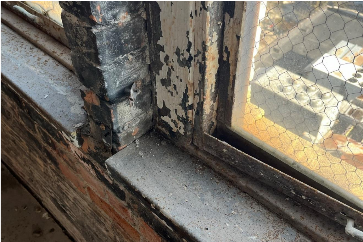
Window #3, 10 th Floor, North elevation, 04/03/23.
