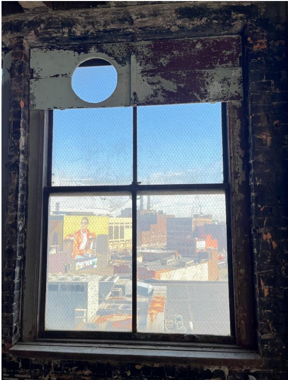
Window #16, 7 th Floor, North elevation, 04/03/23.
