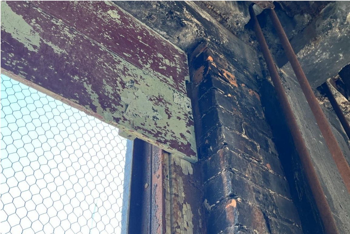
Window #16, 7 th Floor, North elevation, 04/03/23.
