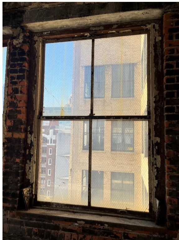
Window #7, 9 th Floor, South courtyard elevation, 04/03/23.
