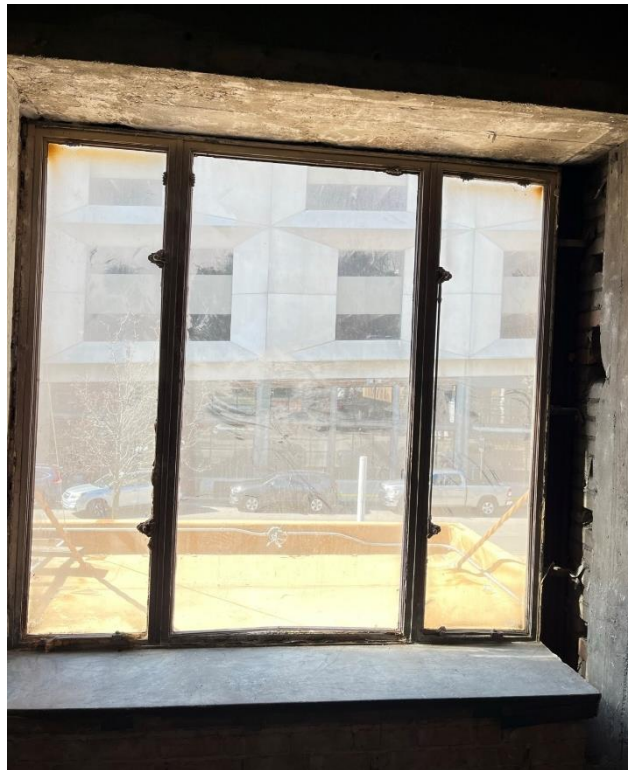
Window #34, Mezzanine, South elevation, 04/03/23.
