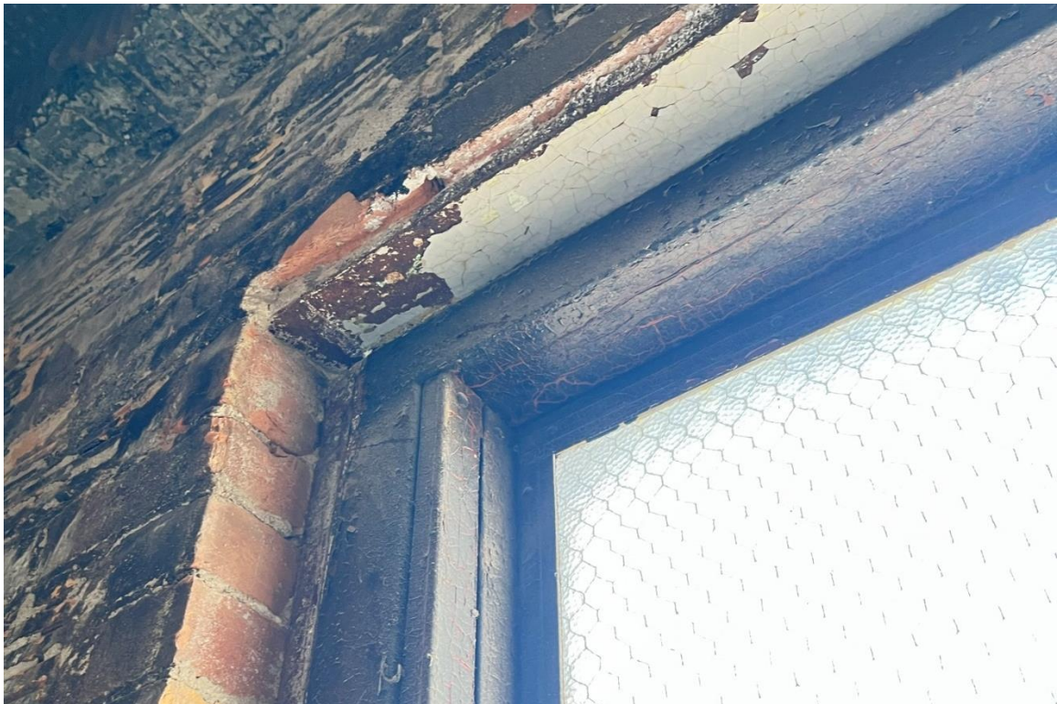
Window #4, 10 th Floor, West elevation, 04/03/23.
