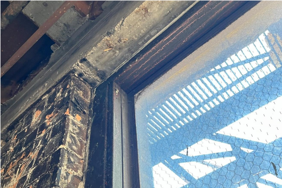
Window #28, 4 th Floor, North elevation, 04/03/23.
