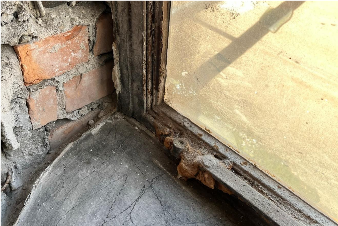
Window #34, Mezzanine, South elevation, 04/03/23.
