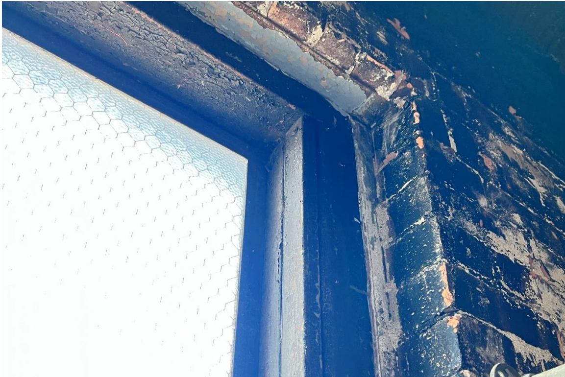
Window #13, 8 th Floor, West elevation, 04/03/23.
