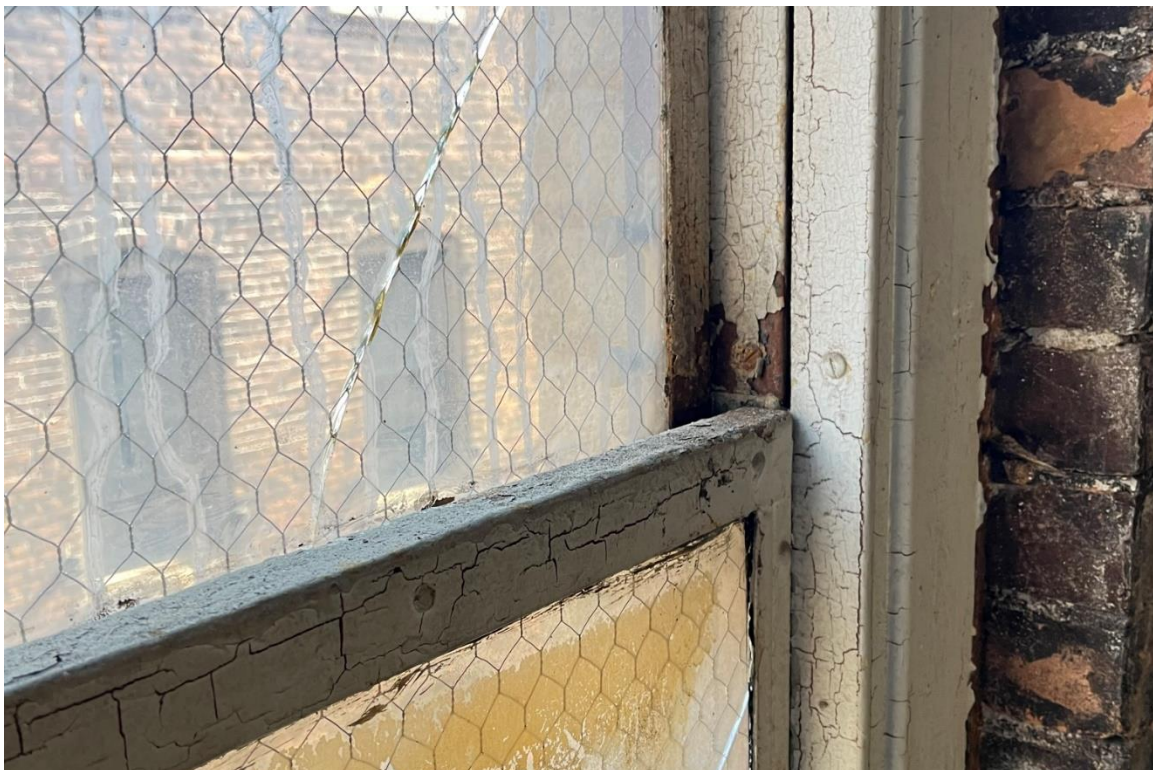
Window #31, 3 rd Floor, North elevation, 04/03/23.
