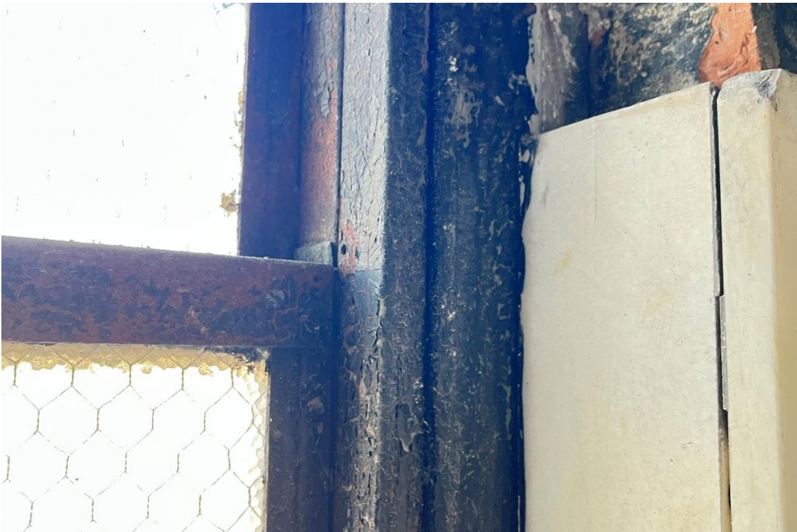
Window #13, 8 th Floor, West elevation, 04/03/23.
