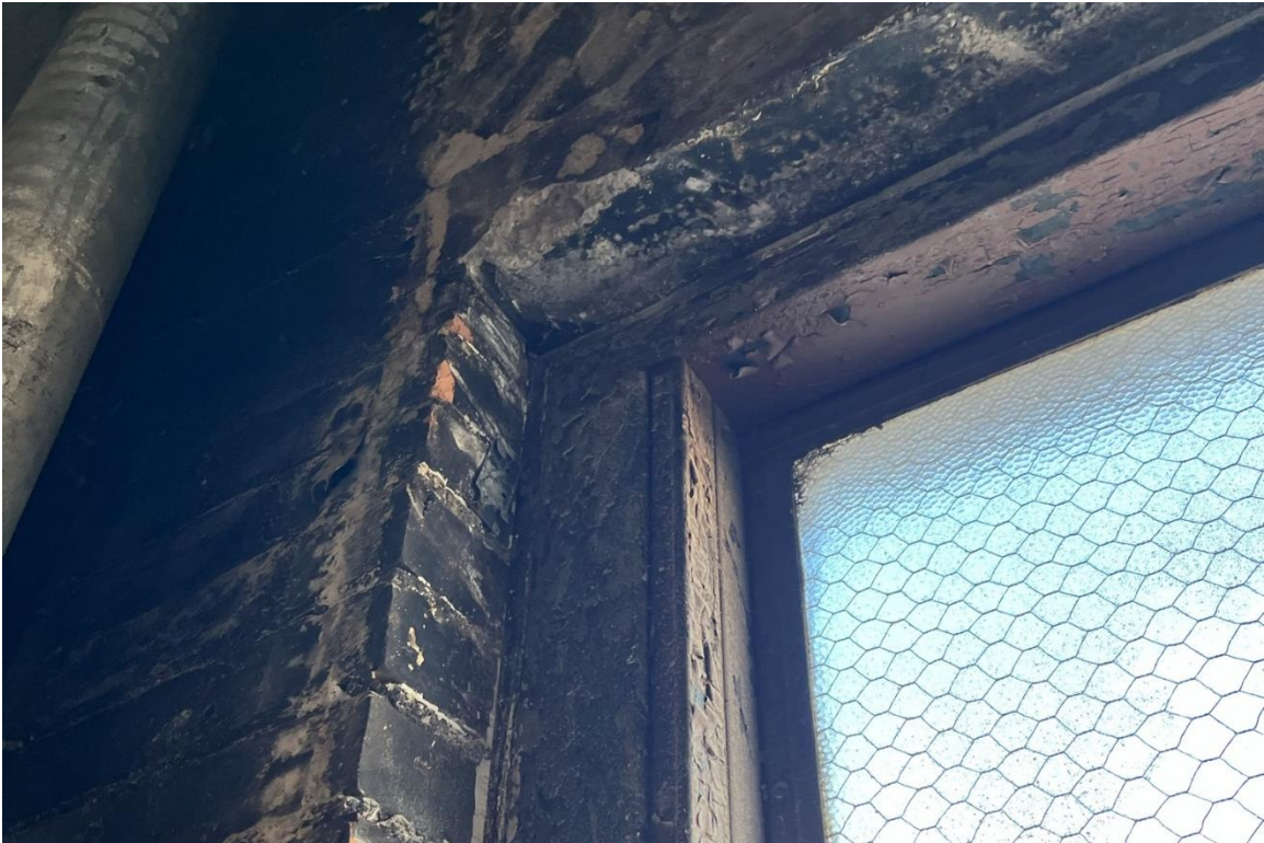
Window #26, 4 th Floor, West elevation, 04/03/23.
