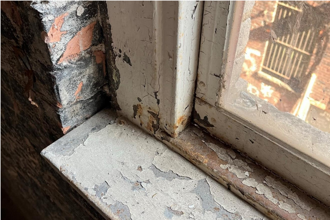
Window #33, 2 nd Floor, North elevation, 04/03/23.
