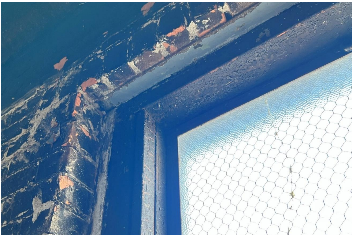
Window #13, 8 th Floor, West elevation, 04/03/23.
