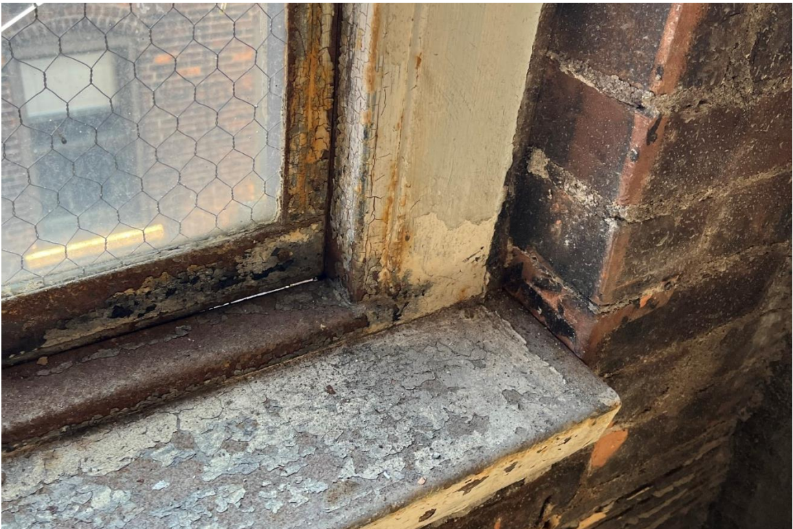
Window #25, 5 th Floor, North elevation, 04/03/23.
