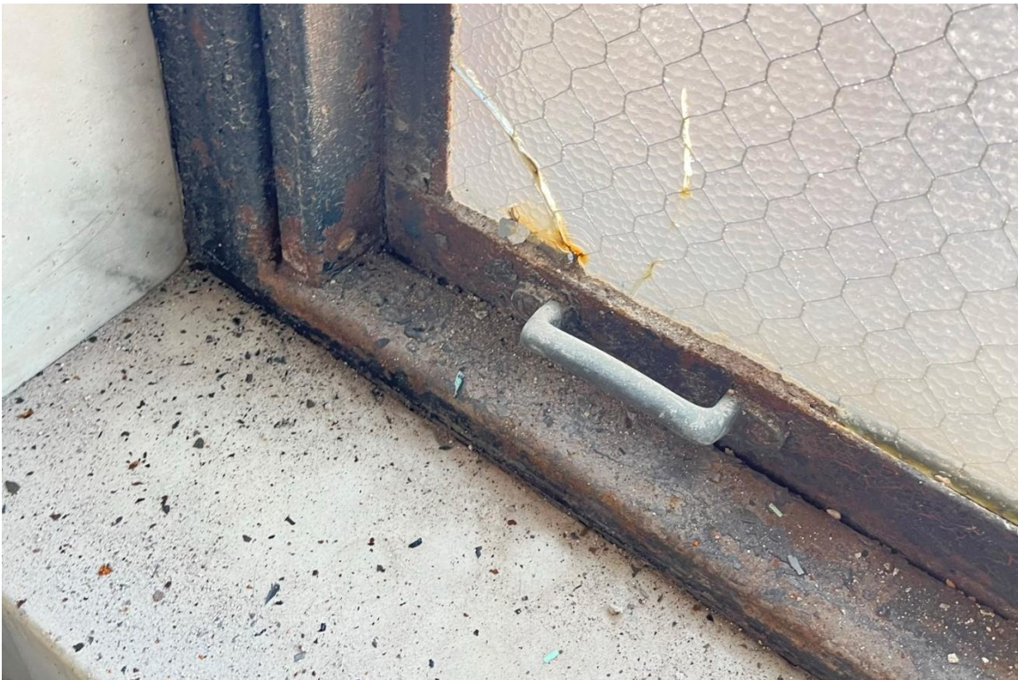
Window #13, 8 th Floor, West elevation, 04/03/23.
