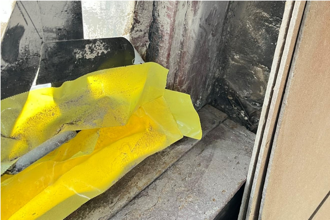
Window #21, 5 th Floor, West elevation, 04/03/23.
