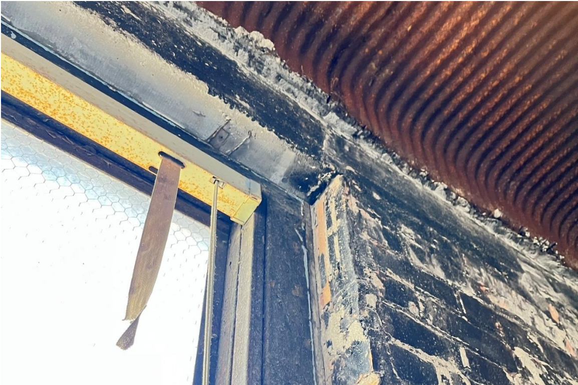
Window #9, 8 th Floor, West elevation, 04/03/23.
