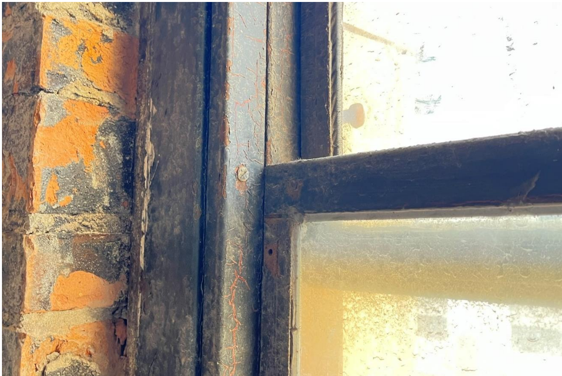
Window #29, 4 th Floor, North elevation, 04/03/23.
