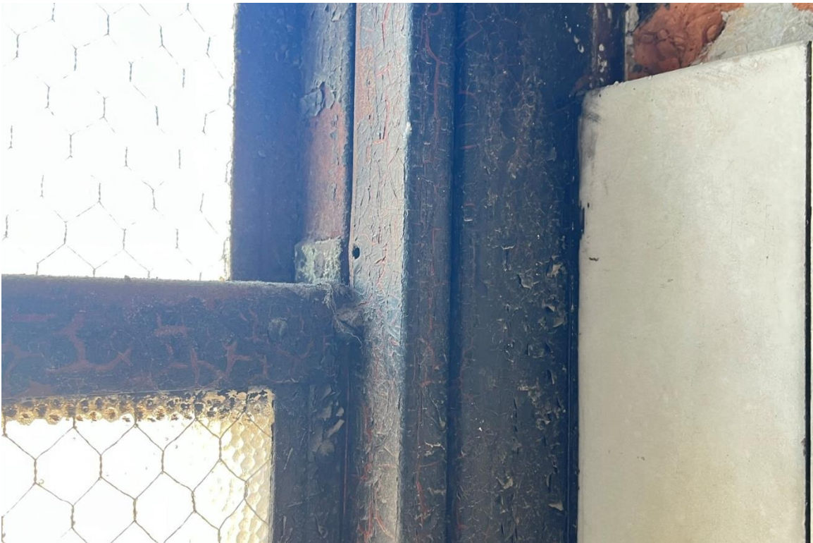
Window #4, 10 th Floor, West elevation, 04/03/23.
