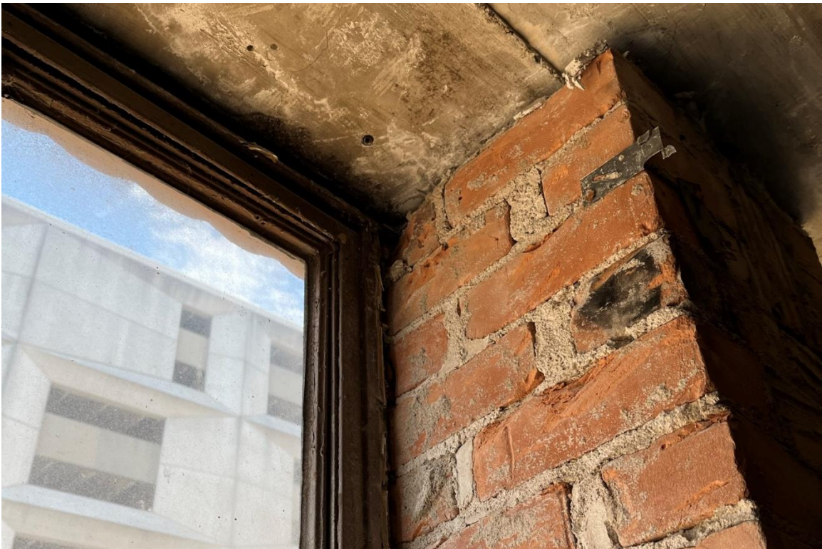
Window #35, Mezzanine, South elevation, 04/03/23.
