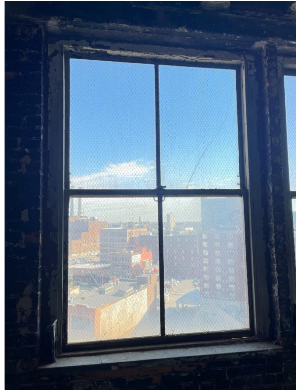
Window #8, 9 th Floor, North elevation, 04/03/23.
