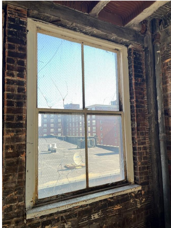
Window #25, 5 th Floor, North elevation, 04/03/23.
