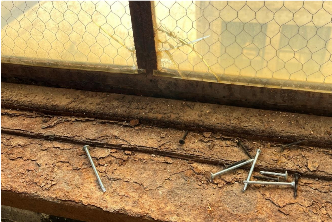
Window #19, 6 th Floor, South courtyard elevation, 04/03/23.
