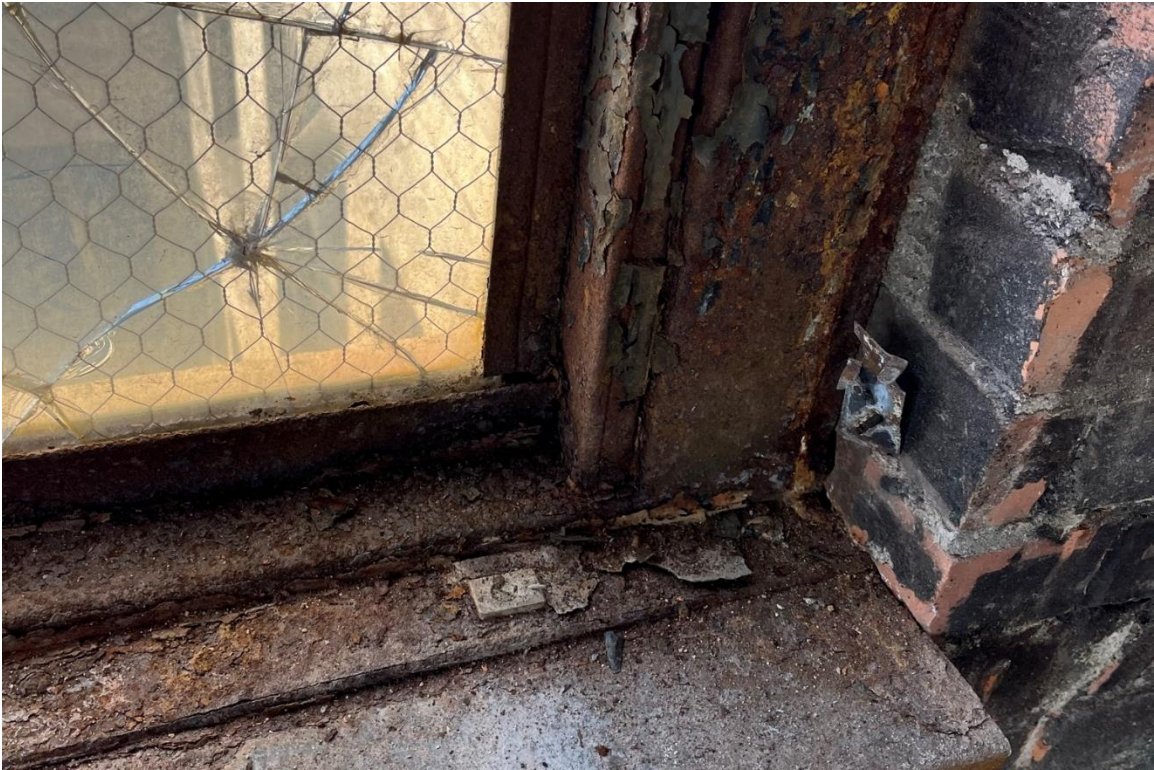
Window #24, 5 th Floor, South courtyard elevation, 04/03/23.
