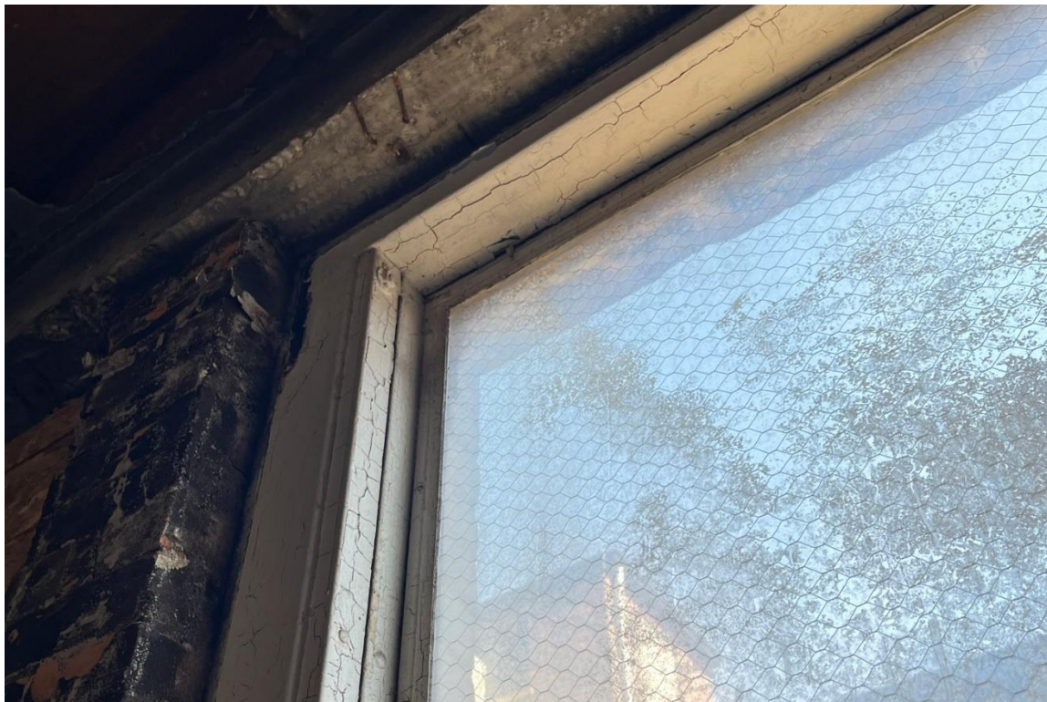
Window #31, 3 rd Floor, North elevation, 04/03/23.
