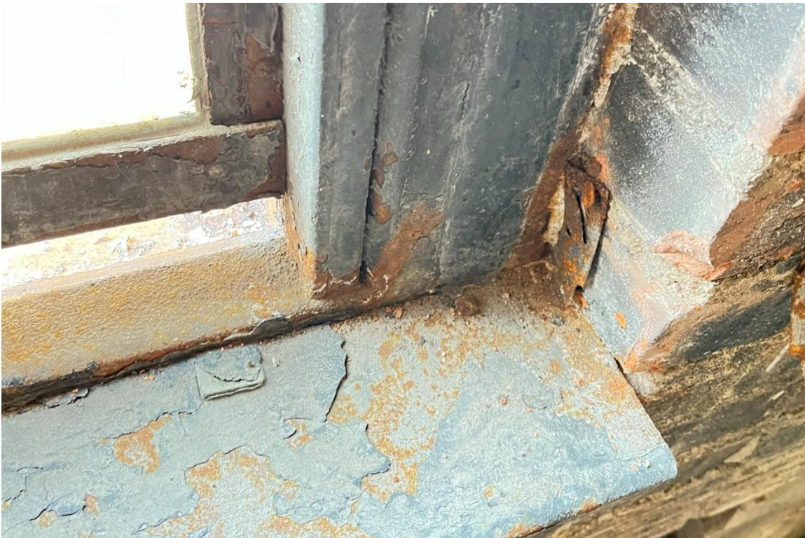
Window #29, 4 th Floor, North elevation, 04/03/23.
