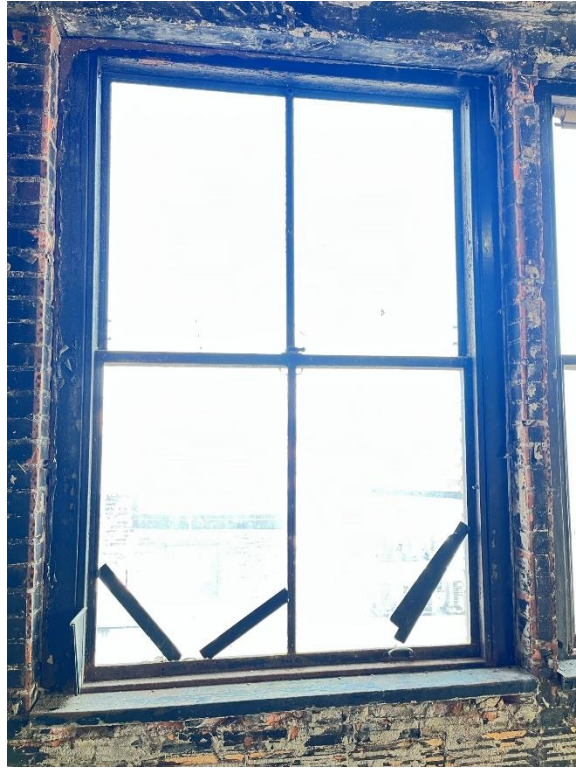
Window #20, 6 th Floor, North elevation, 04/03/23.
