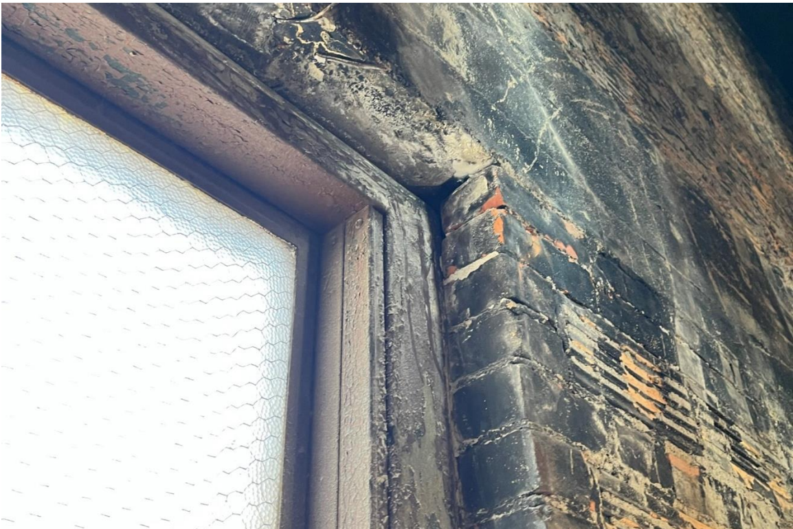
Window #26, 4 th Floor, West elevation, 04/03/23.
