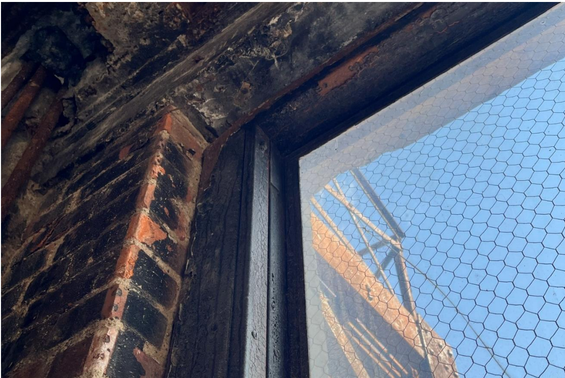
Window #20, 6 th Floor, North elevation, 04/03/23.
