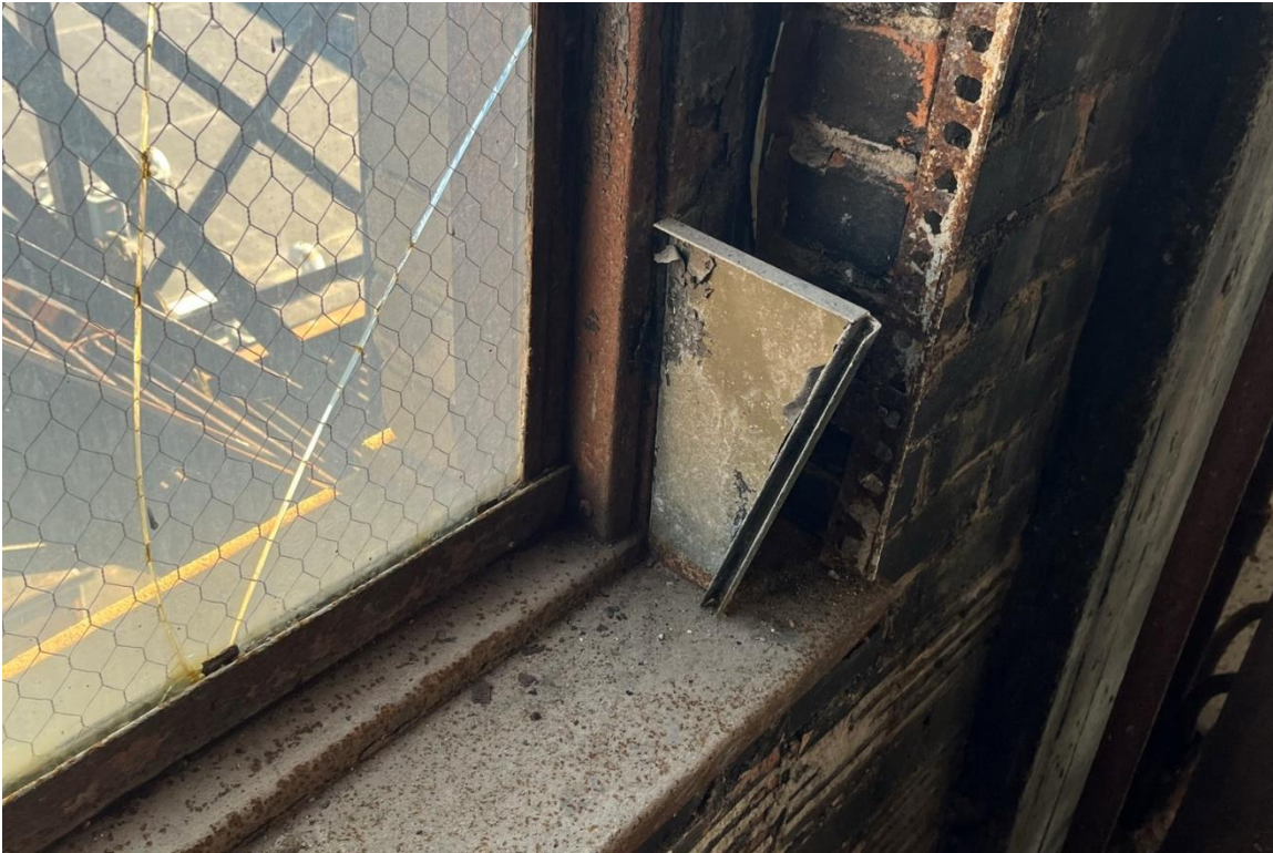
Window #12, 8 th Floor, North elevation, 04/03/23.
