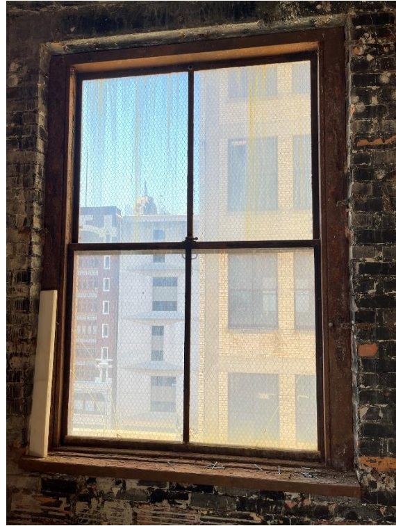
Window #19, 6 th Floor, South courtyard elevation, 04/03/23.
