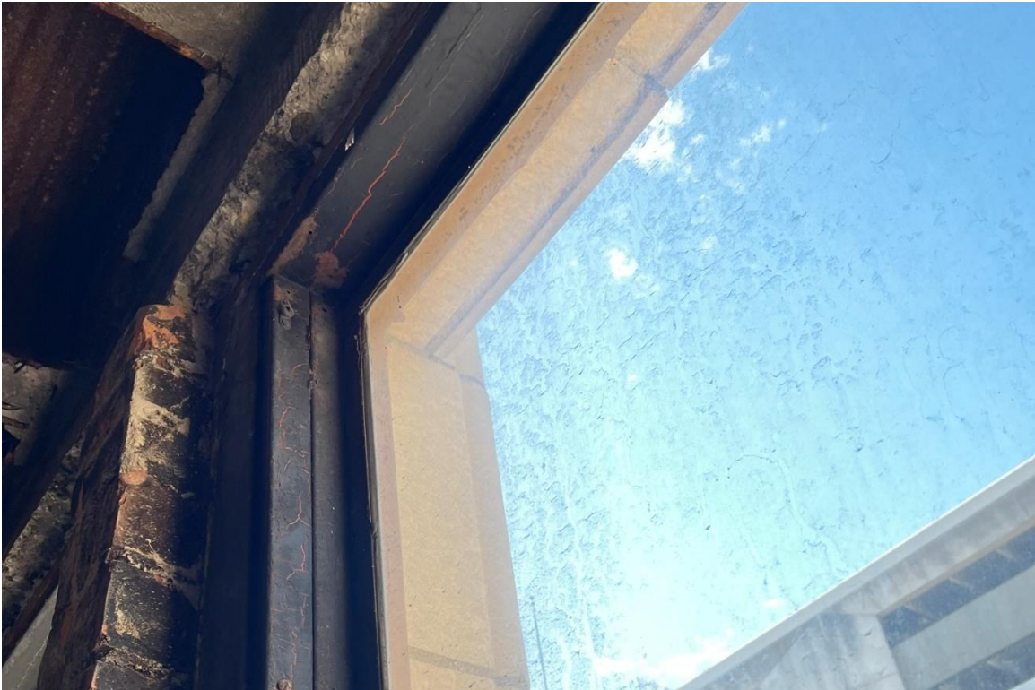
Window #29, 4 th Floor, North elevation, 04/03/23.
