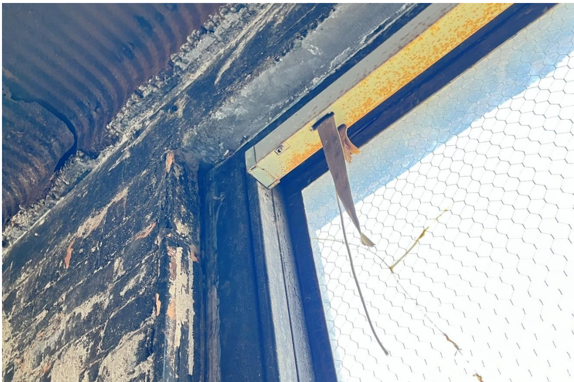
Window #9, 8 th Floor, West elevation, 04/03/23.
