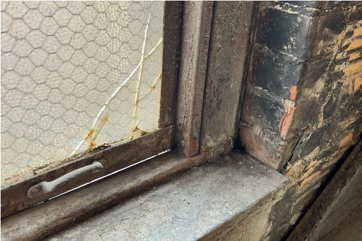
Window #26, 4 th Floor, West elevation, 04/03/23.
