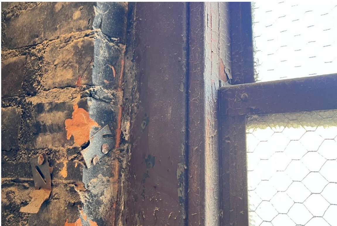
Window #17, 6 th Floor, West elevation, 04/03/23.
