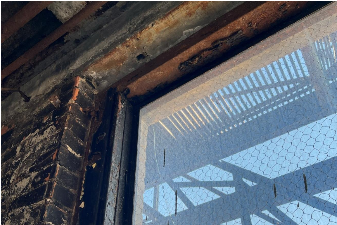
Window #12, 8 th Floor, North elevation, 04/03/23.
