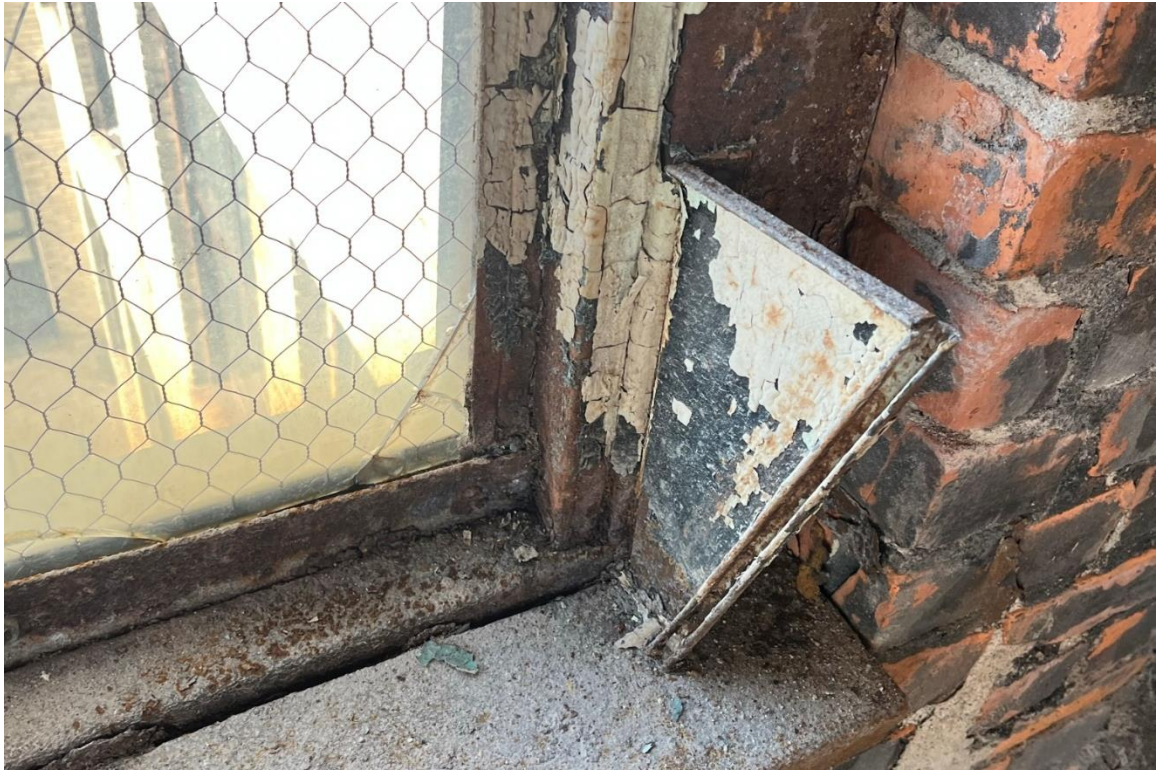
Window #7, 9 th Floor, South courtyard elevation, 04/03/23.
