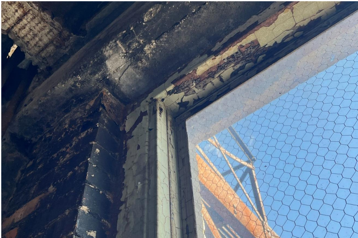
Window #8, 9 th Floor, North elevation, 04/03/23.
