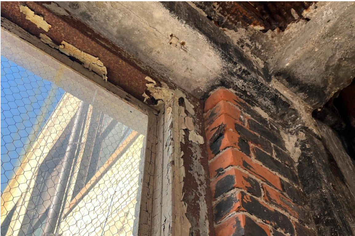
Window #7, 9 th Floor, South courtyard elevation, 04/03/23.
