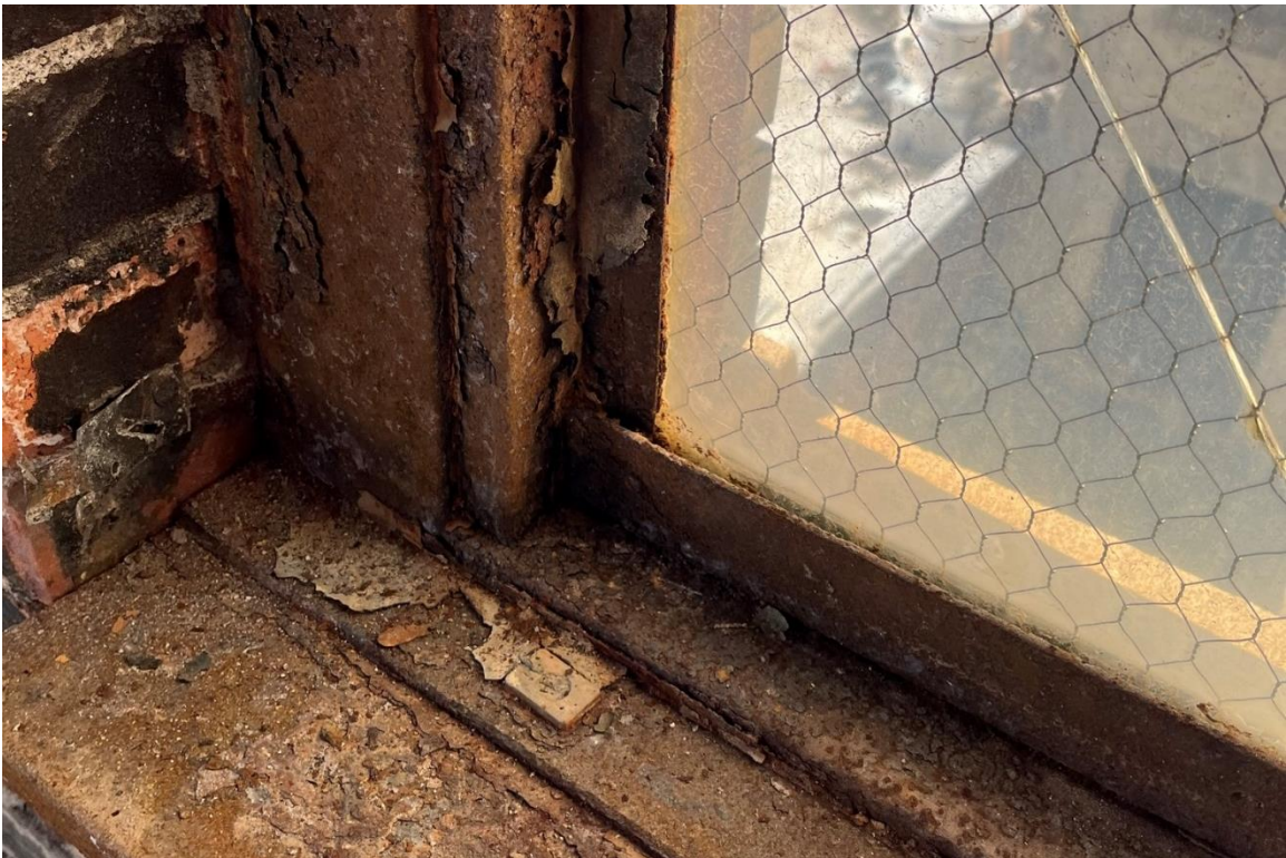
Window #24, 5 th Floor, South courtyard elevation, 04/03/23.
