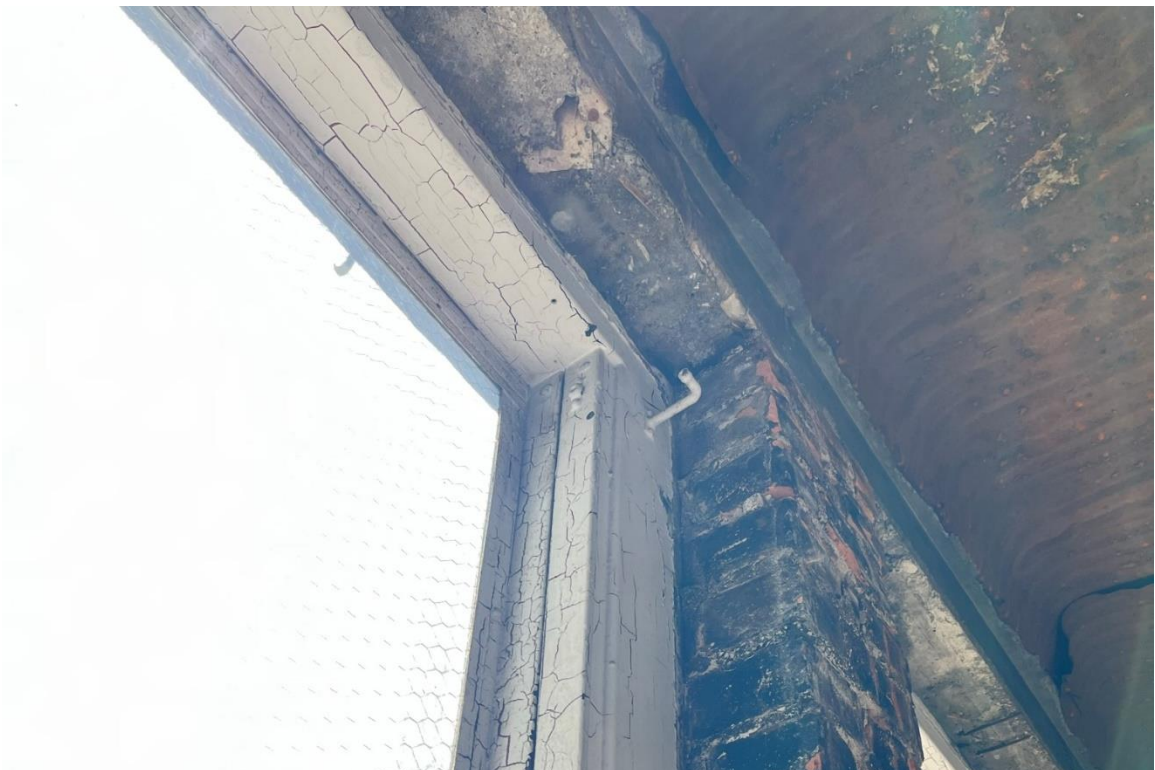
Window #30, 3 rd Floor, East elevation, 04/03/23.
