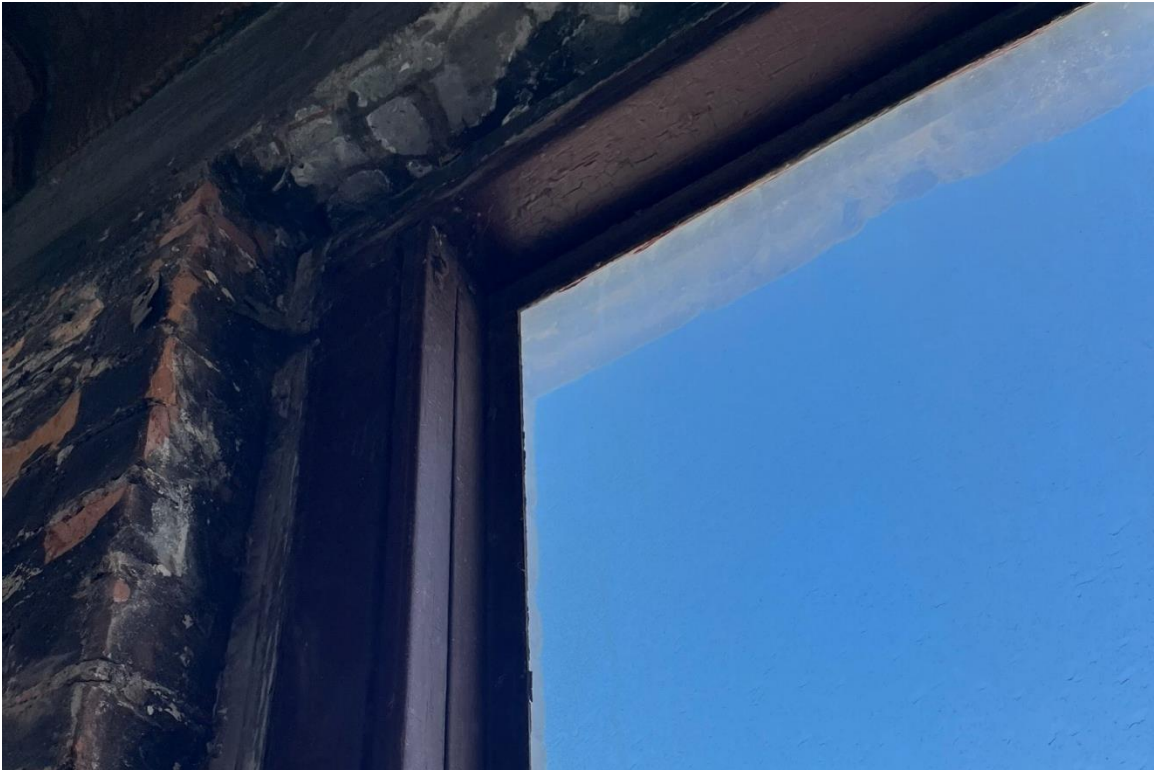
Window #21, 5 th Floor, West elevation, 04/03/23.
