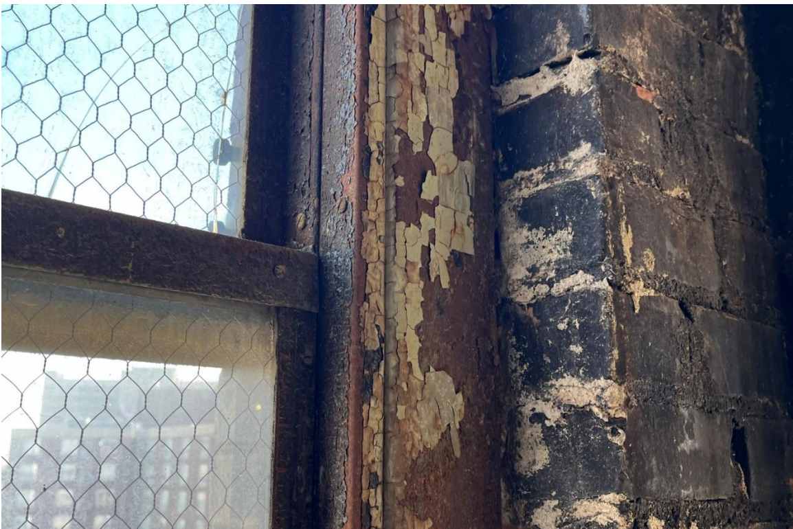
Window #16, 7 th Floor, North elevation, 04/03/23.
