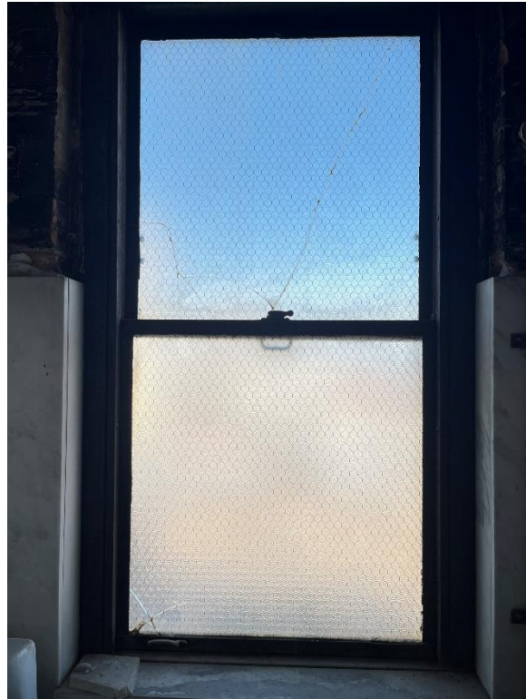
Window #4, 10 th Floor, West elevation, 04/03/23.
