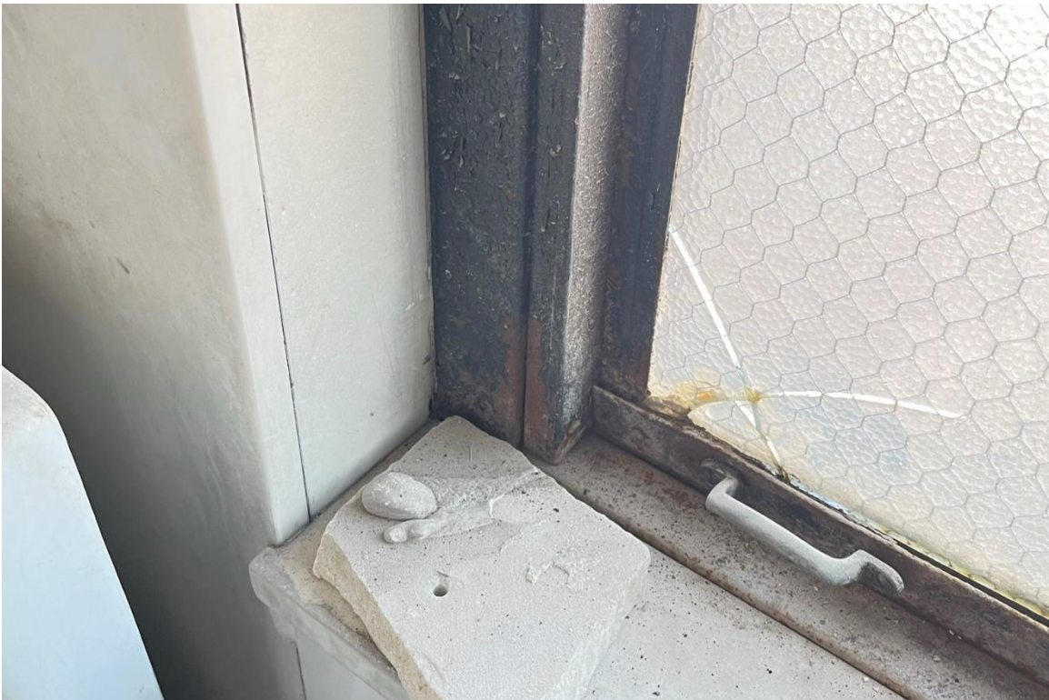
Window #4, 10 th Floor, West elevation, 04/03/23.
