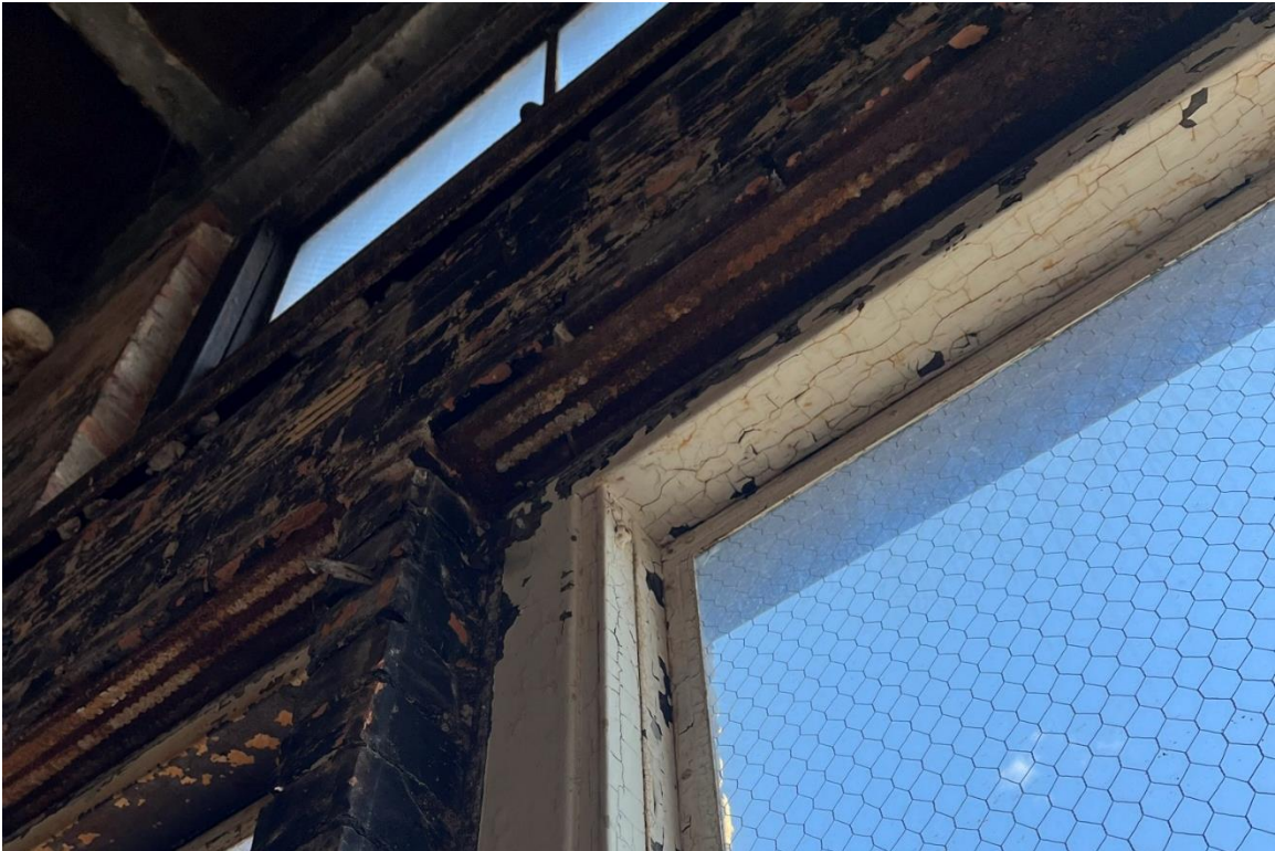
Window #3, 10 th Floor, North elevation, 04/03/23.
