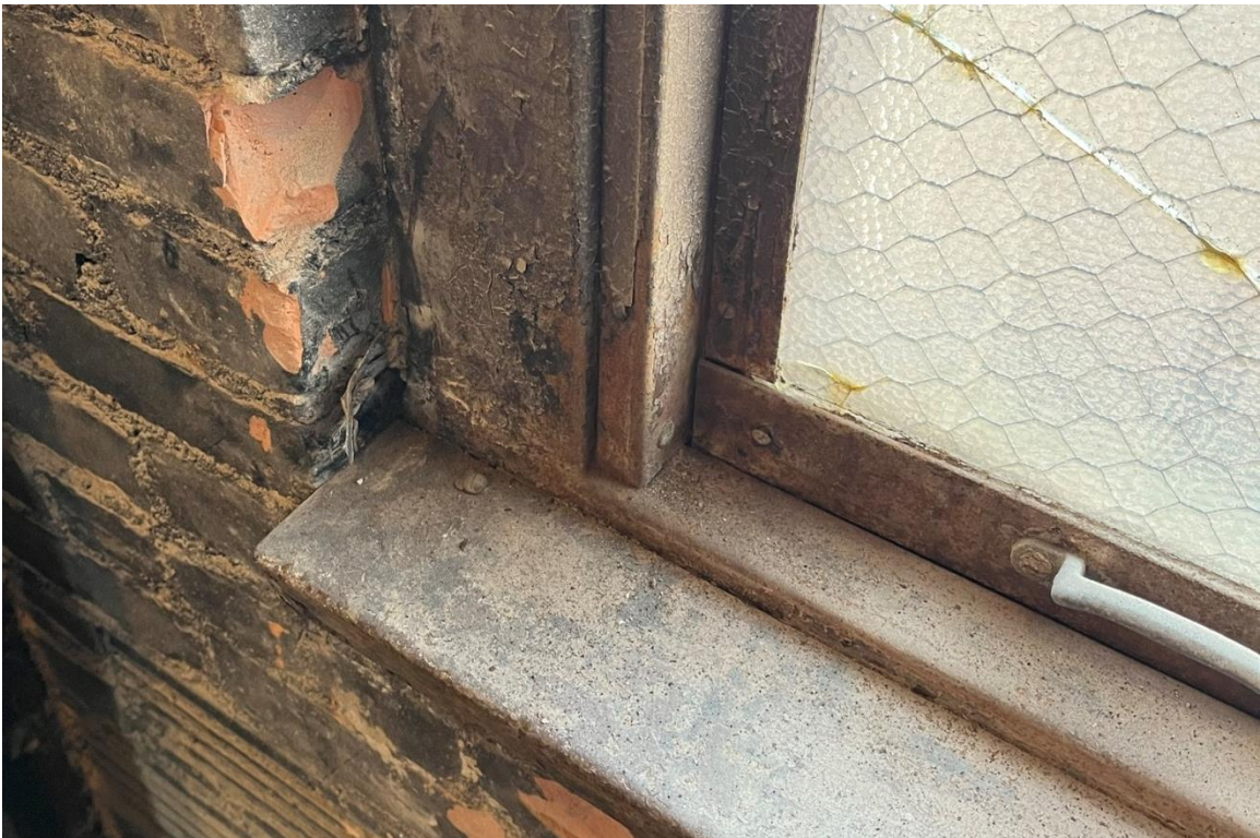
Window #17, 6 th Floor, West elevation, 04/03/23.
