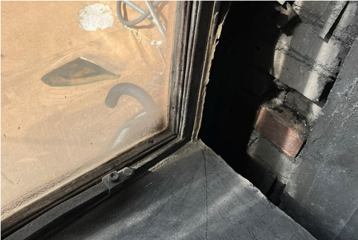
Window #34, Mezzanine, South elevation, 04/03/23.
