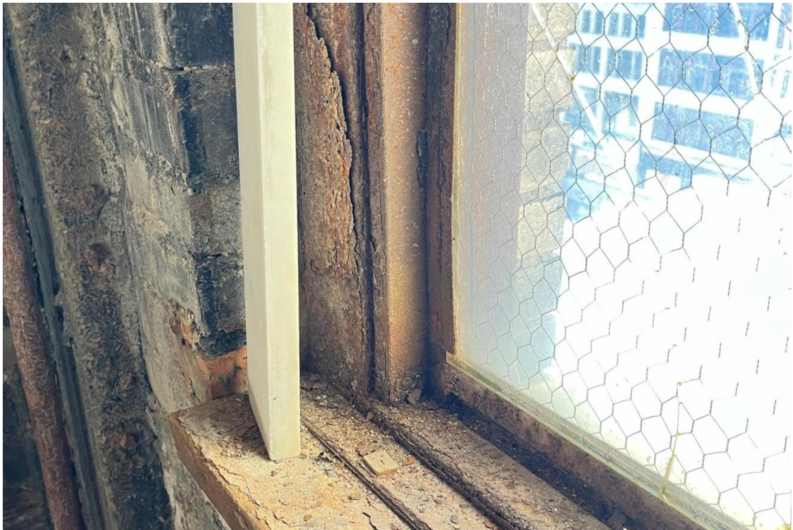
Window #19, 6 th Floor, South courtyard elevation, 04/03/23.
