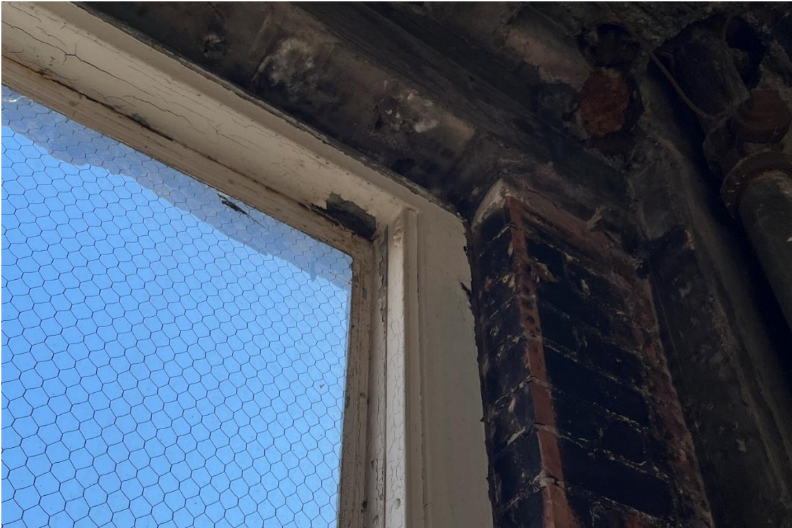
Window #25, 5 th Floor, North elevation, 04/03/23.
