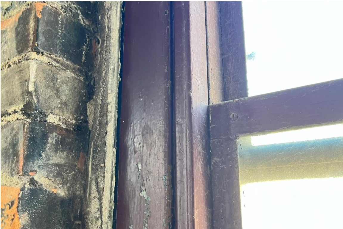
Window #21, 5 th Floor, West elevation, 04/03/23.
