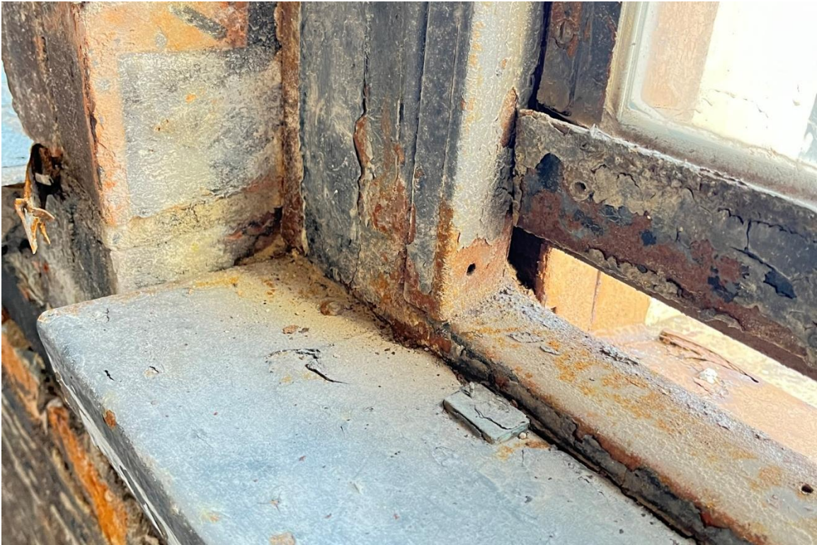
Window #29, 4 th Floor, North elevation, 04/03/23.
