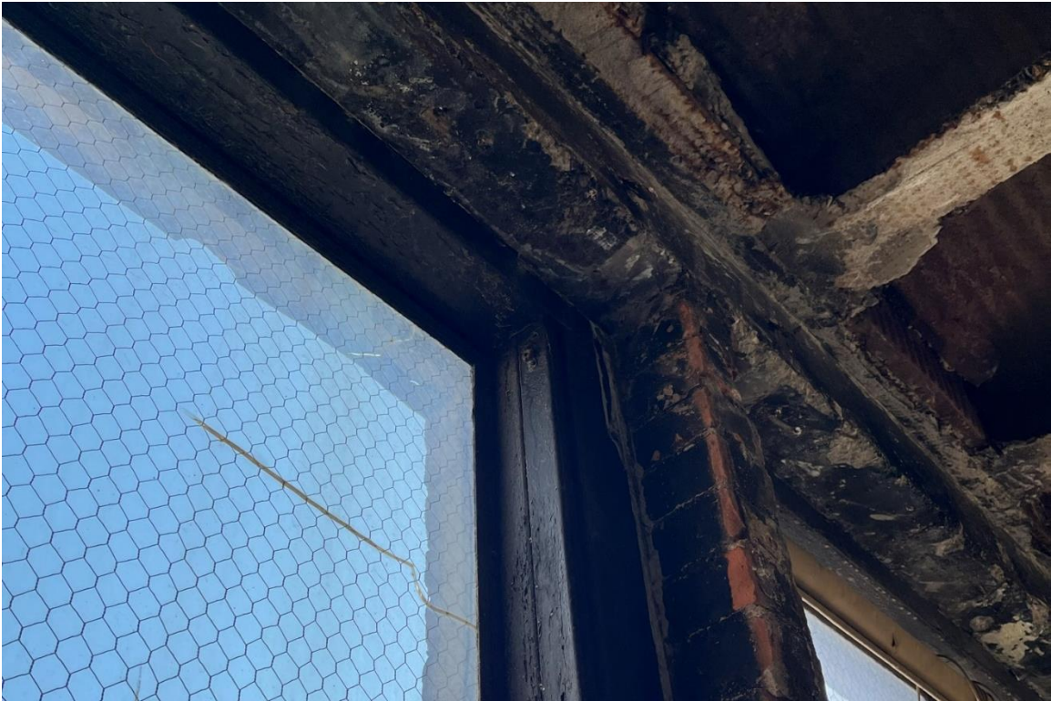
Window #20, 6 th Floor, North elevation, 04/03/23.
