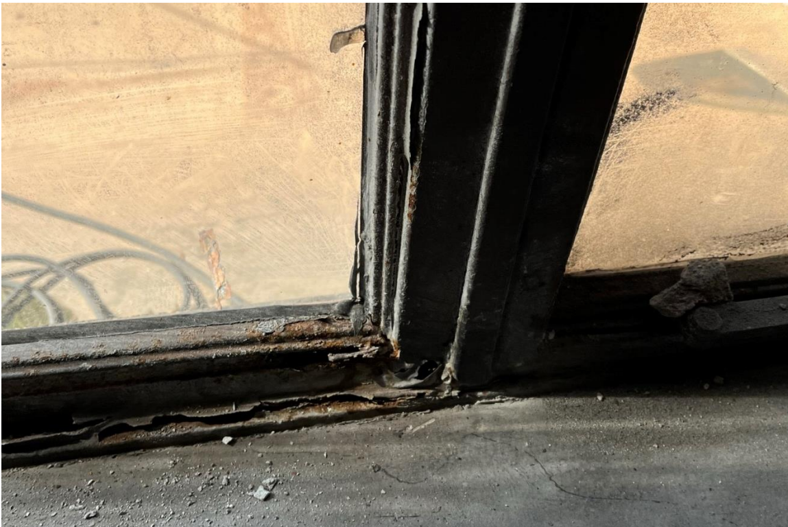
Window #34, Mezzanine, South elevation, 04/03/23.
