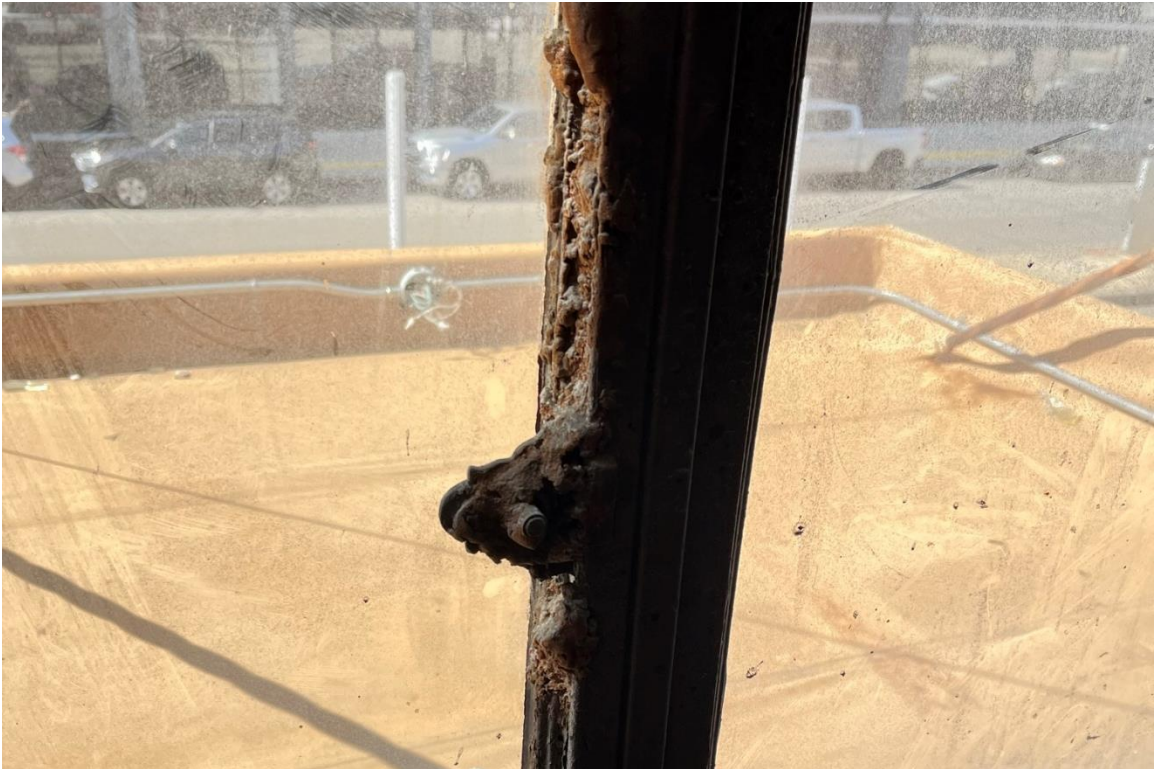
Window #34, Mezzanine, South elevation, 04/03/23.
