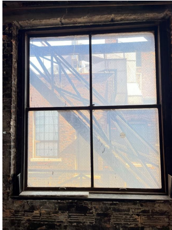
Window #28, 4 th Floor, North elevation, 04/03/23.
