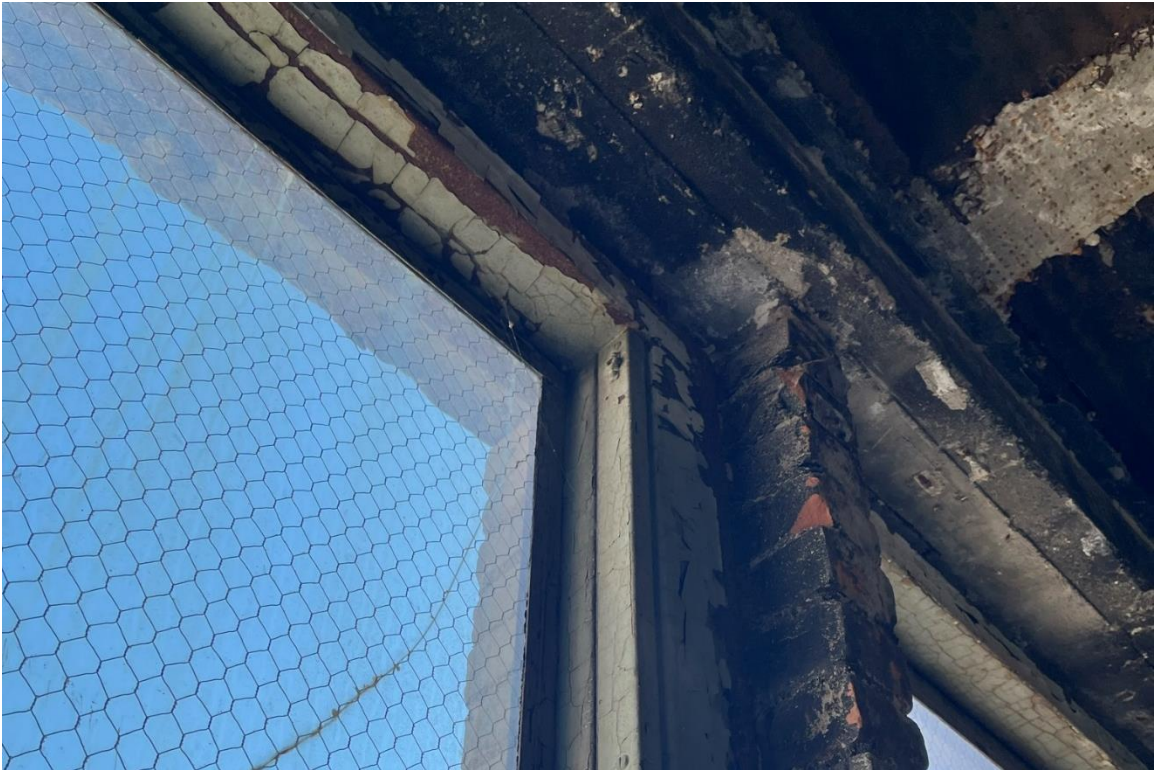
Window #8, 9 th Floor, North elevation, 04/03/23.
