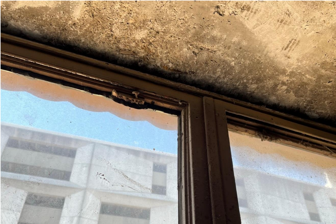
Window #34, Mezzanine, South elevation, 04/03/23.
