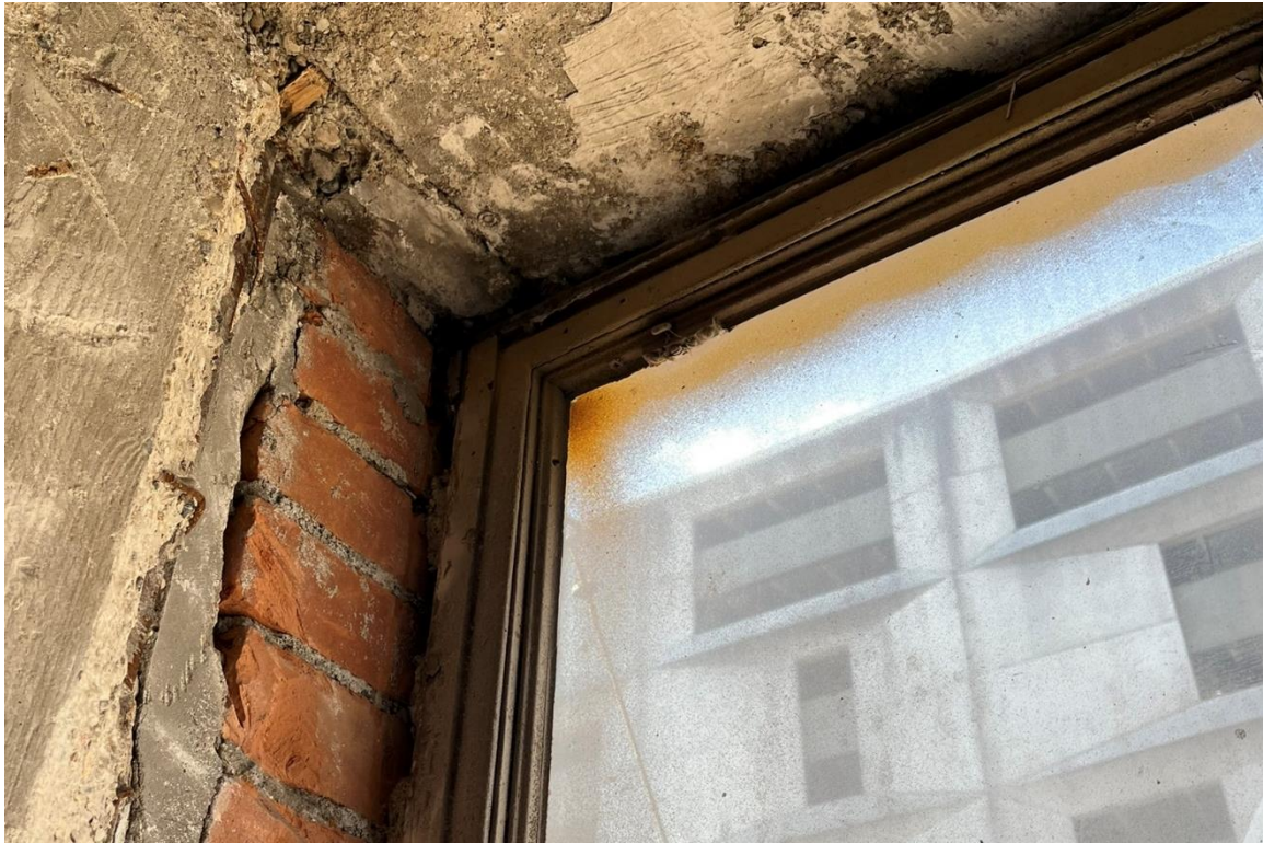
Window #34, Mezzanine, South elevation, 04/03/23.
