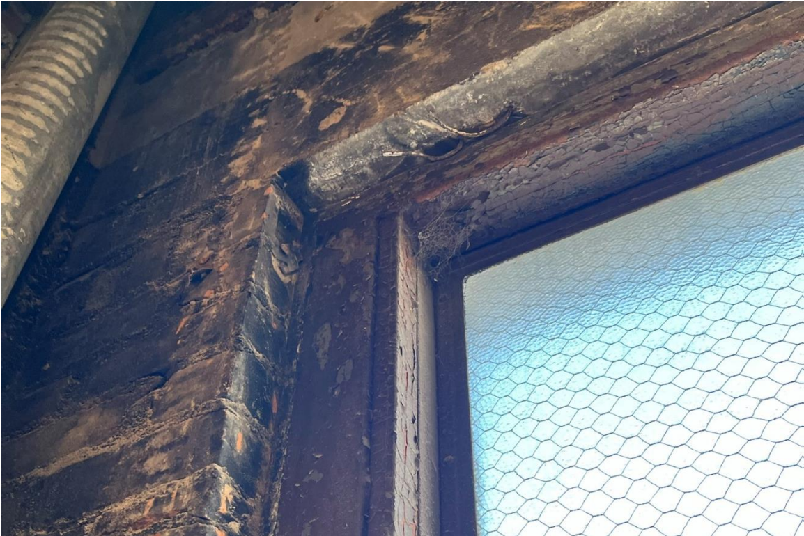
Window #17, 6 th Floor, West elevation, 04/03/23.
