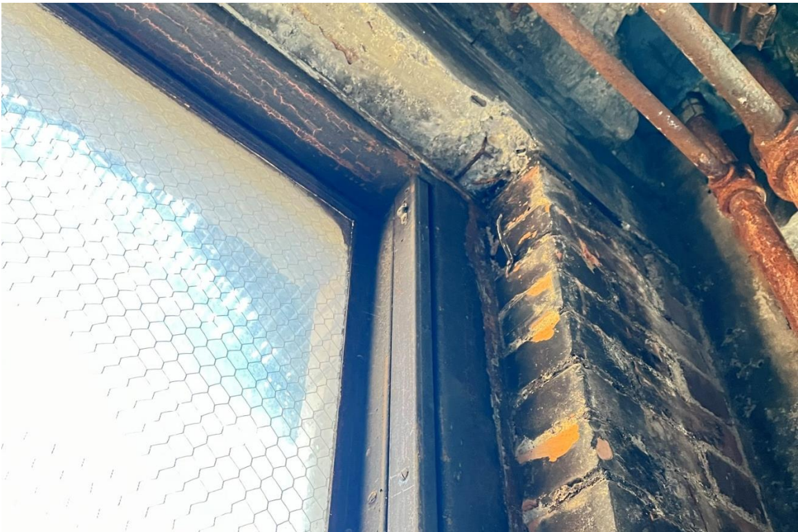
Window #28, 4 th Floor, North elevation, 04/03/23.
