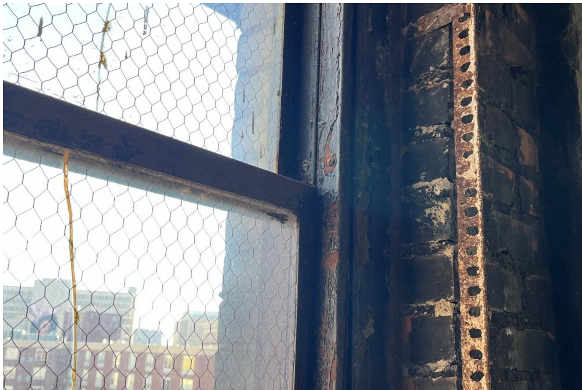
Window #12, 8 th Floor, North elevation, 04/03/23.
