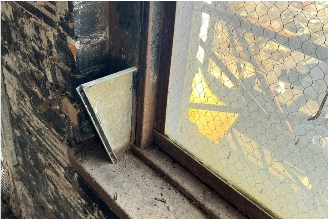
Window #12, 8 th Floor, North elevation, 04/03/23.
