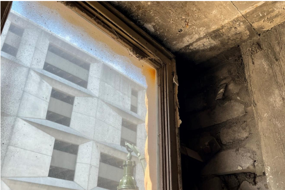
Window #34, Mezzanine, South elevation, 04/03/23.
