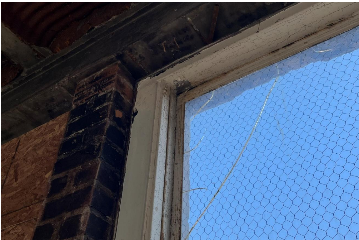
Window #25, 5 th Floor, North elevation, 04/03/23.
