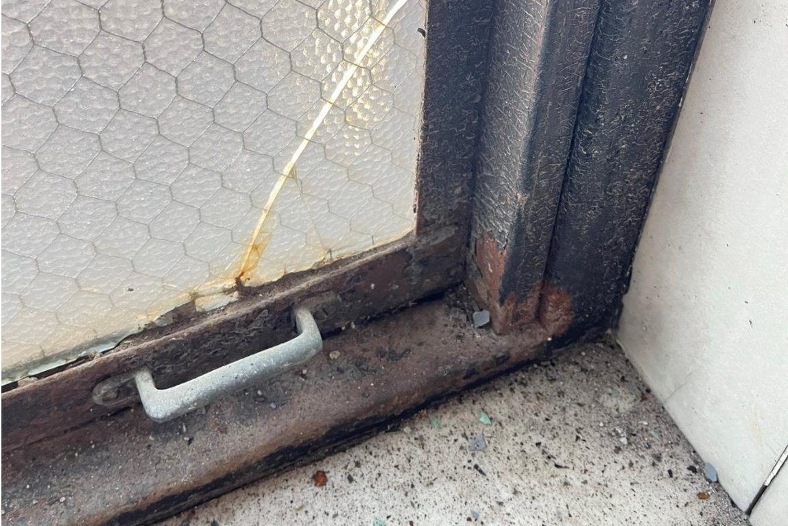
Window #13, 8 th Floor, West elevation, 04/03/23.
