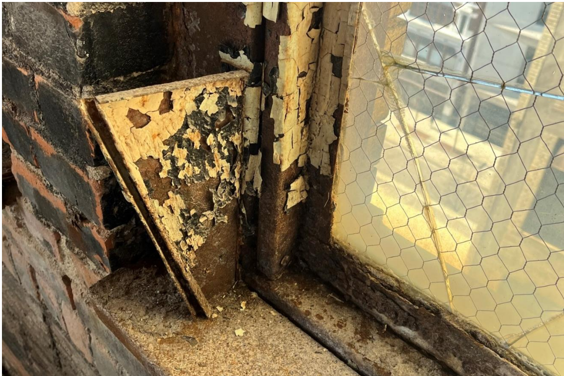
Window #7, 9 th Floor, South courtyard elevation, 04/03/23.
