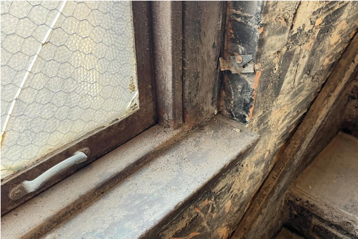
Window #17, 6 th Floor, West elevation, 04/03/23.
