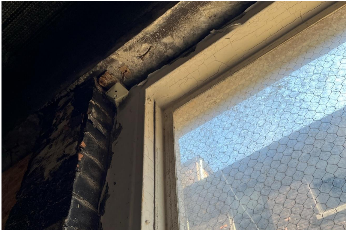
Window #33, 2 nd Floor, North elevation, 04/03/23.
