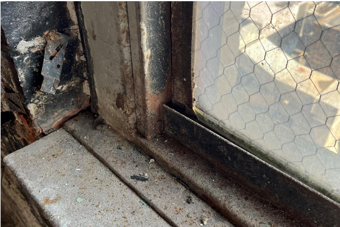
Window #16, 7 th Floor, North elevation, 04/03/23.
