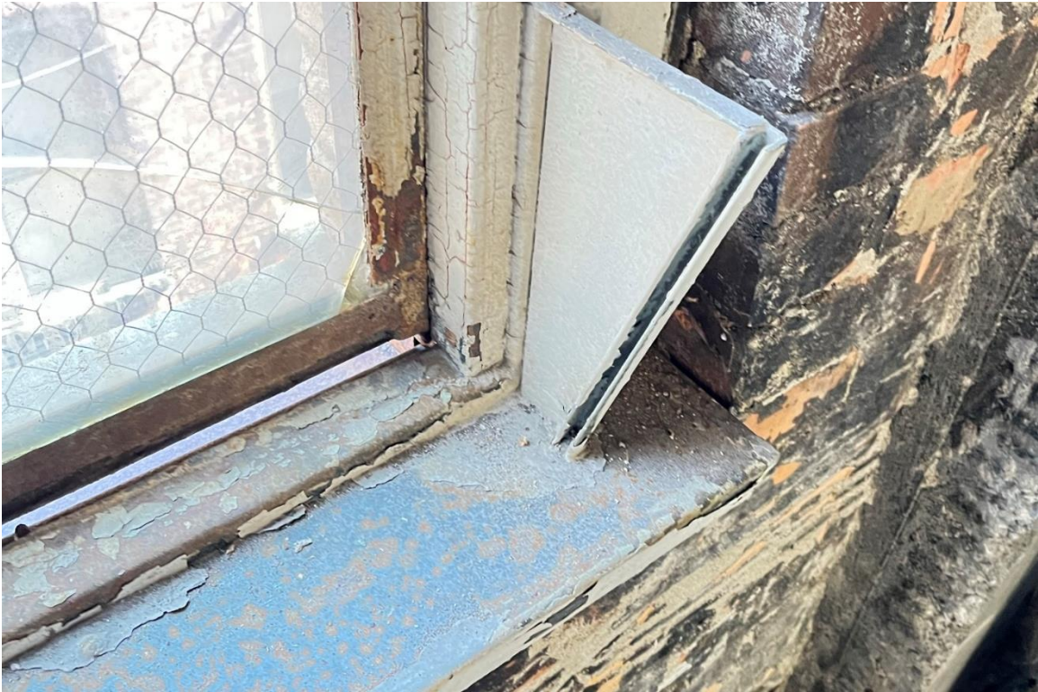
Window #31, 3 rd Floor, North elevation, 04/03/23.
