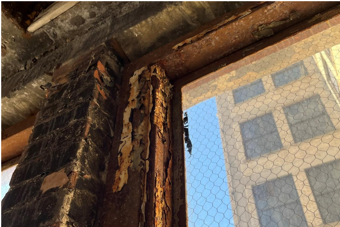
Window #24, 5 th Floor, South courtyard elevation, 04/03/23.
