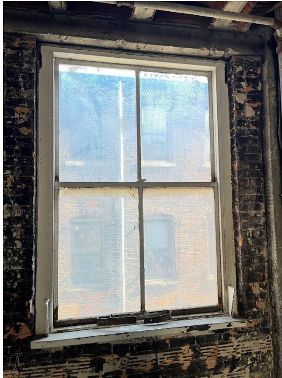
Window #31, 3 rd Floor, North elevation, 04/03/23.
