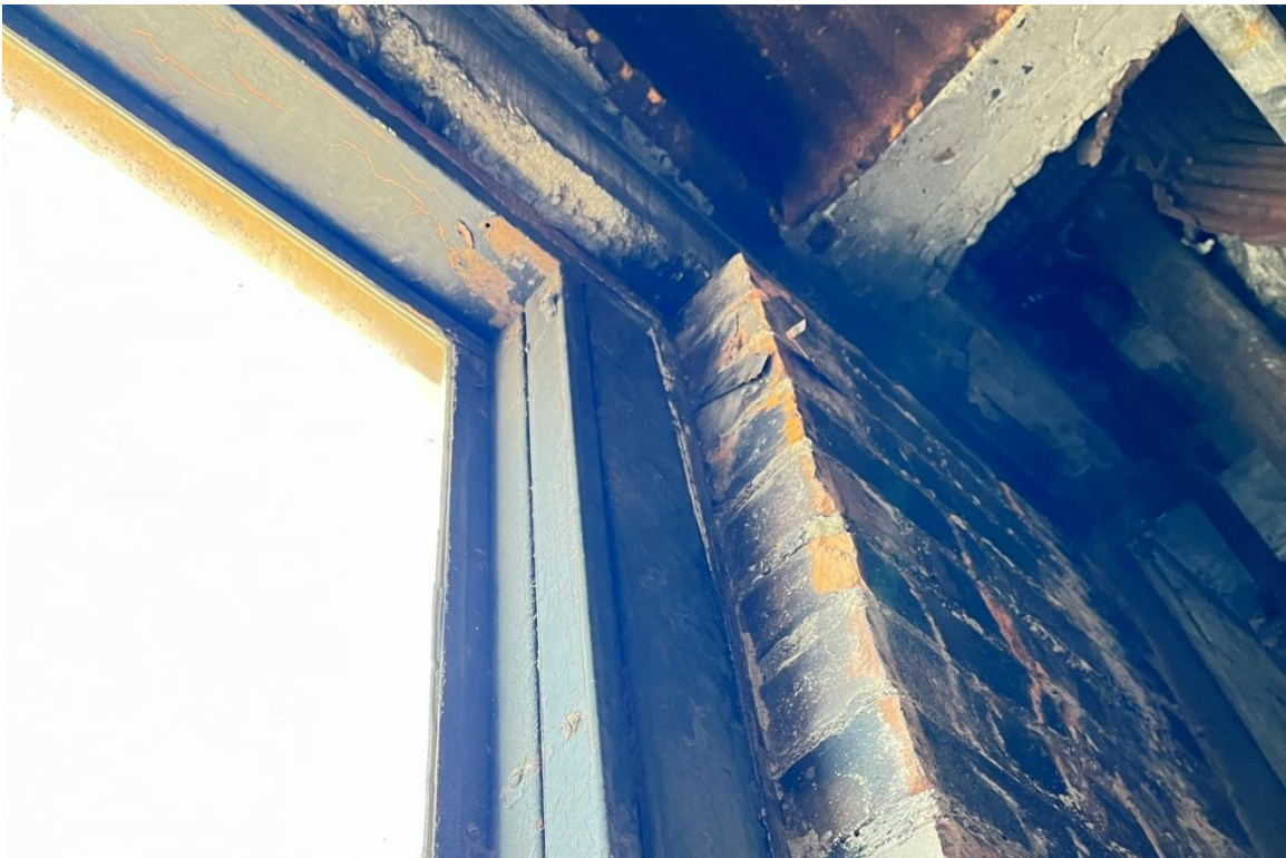
Window #29, 4 th Floor, North elevation, 04/03/23.
