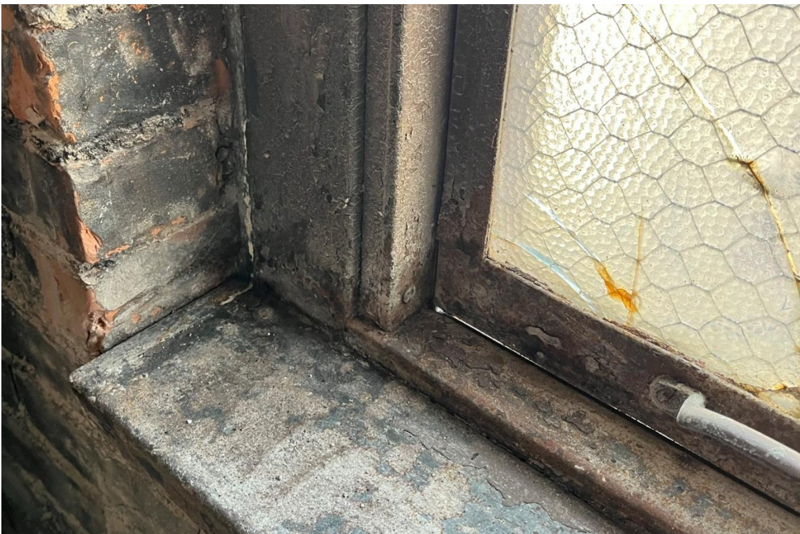
Window #26, 4 th Floor, West elevation, 04/03/23.
