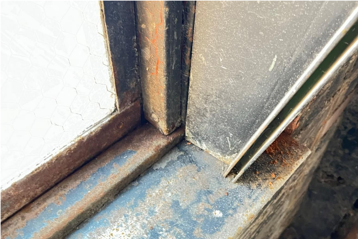
Window #28, 4 th Floor, North elevation, 04/03/23.
