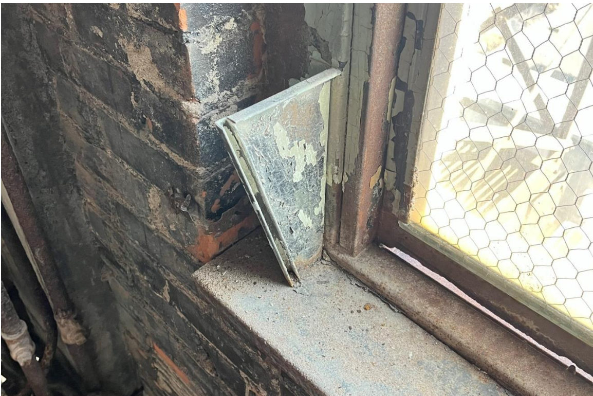
Window #8, 9 th Floor, North elevation, 04/03/23.
