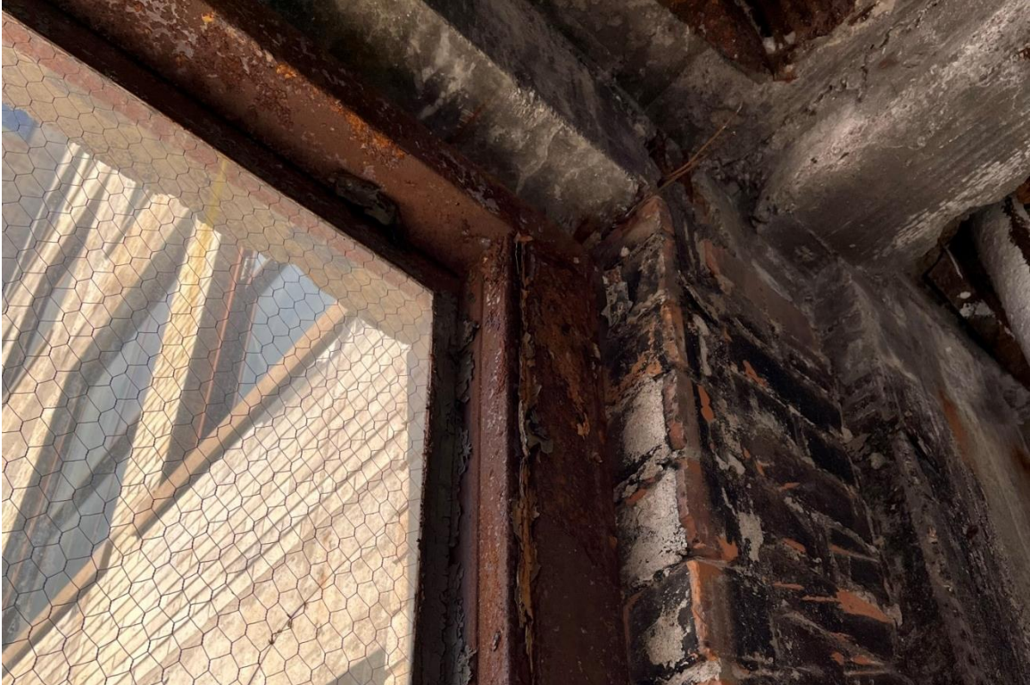
Window #24, 5 th Floor, South courtyard elevation, 04/03/23.
