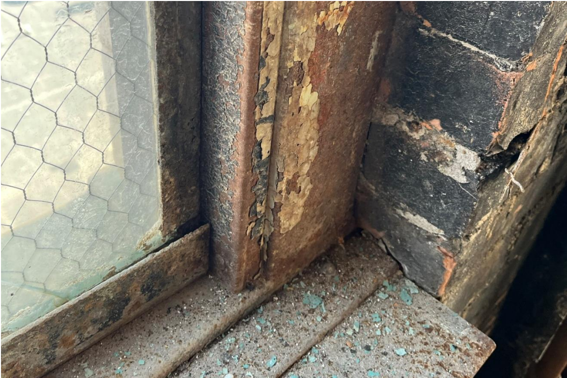
Window #16, 7 th Floor, North elevation, 04/03/23.
