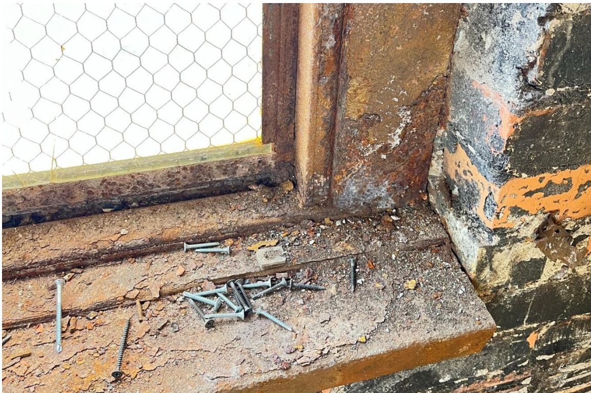
Window #19, 6 th Floor, South courtyard elevation, 04/03/23.
