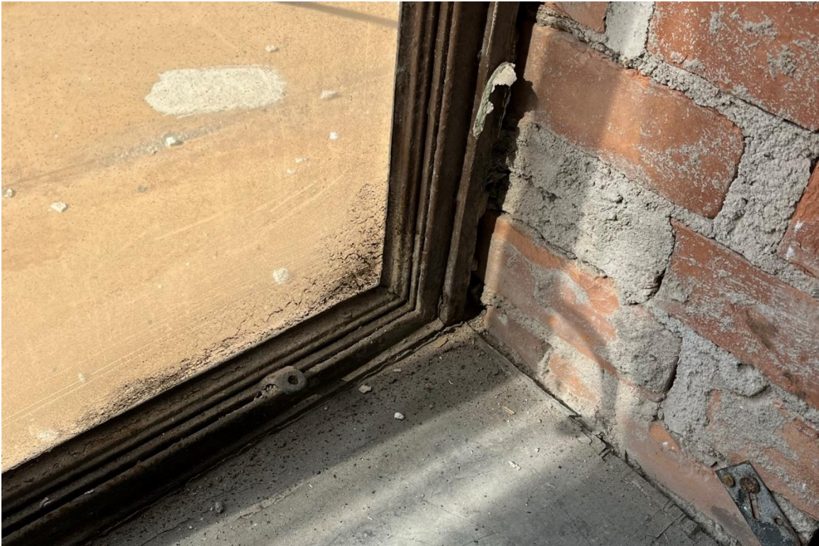
Window #35, Mezzanine, South elevation, 04/03/23.
