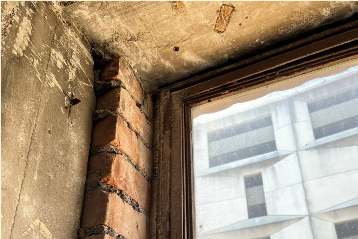
Window #35, Mezzanine, South elevation, 04/03/23.
