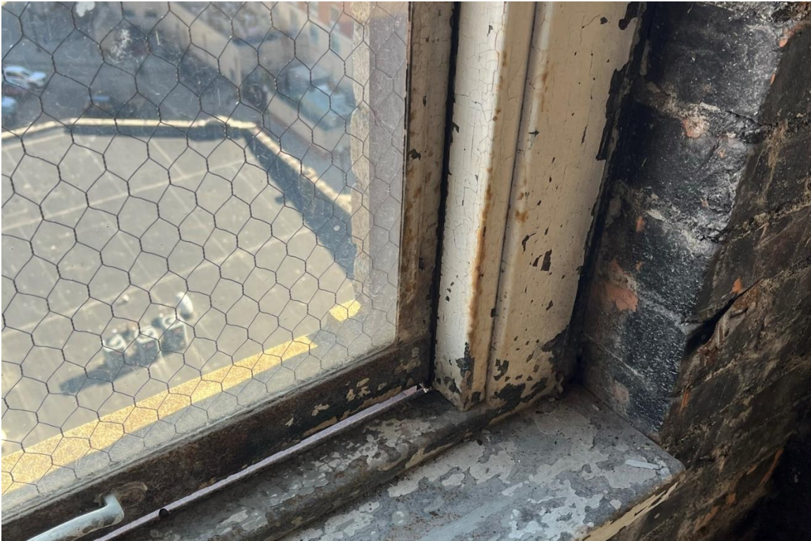
Window #3, 10 th Floor, North elevation, 04/03/23.
