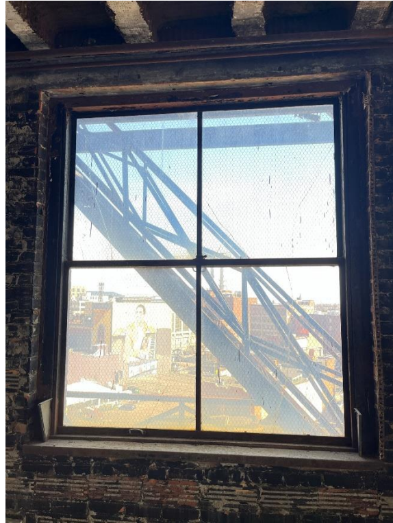
Window #12, 8 th Floor, North elevation, 04/03/23.
