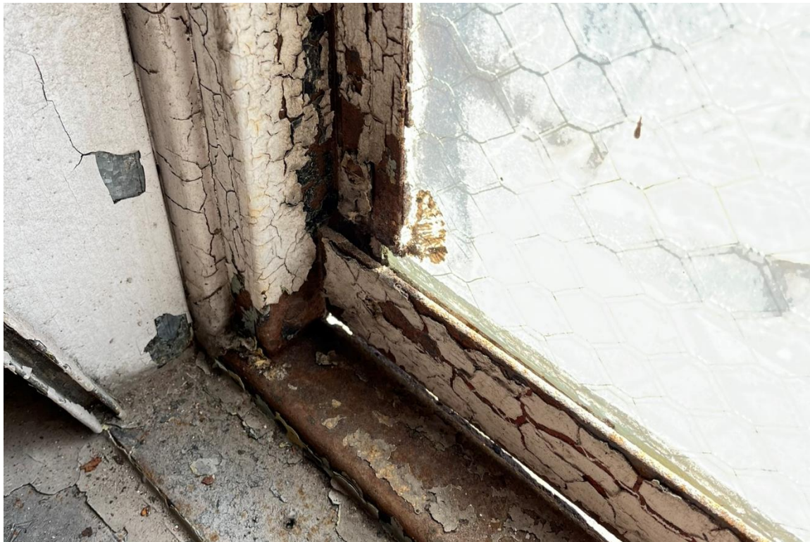
Window #30, 3 rd Floor, East elevation, 04/03/23.
