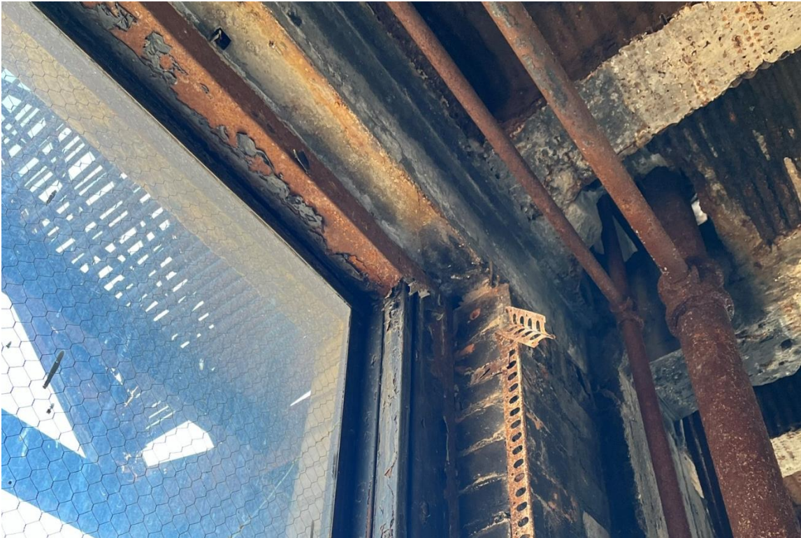
Window #12, 8 th Floor, North elevation, 04/03/23.
