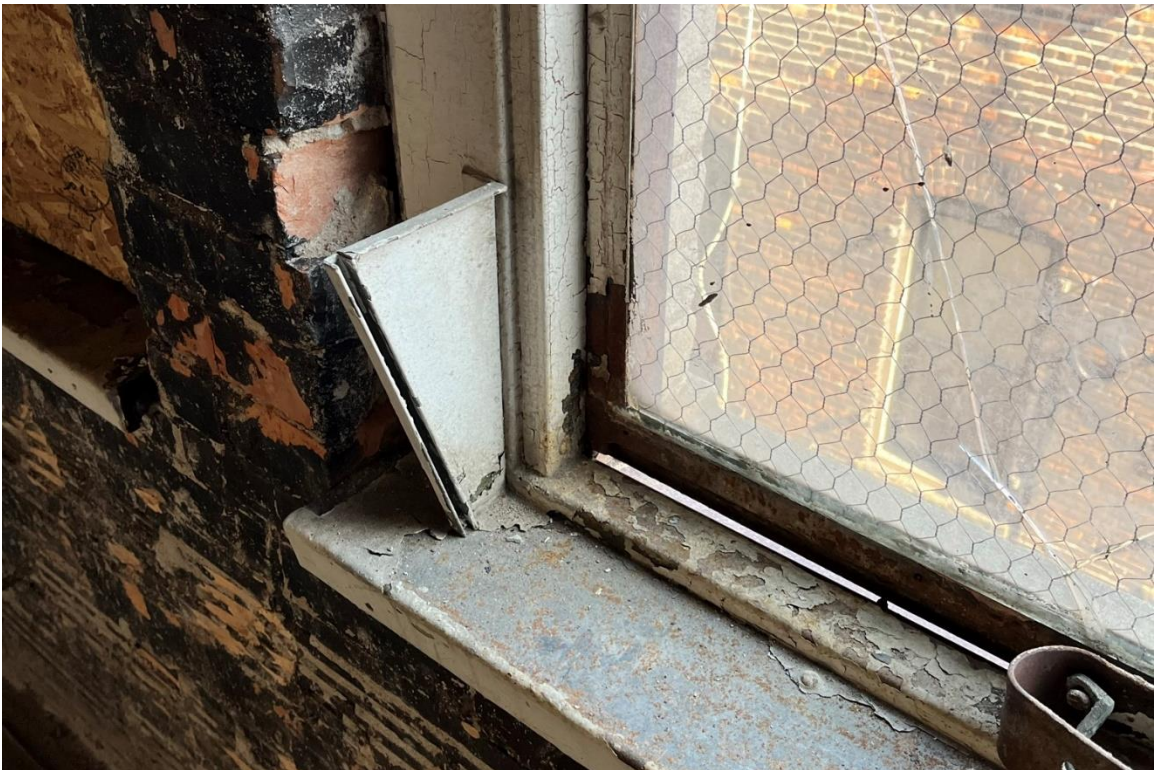
Window #31, 3 rd Floor, North elevation, 04/03/23.
