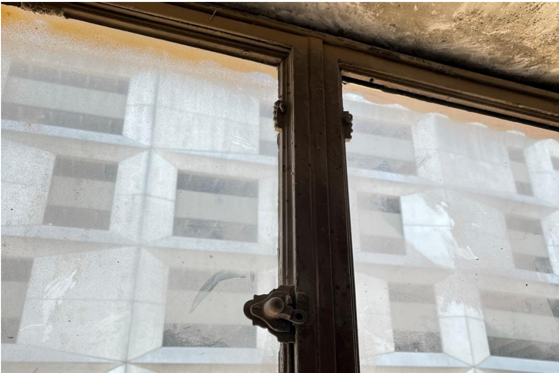
Window #34, Mezzanine, South elevation, 04/03/23.
