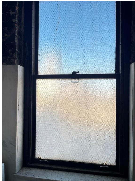
Window #13, 8 th Floor, West elevation, 04/03/23.
