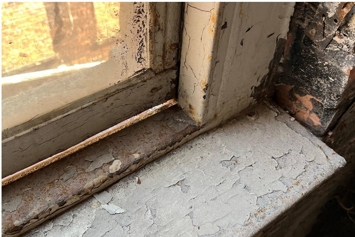
Window #33, 2 nd Floor, North elevation, 04/03/23.
