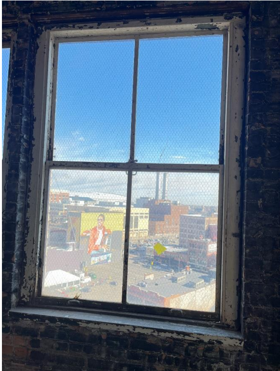
Window #3, 10 th Floor, North elevation, 04/03/23.
