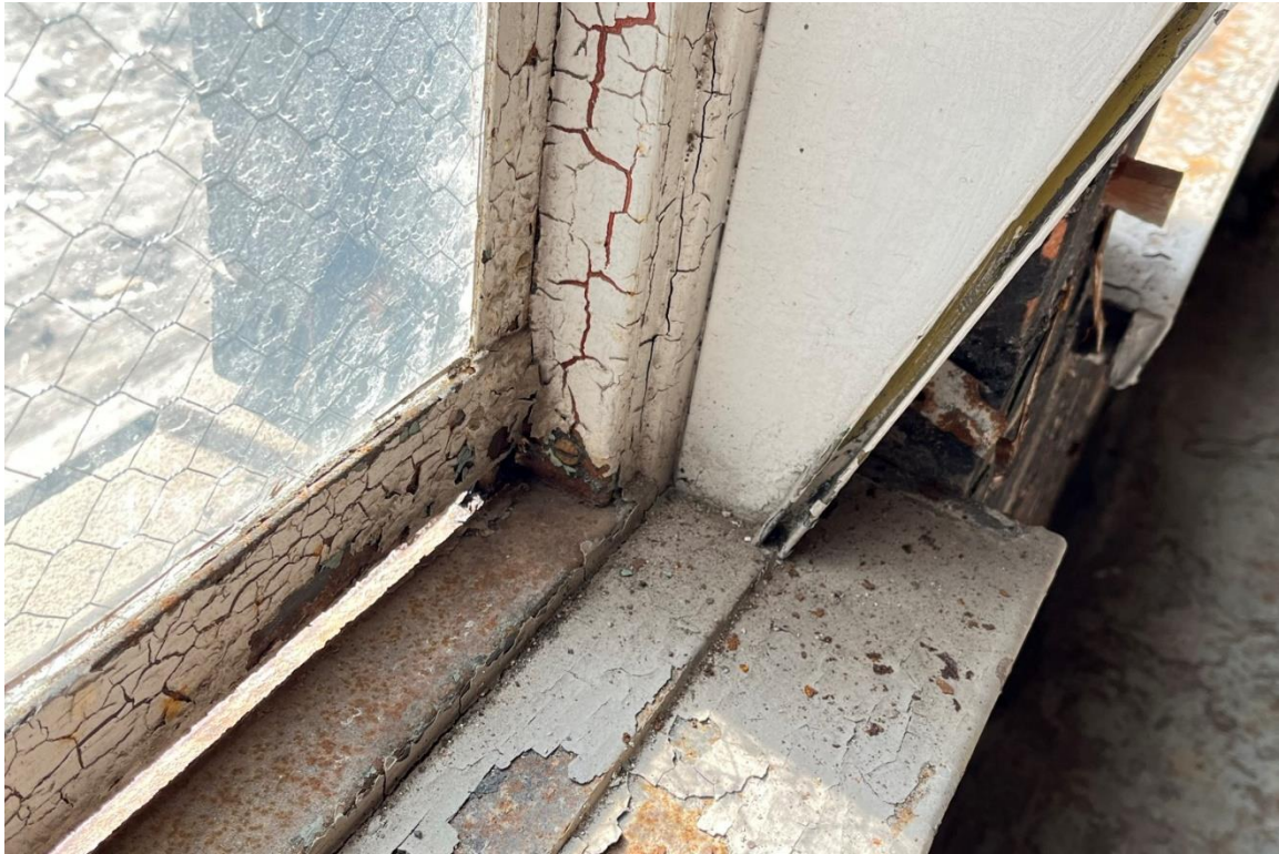
Window #30, 3 rd Floor, East elevation, 04/03/23.
