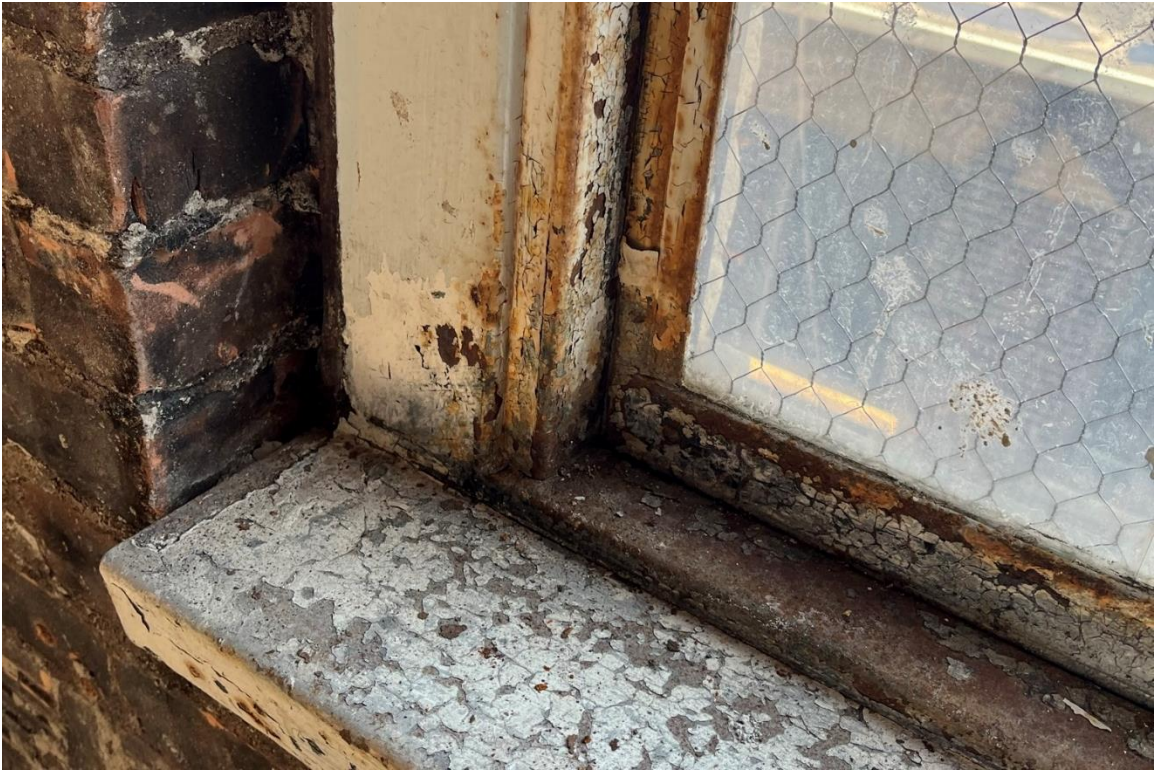
Window #25, 5 th Floor, North elevation, 04/03/23.
