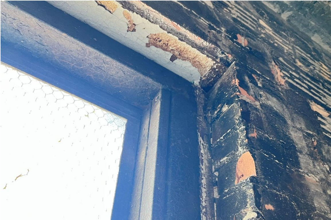
Window #4, 10 th Floor, West elevation, 04/03/23.
