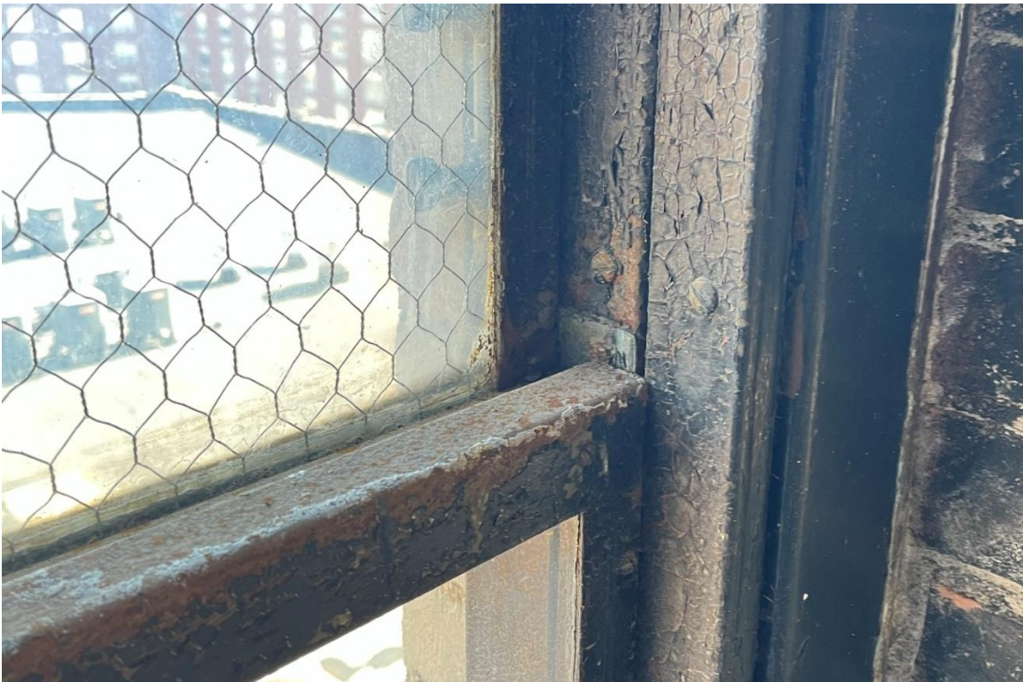
Window #20, 6 th Floor, North elevation, 04/03/23.
