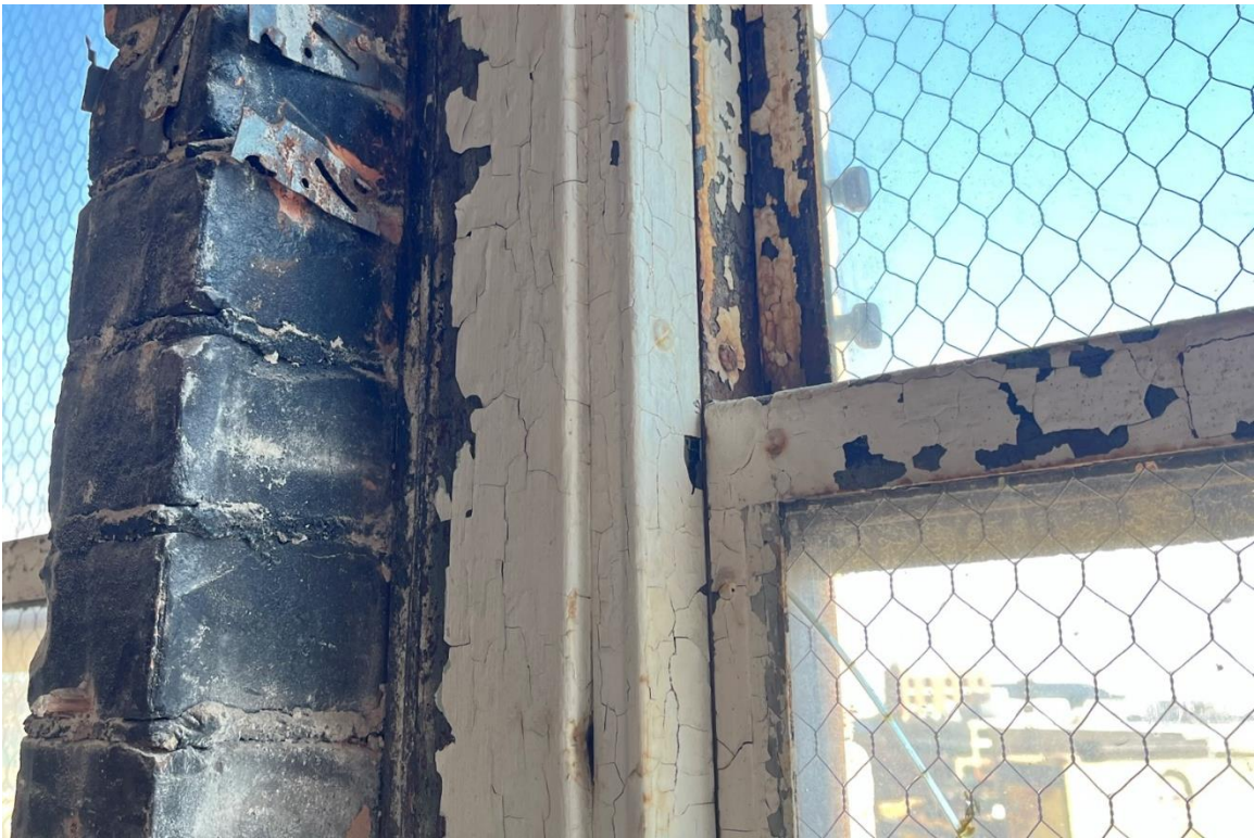
Window #3, 10 th Floor, North elevation, 04/03/23.
