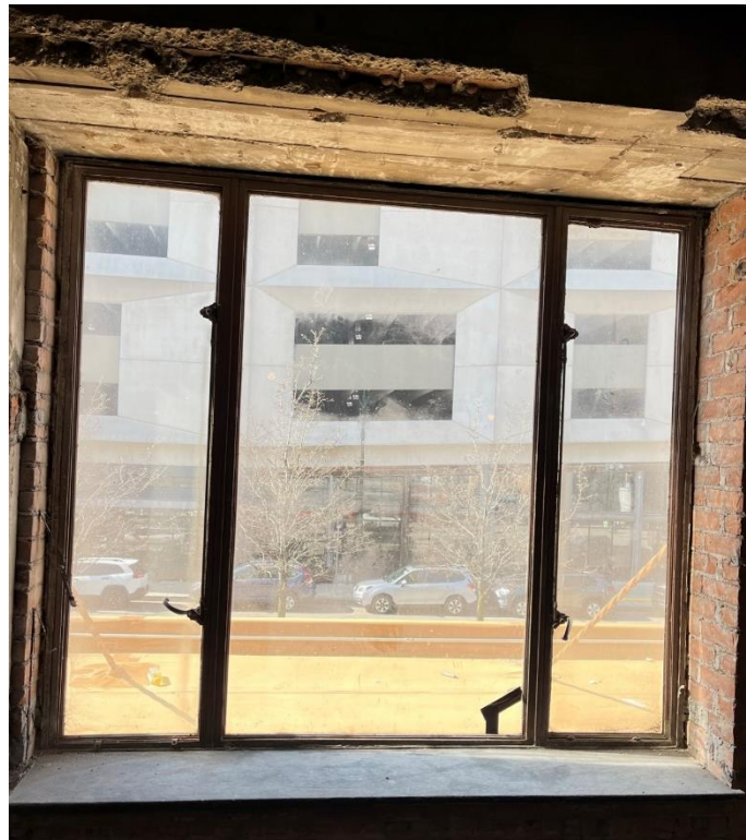
Window #35, Mezzanine, South elevation, 04/03/23.
