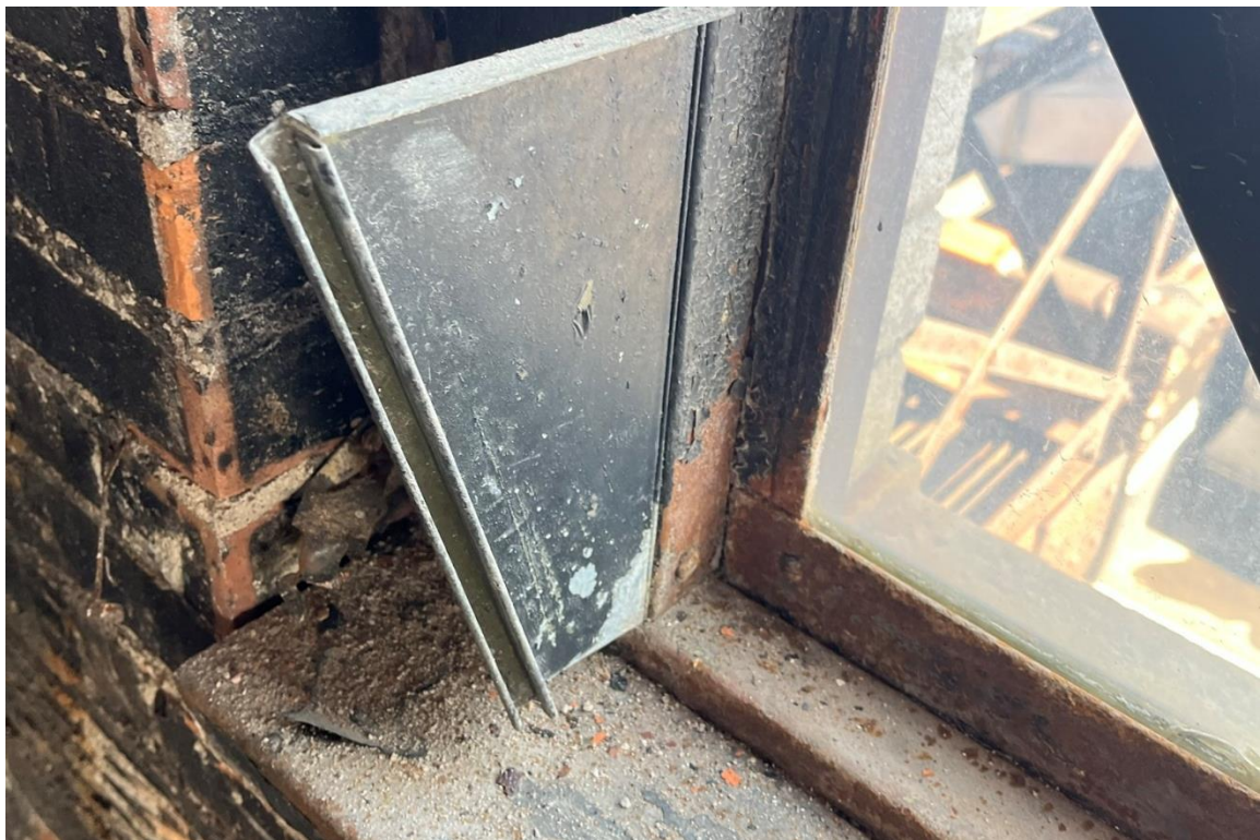
Window #20, 6 th Floor, North elevation, 04/03/23.
