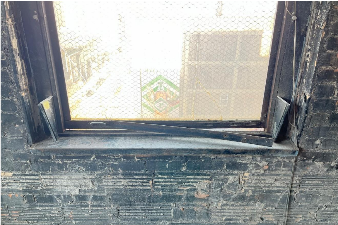
Window #9, 8 th Floor, West elevation, 04/03/23.
