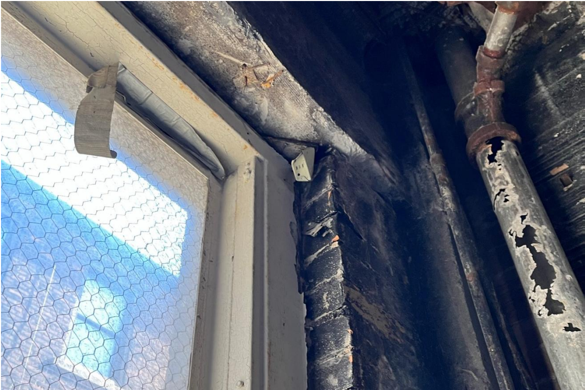
Window #33, 2 nd Floor, North elevation, 04/03/23.
