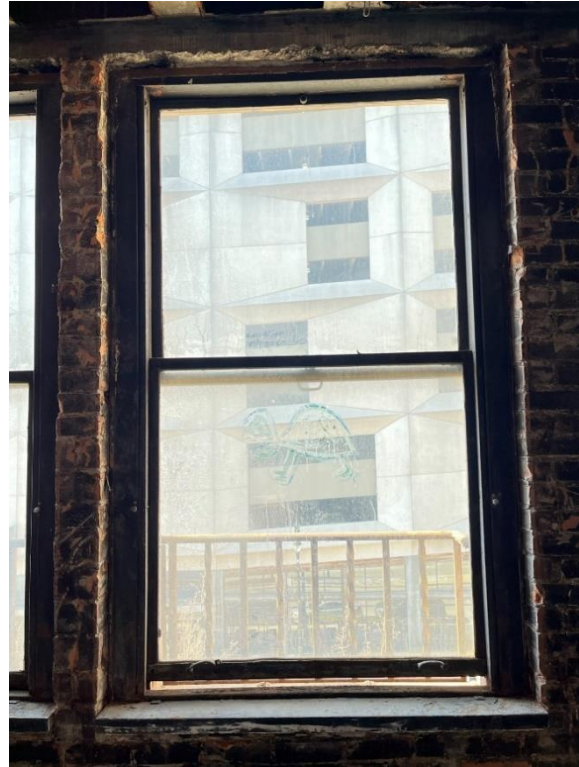
Window #29, 4 th Floor, North elevation, 04/03/23.
