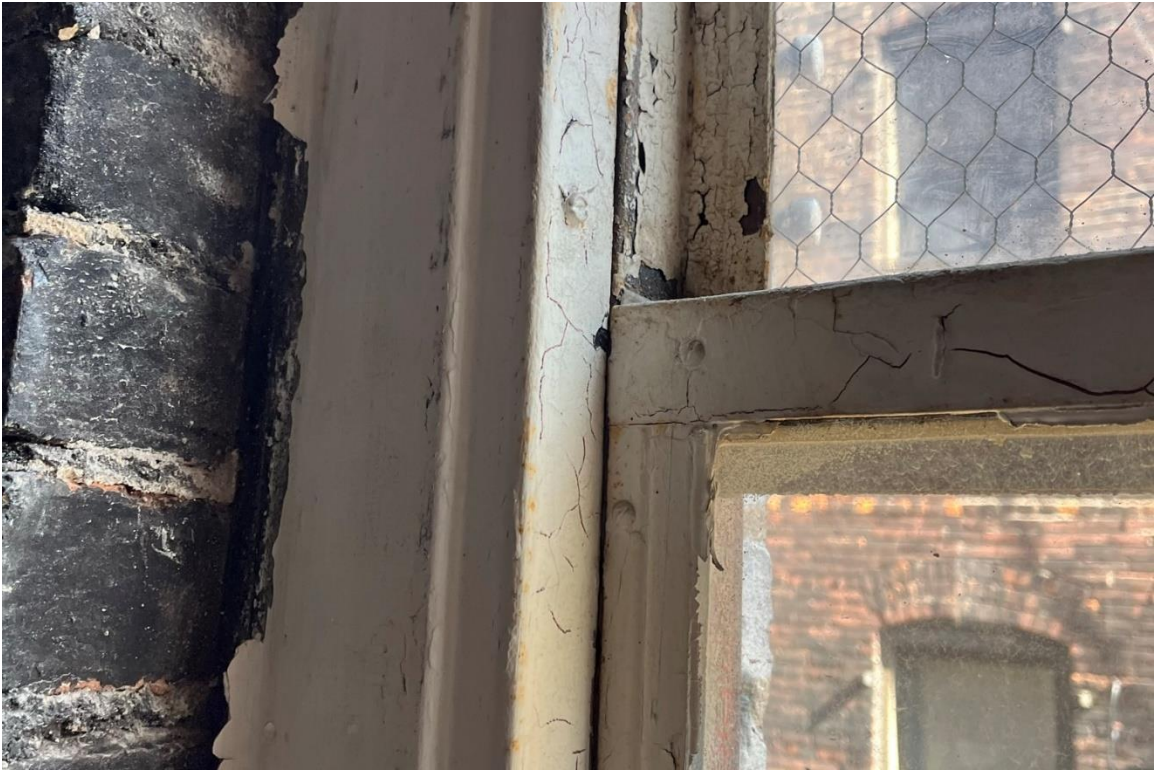
Window #33, 2 nd Floor, North elevation, 04/03/23.
