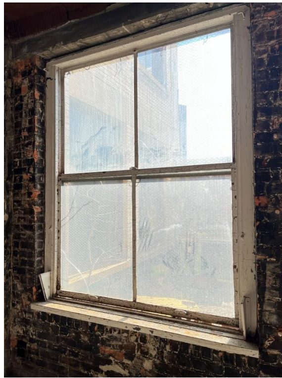
Window #30, 3 rd Floor, East elevation, 04/03/23.
