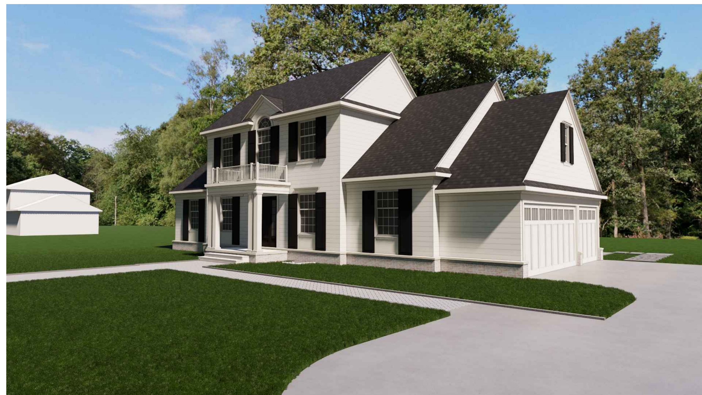
ANGLED FRONT (NORTHEAST) VIEW
