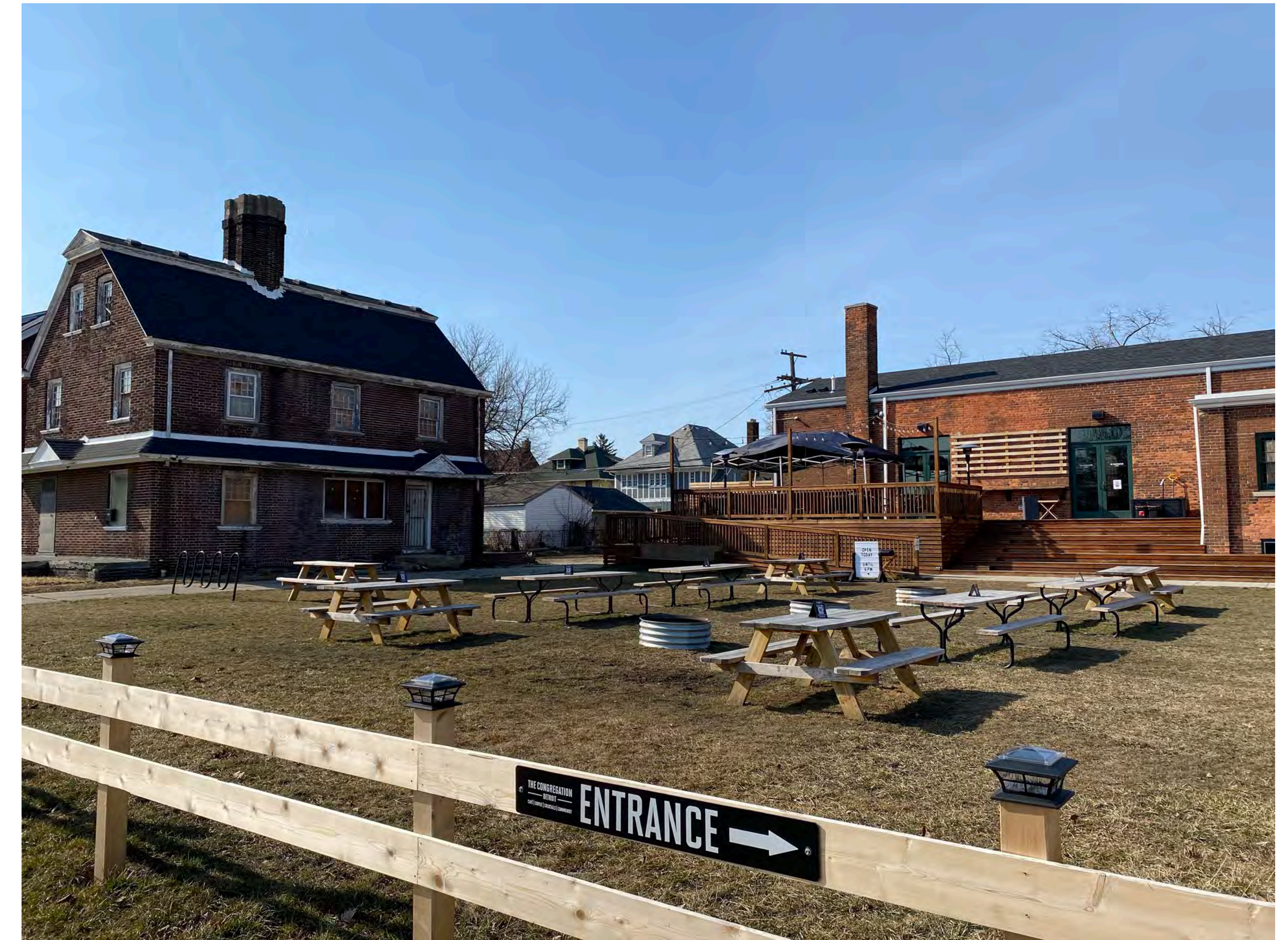
B - FRONT CORNER OF THE SITE
