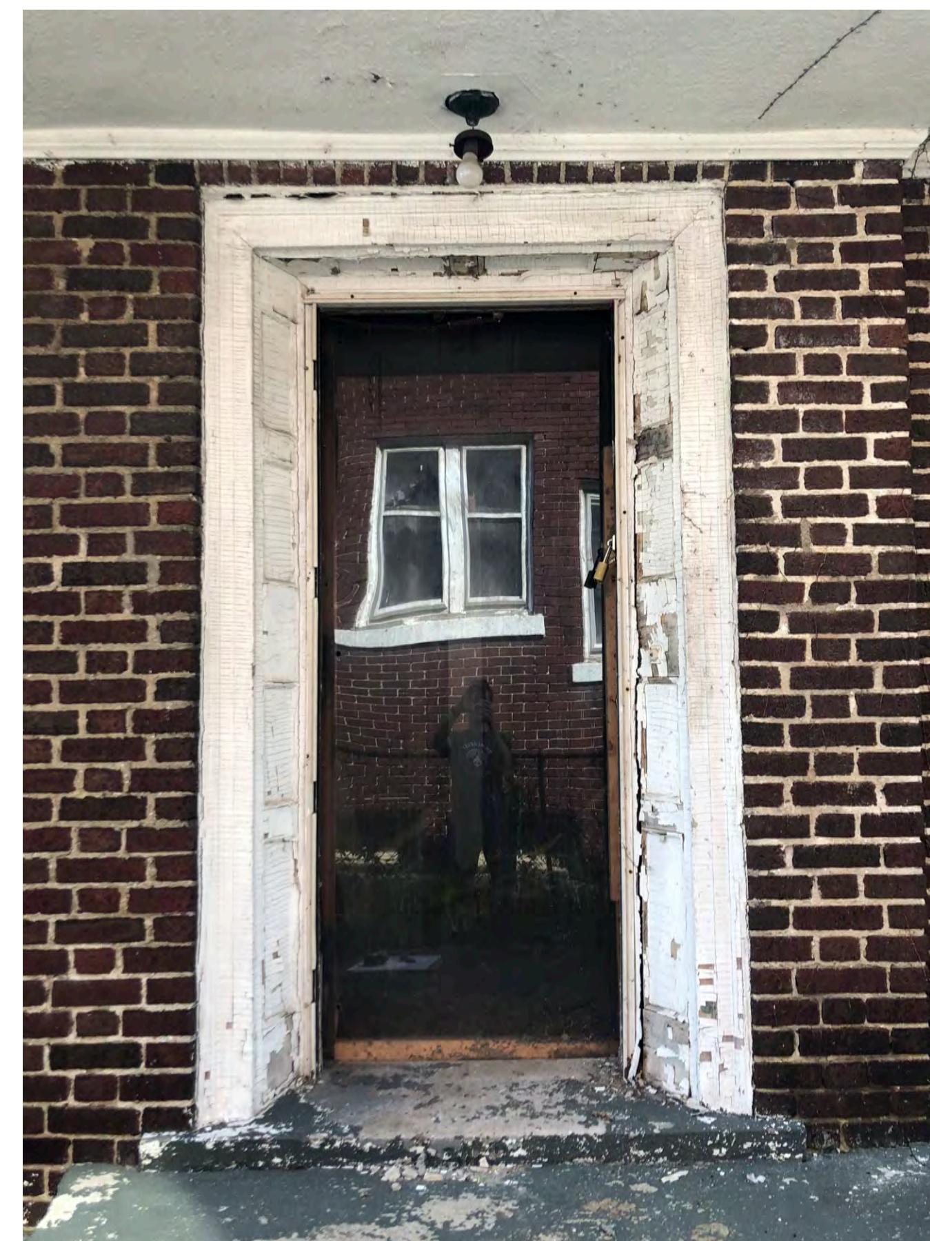
DOOR B - NEW DOOR (102) FOR SECONDARY ENTRANCE TO RESTAURANT - SEE DOOR SCHEDULE FOR DETAILS
