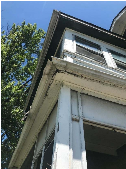
Fig 23: Typical condition of gutters
