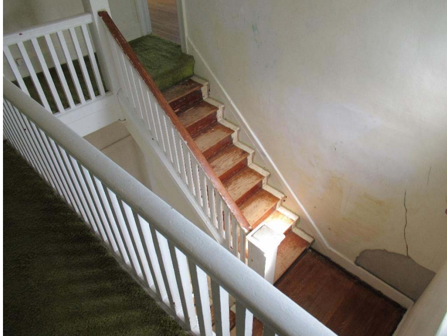
Fig 34: Second floor corridor carpeting and pine wood stairway
