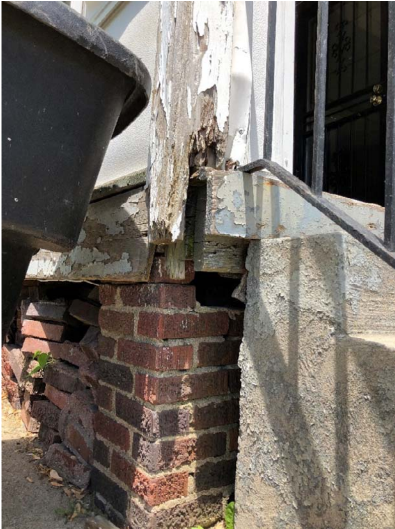
Figure 5 Brick Pier at Corner of Back Porch
