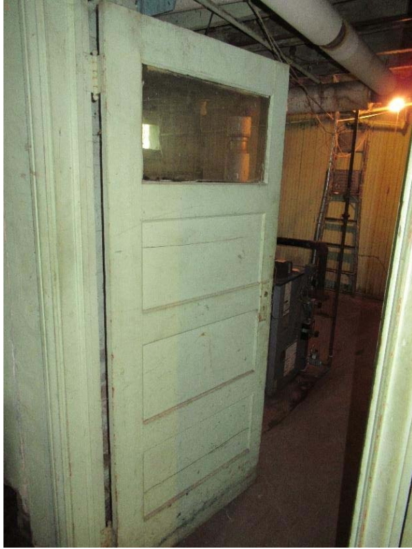
Fig 46: Basement door to boiler room
