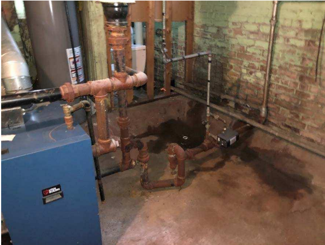
Figure 3 Shallow pit in basement slab and view of perimeter foundation wall
