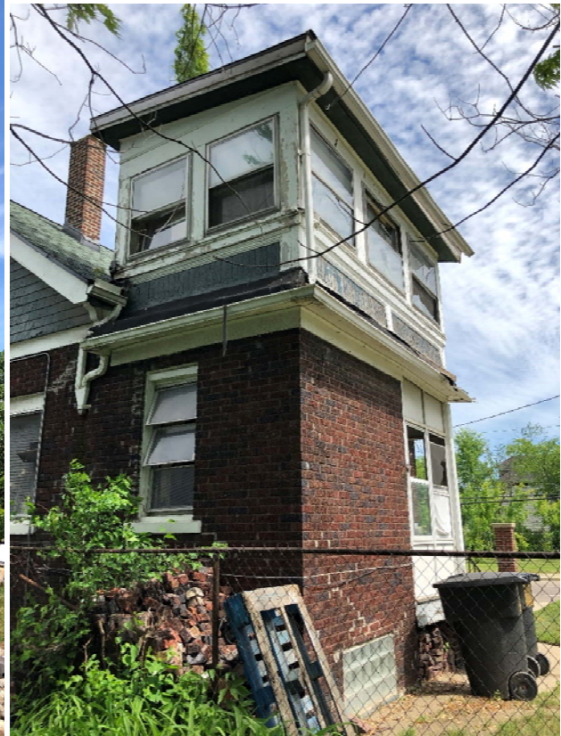
Figure 2 Northwestern Back Porch
