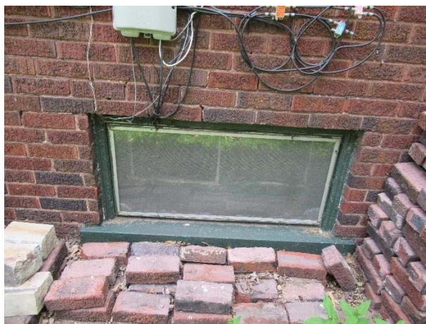
Fig 12: Typical original basement window
