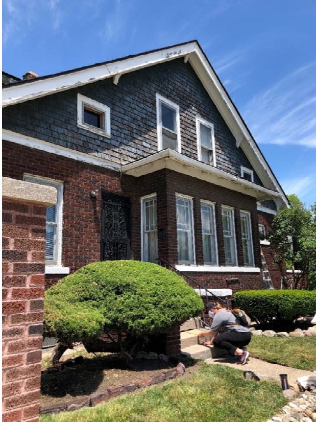
Figure 1 Eastern Dining Room Extension
