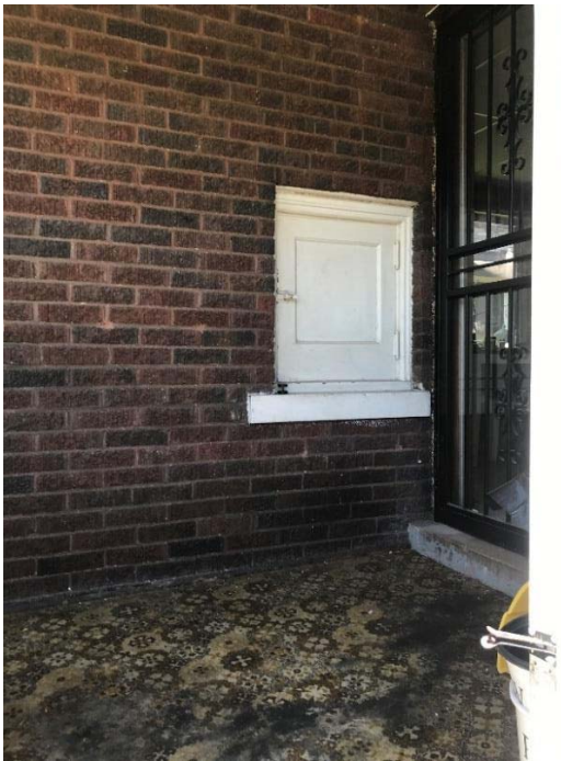
Fig 21: Interior of first floor rear enclosed porch facing northeast
