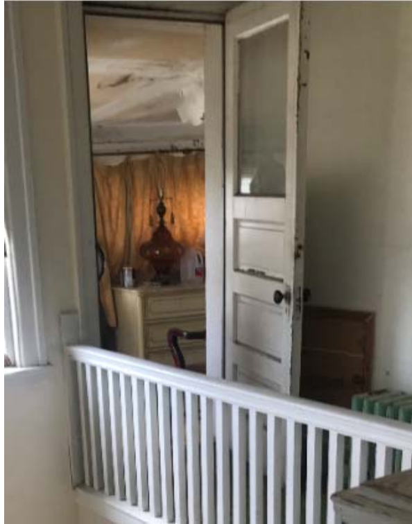
Fig 48: Door from second floor corridor to enclosed rear porch
