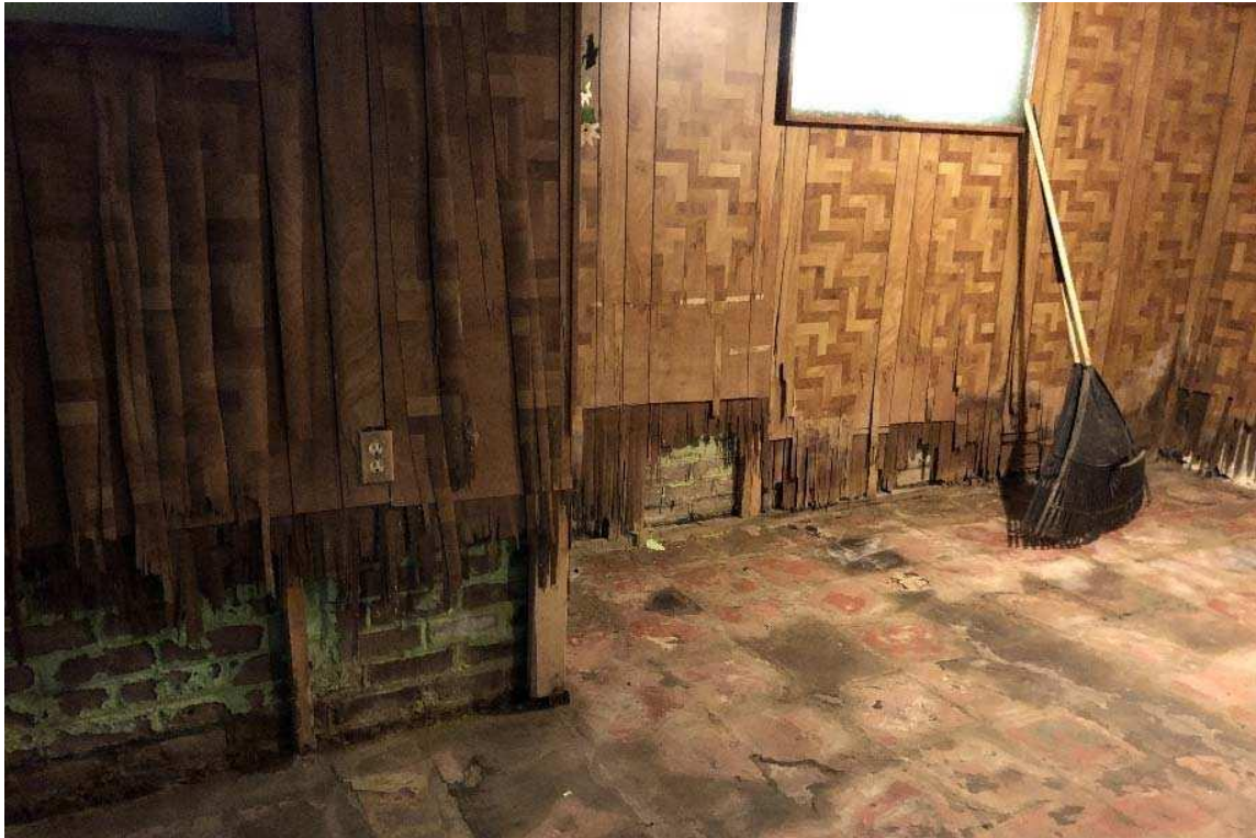
Figure 6 Basement floor and walls
