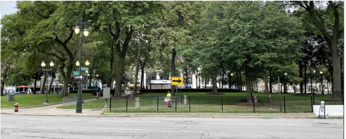
Looking north at south edge of west side, note how perimeter sidewalk ends
