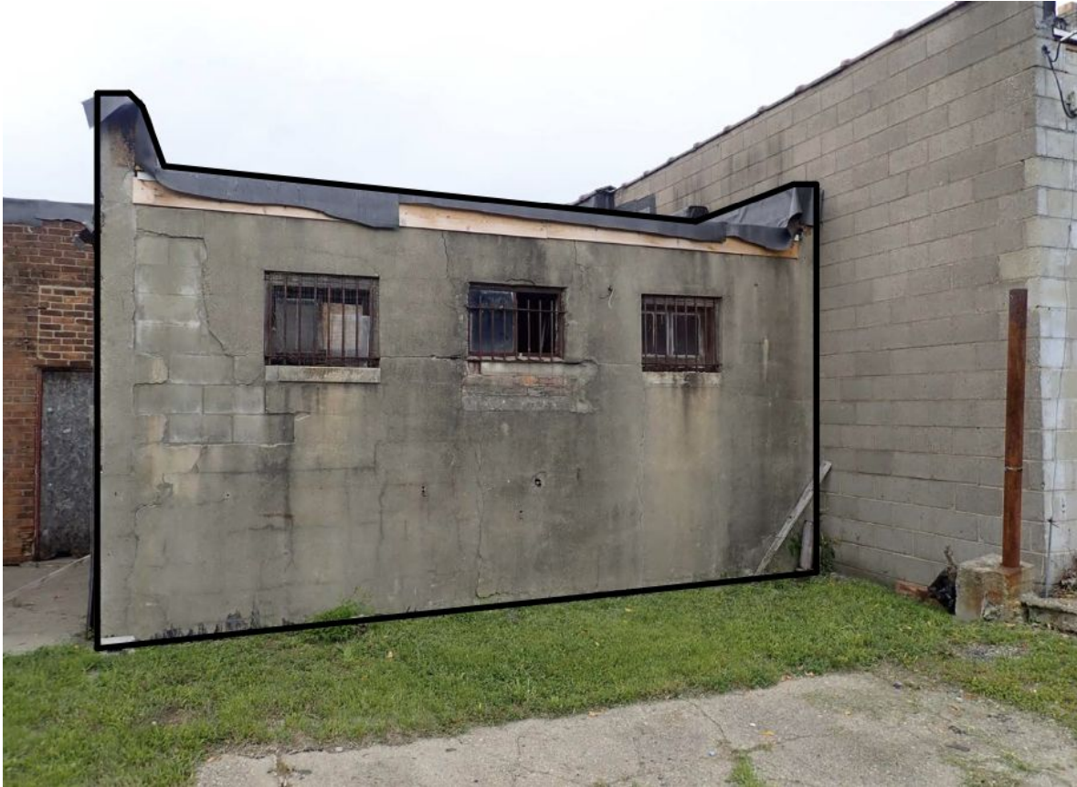
Existing Rear Addition to be Demolished
