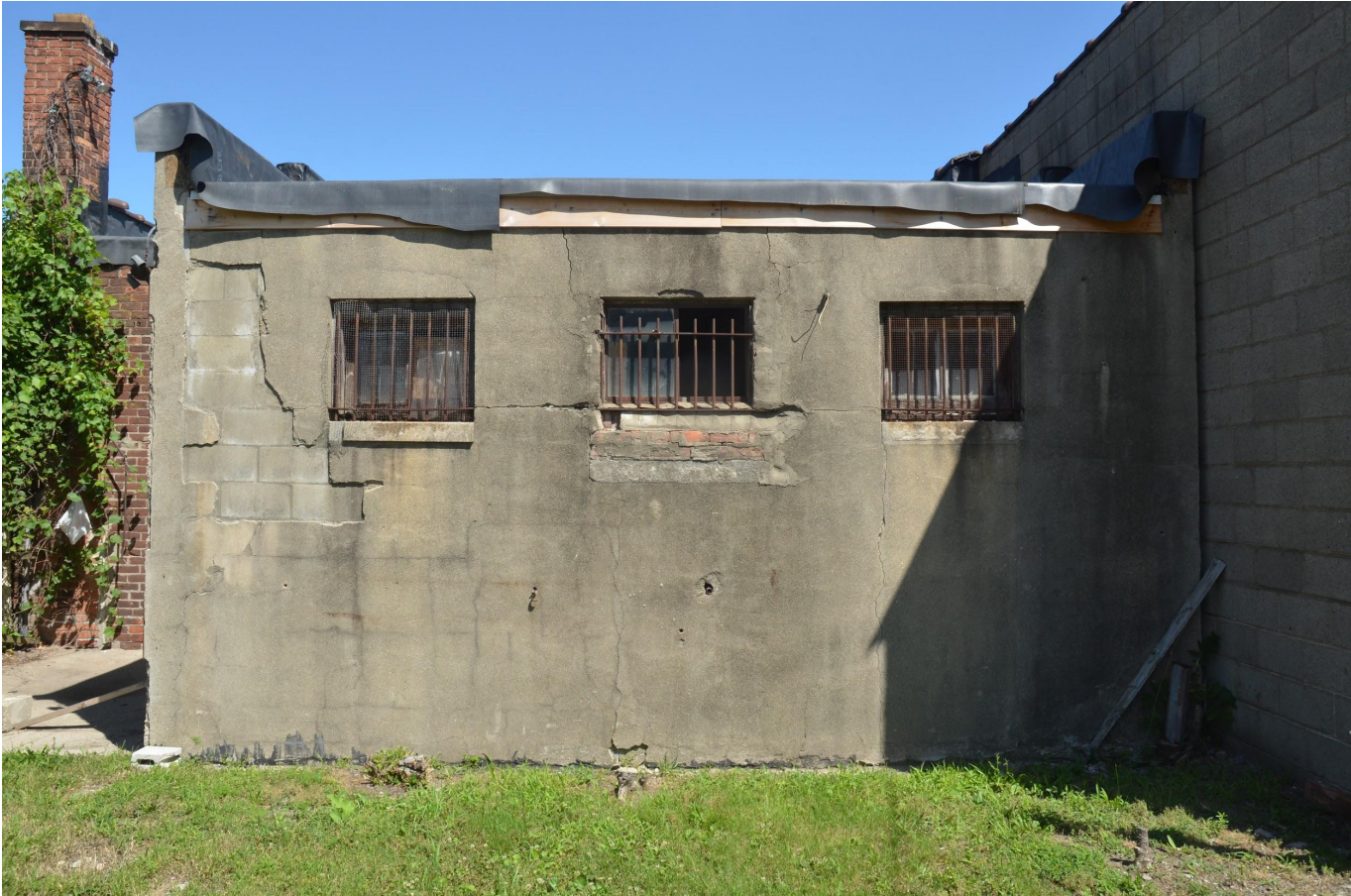
Existing Rear Addition
