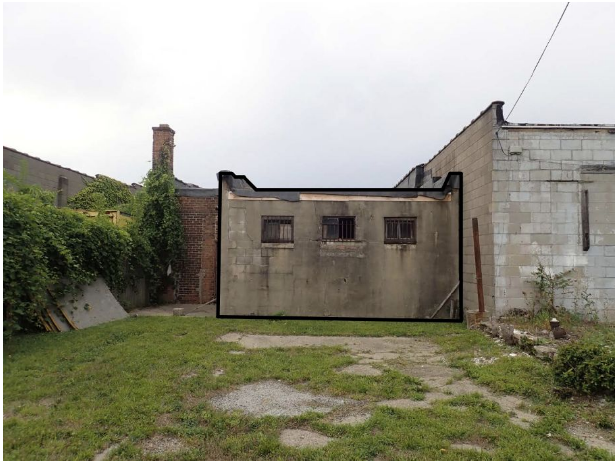
Existing Rear Addition to be Demolished
