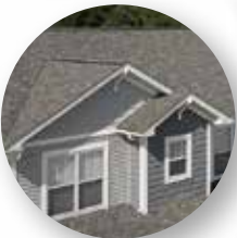
Roofing and Ventilation
