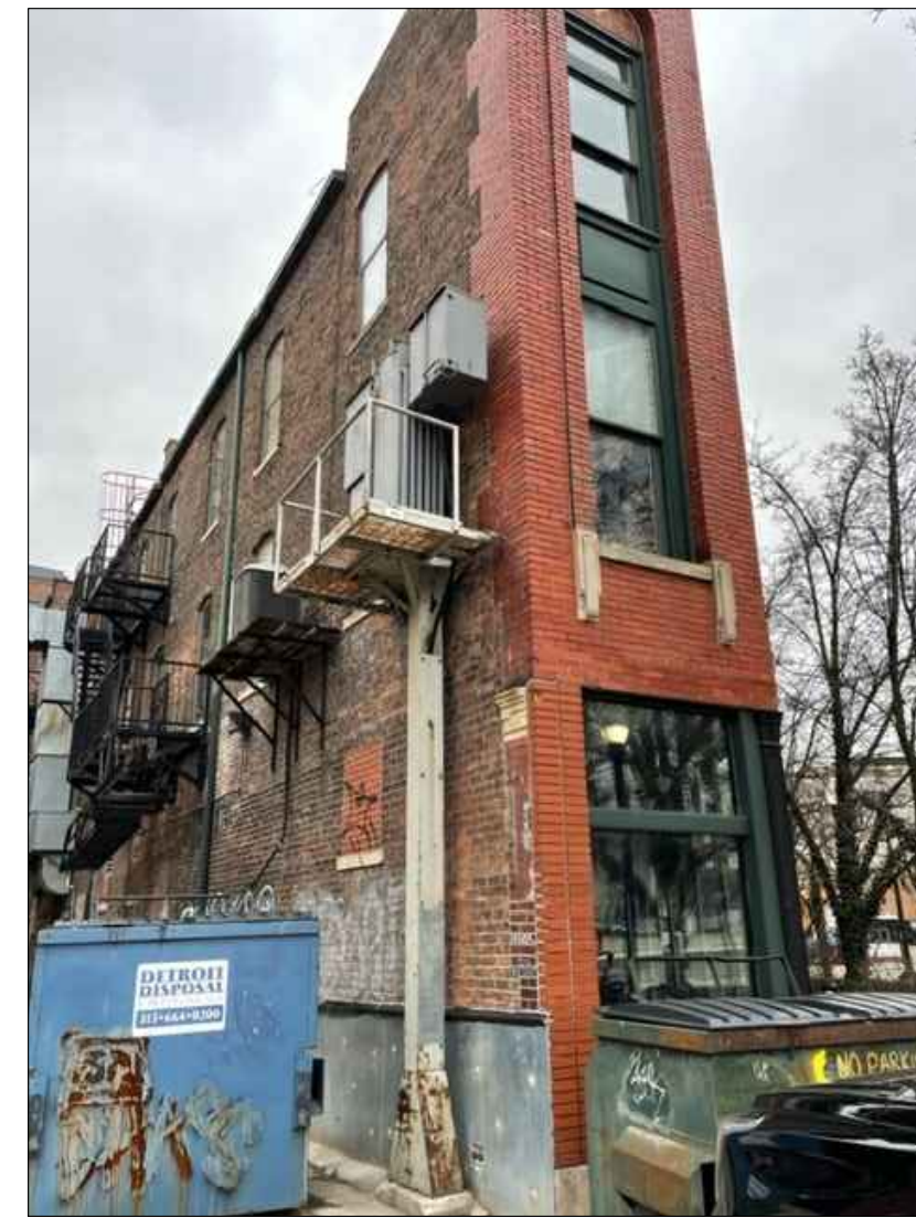
VIEW LOOKING NORTH
