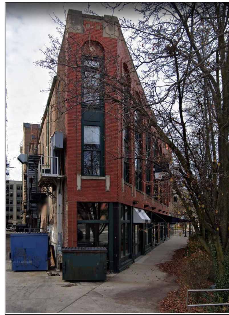
VIEW LOOKING NORTH
