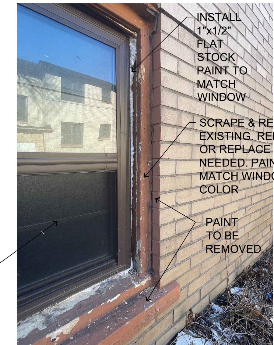
window with metal removed (bottom right view)
