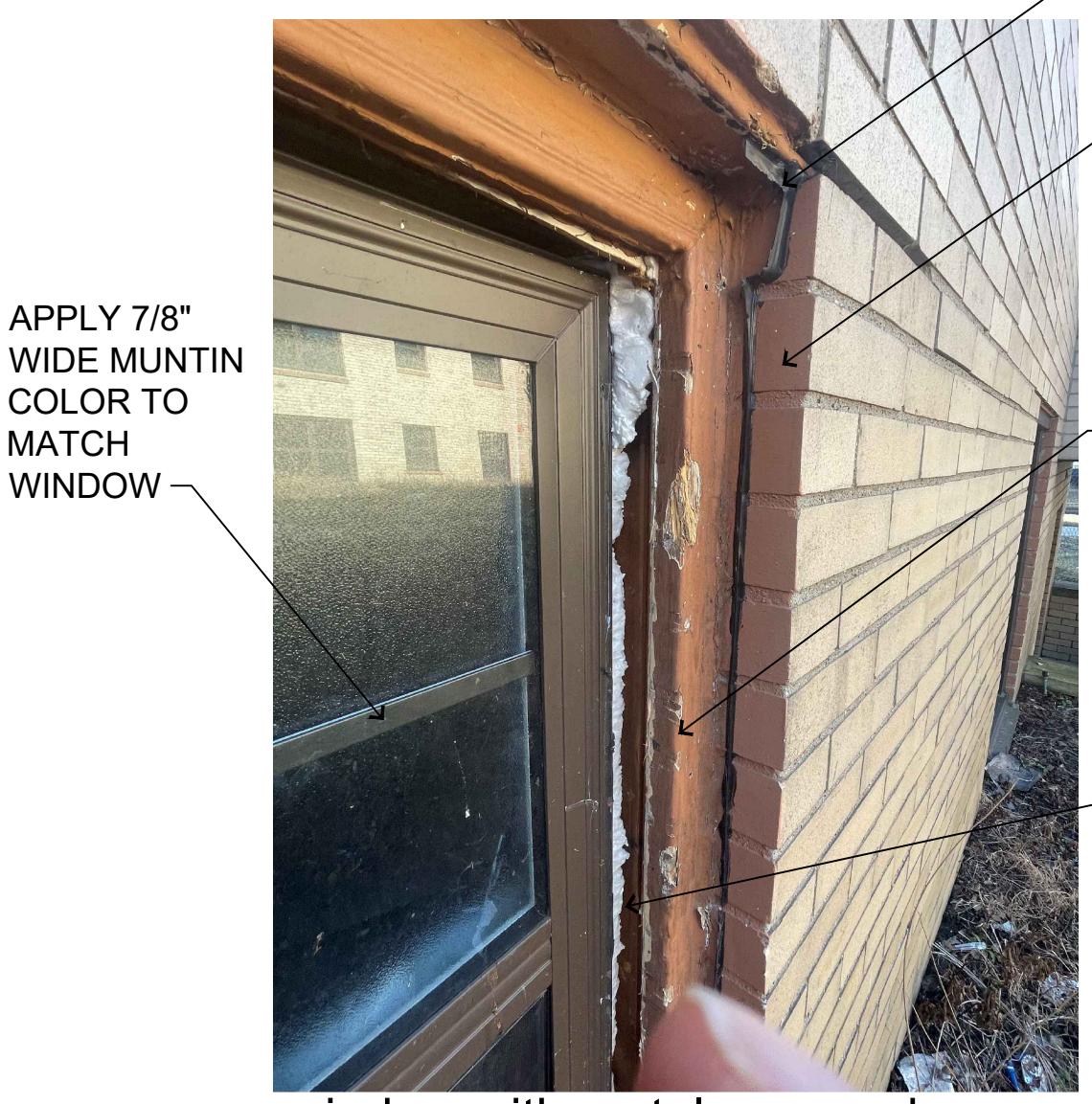
window with metal removed (top right view)
