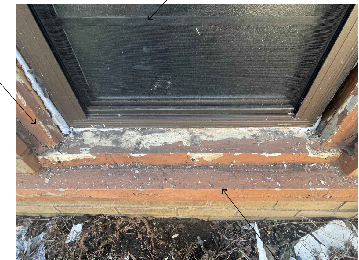
window with metal removed (bottom stool view)
