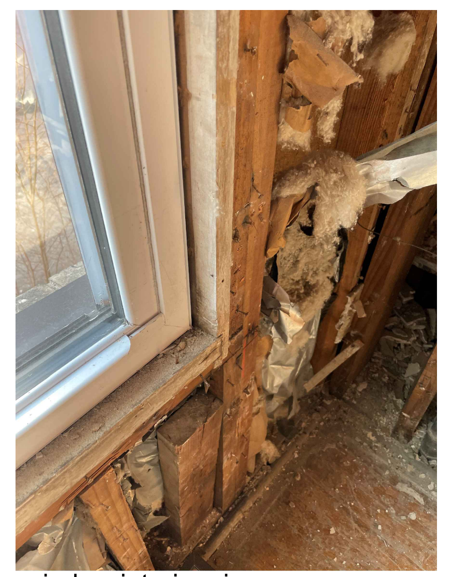
window interior view
