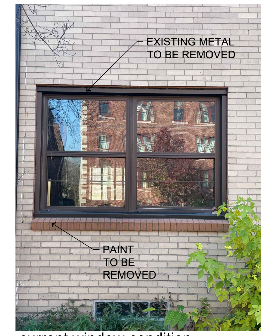
current window condition (typical for 160 windows)
