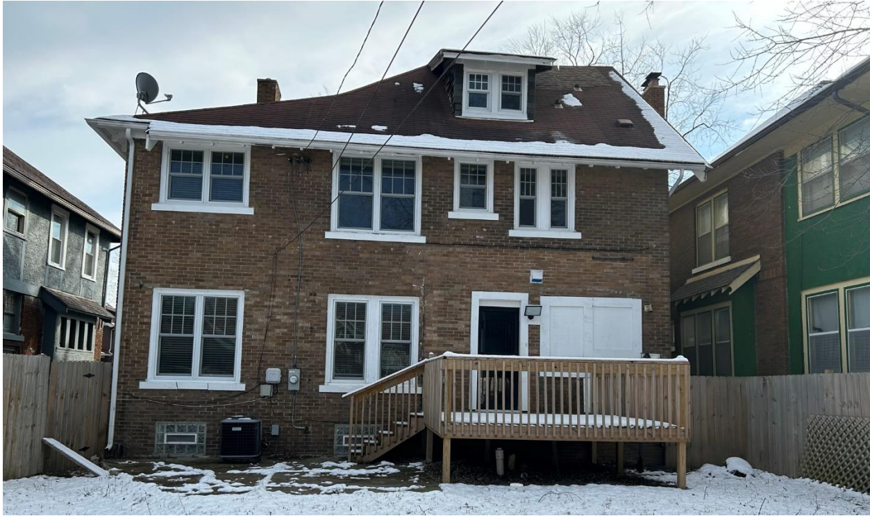
1652 Edison Street, Detroit, Michigan 48206. Rear (north) facade.
