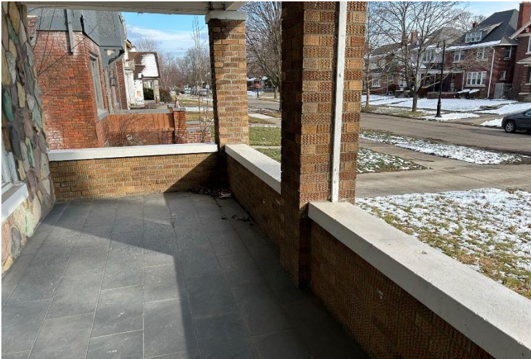
1652 Edison Street, Detroit, Michigan 48206. Front porch floor.
