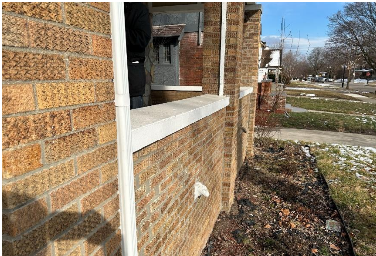
1652 Edison Street, Detroit, Michigan 48206. Front porch masonry brick.
