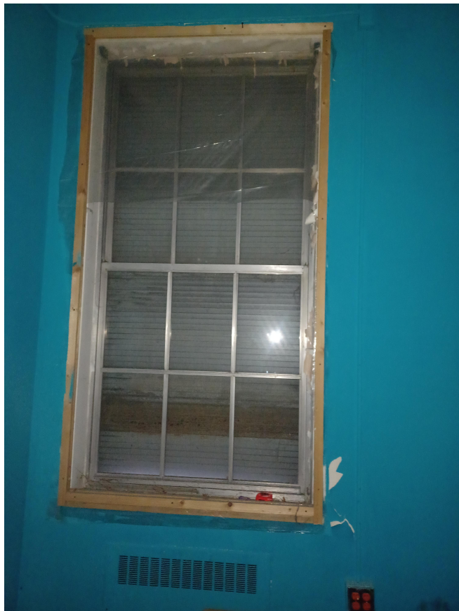
INTERIOR VIEW OF (W3) ALUMINUM WINDOW ON THE FIRST FLOOR
