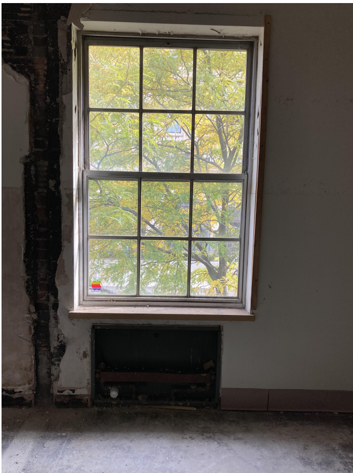
(W2) INTERIOR VIEW
