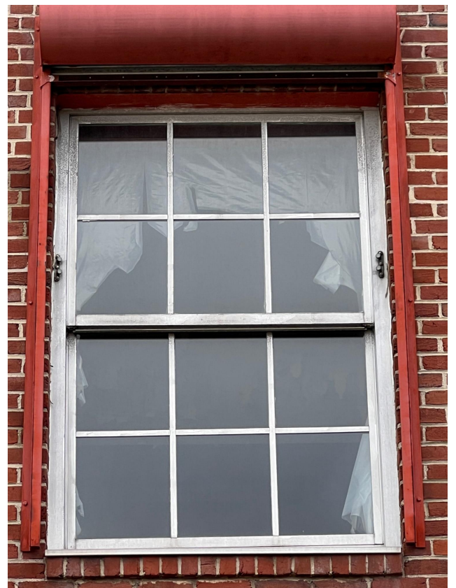
(W1) EXTERIOR VIEW EXISTING ALUMINUM WINDOW
