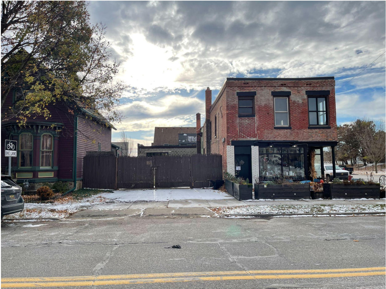
Front (North) Elevation - Bagley Avenue
